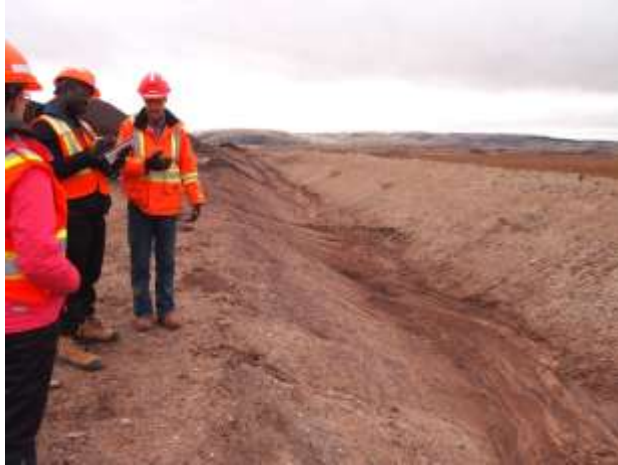
Picture 40: Ditch with no erosion protection
