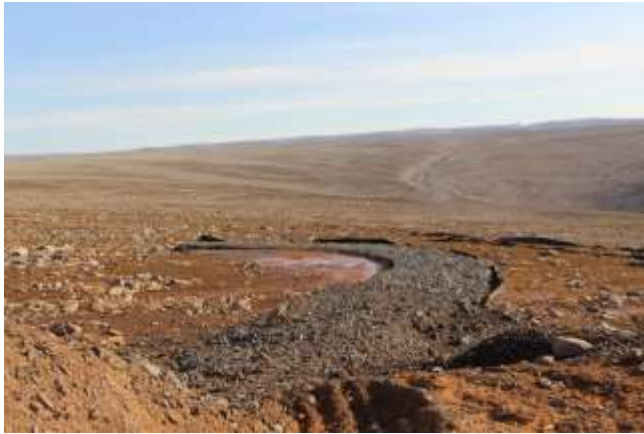
Picture 4: Check dam and silt fences beside Haul Road
