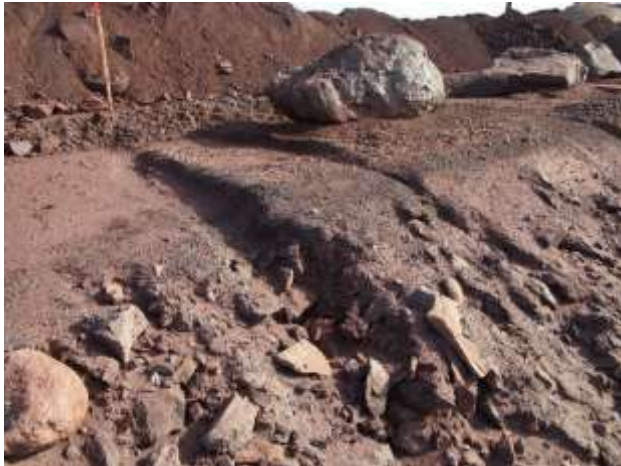
Picture 20: Erosion of Crusher Pad
