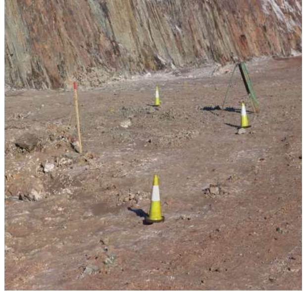
Picture 9: Cone set-up for blasting operation
