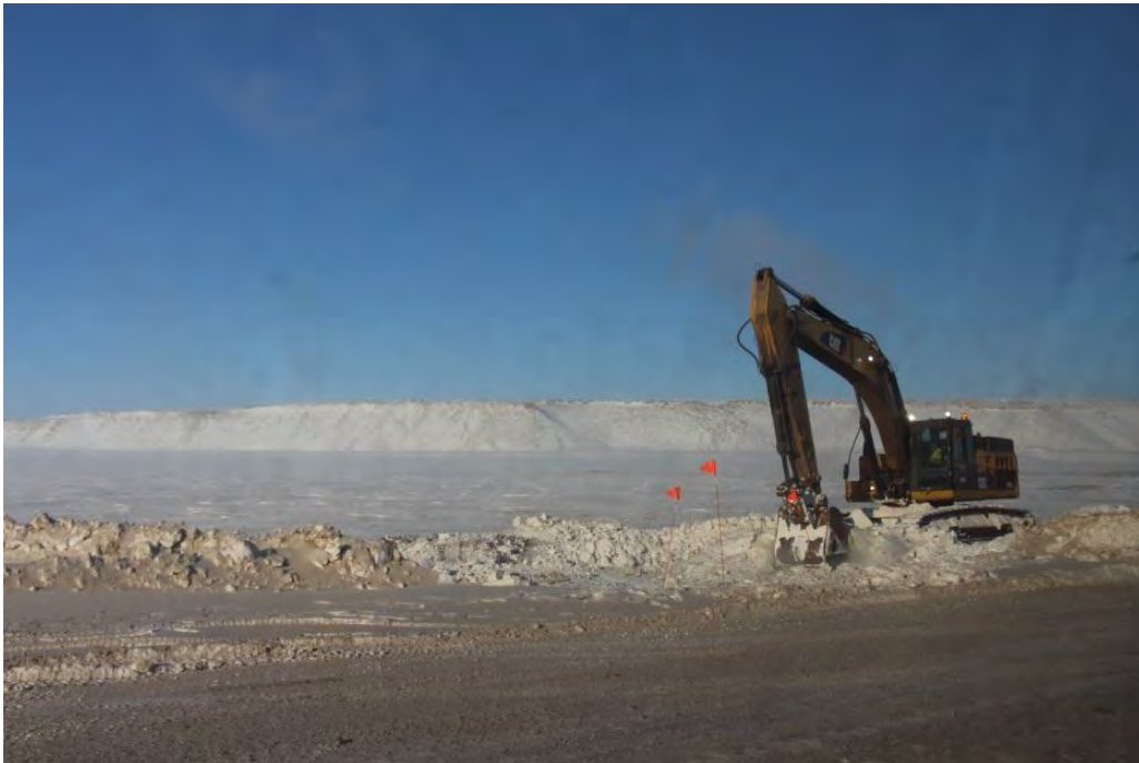
Photo 21: Excavator opening culverts preparing for freshet
