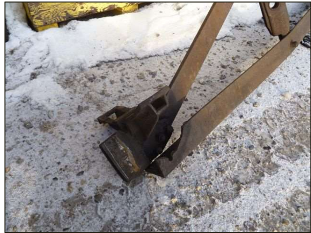
Figure Z: Worn brake beam - removed
