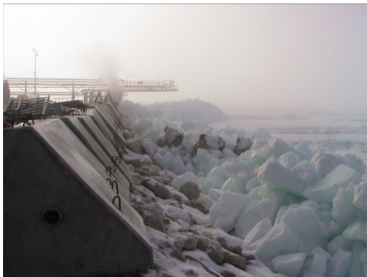
Figure 3.28: Armour stone displaced by ice (drilling island in the North Caspian Sea)
