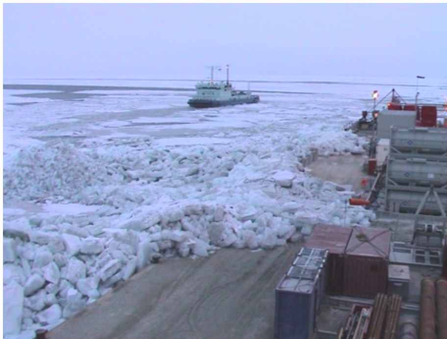
Figure 4.1 Ice over-ride incident in the Caspian Sea
