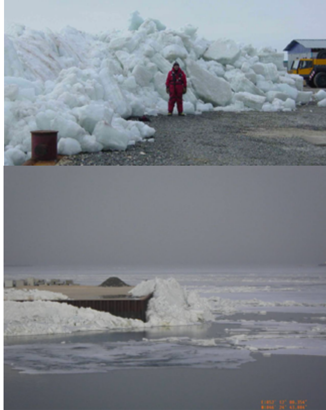
Figure 4.2: Example of pile-ups at perimeters of Caspian Sea platforms
