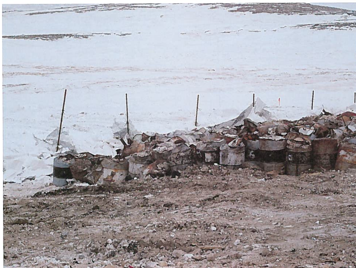
Figure 2: Blown down snow fencing and ash barrels at the inert materials landfill.
