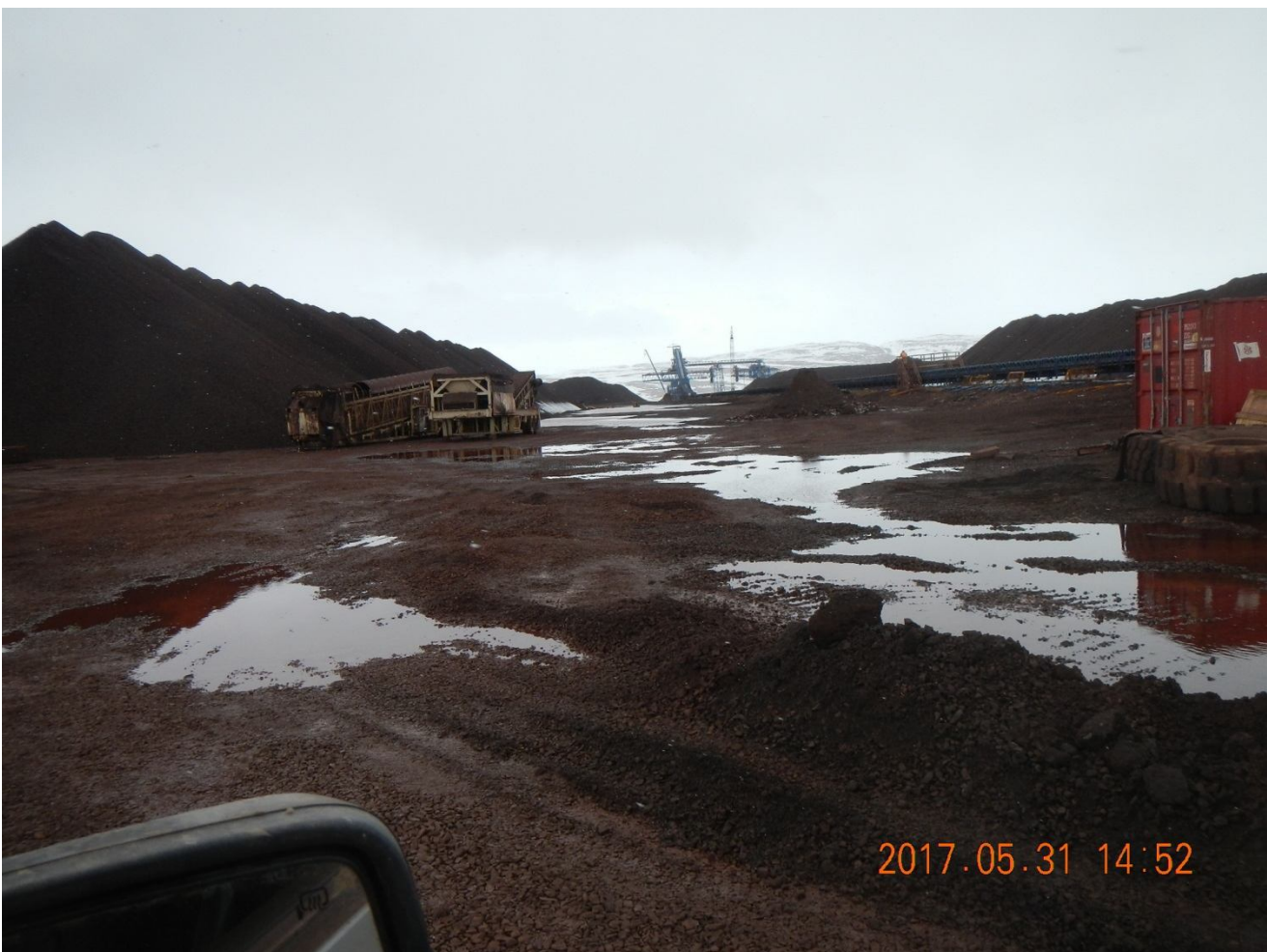
Figure 5: water pooling inside the ore stockpile pad
