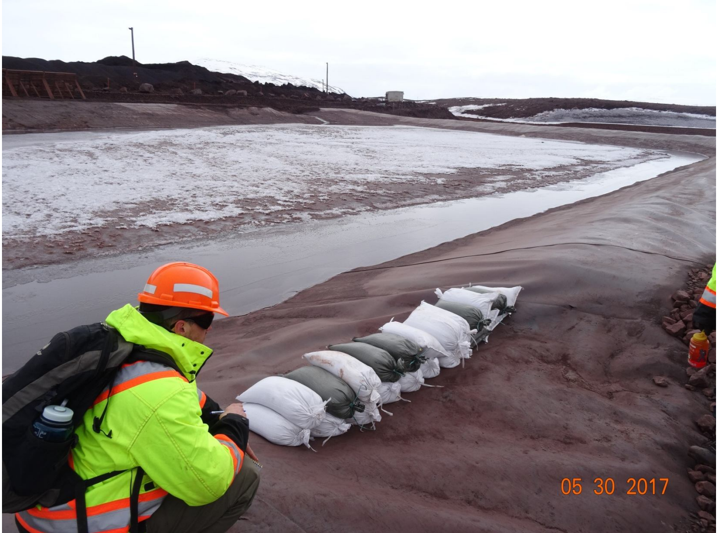
Figure 6: sandbags improperly installed
