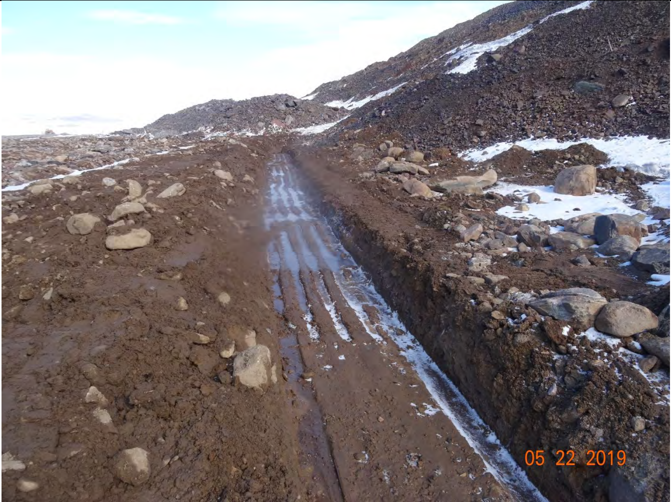
Description: Waste Rock Stockpile improperly constructed Ditches
