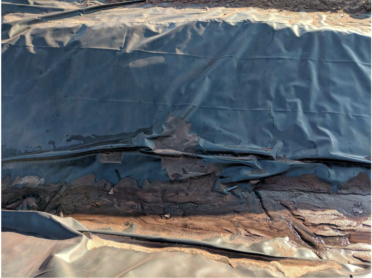
Photo 5: MP-05 Ditch Liner Repairs
