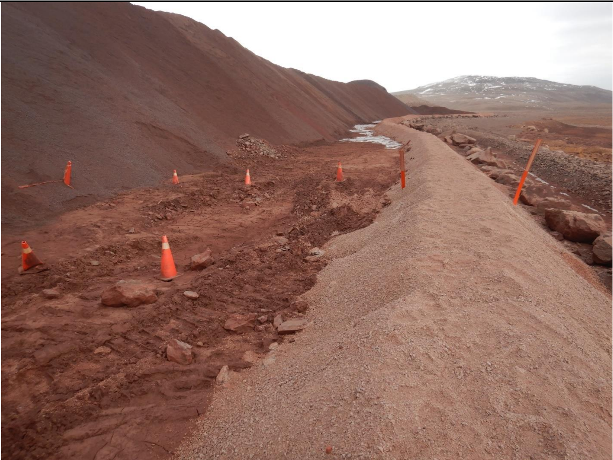
Description: Berm and sump installed.
