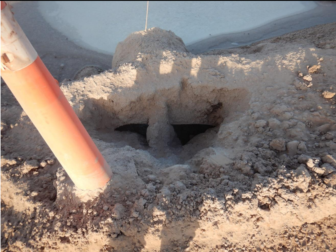
Description: Cv-001 damaged culvert.
