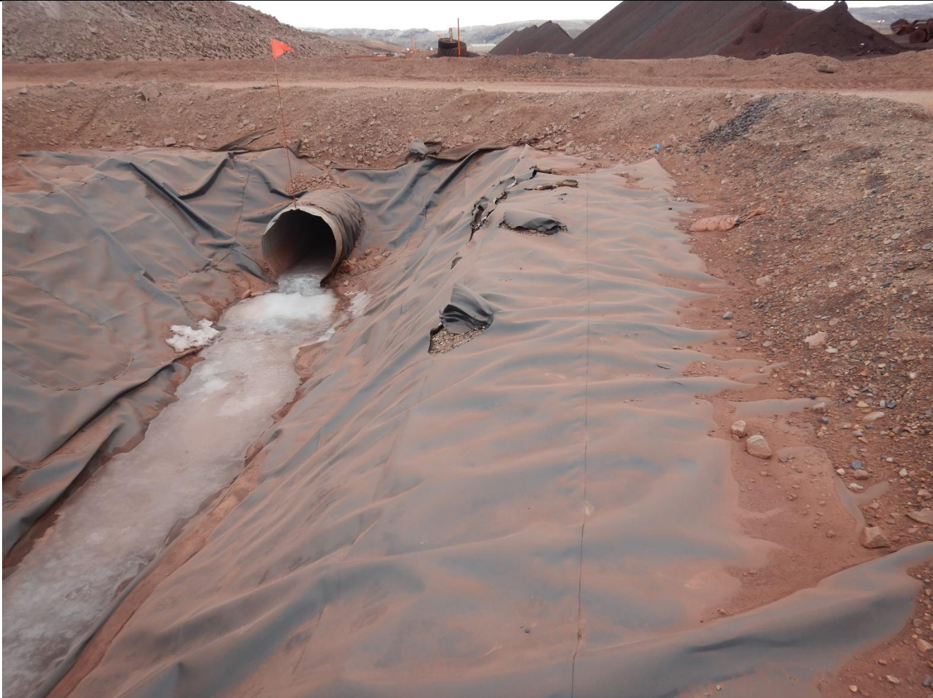
Description: damaged liner at MP-05
