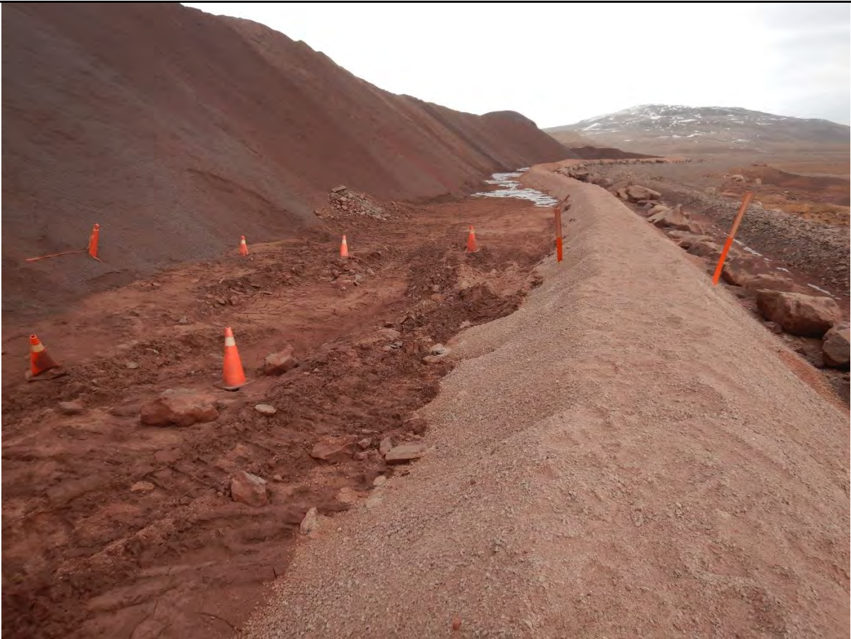
Description: Berm and sump installed.
