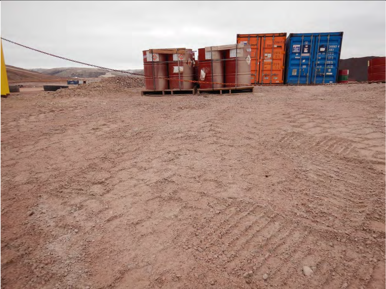
Description: standing outside the HWB’s looking in, you can clearly see there is no defined berm.
