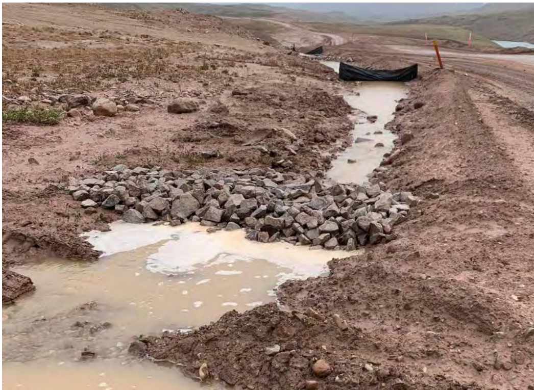
Photo 2 – Check Dams Constructed in Ditch Upstream of Culvert CV-154A – August 2021
