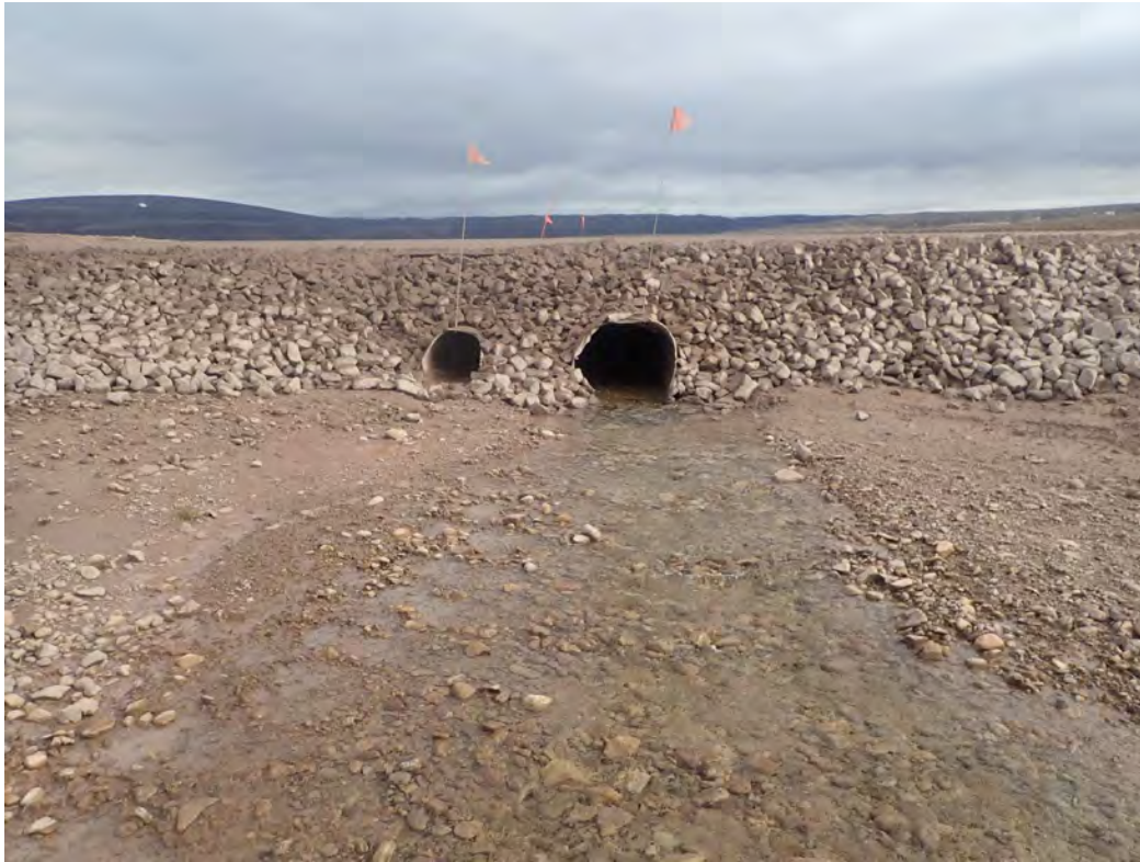
Photo 3 – Rip Rap Placed at CV-115 Outlet to Stabilize Embankment – August 2021
