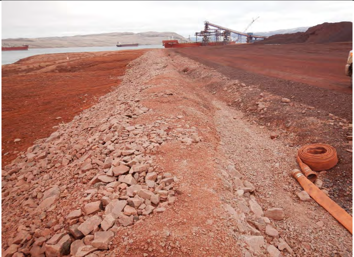
Description: hoses required for pumping and leaking area of the ditch.
