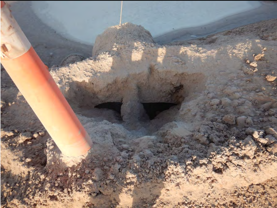
Description: Cv-001 damaged culvert.
