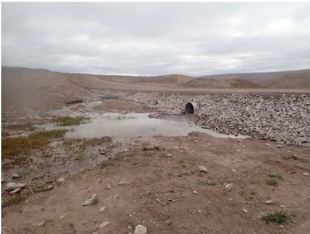
Photo 4 – Rip Rap Placed at CV-093 Inlet to Stabilize Embankment – August 2021
