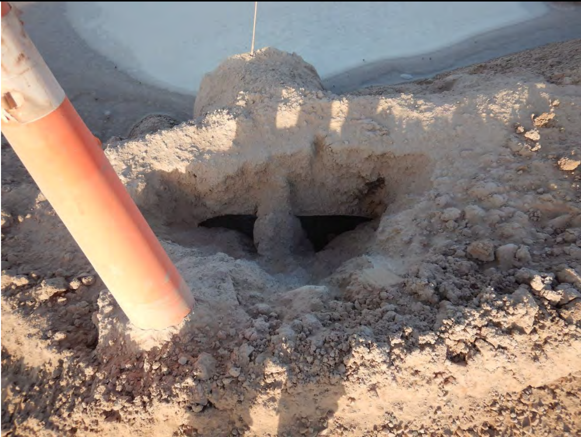
Description: Cv-001 damaged culvert.
