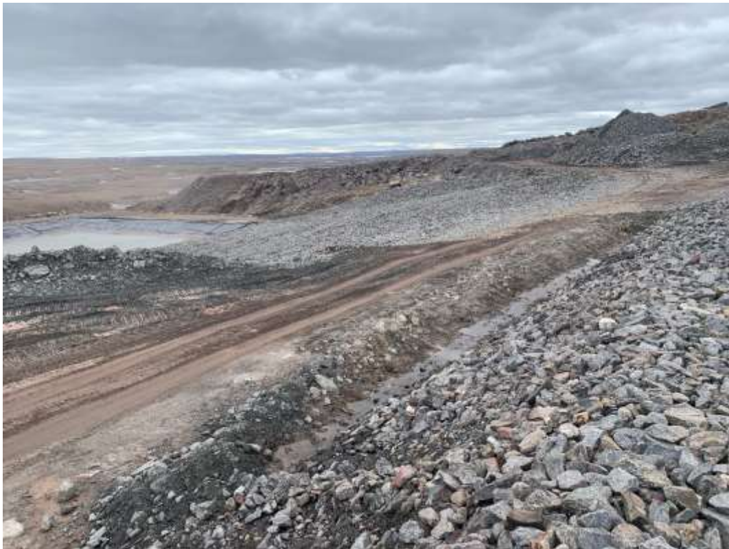
Photo 4. Temporary Diversion Swale at MS-106OS-01 spill location on July 2, 2021
