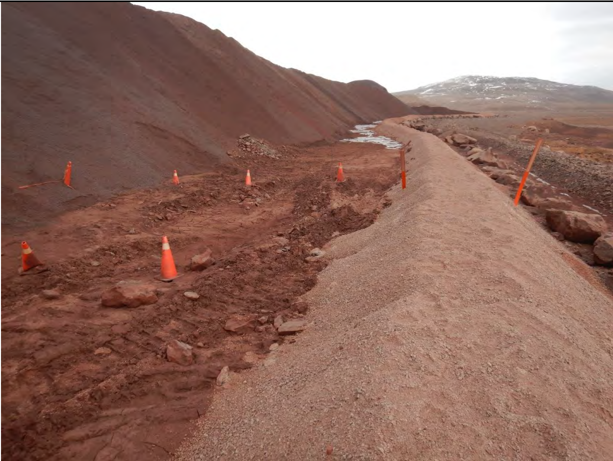
Description: Berm and sump installed.
