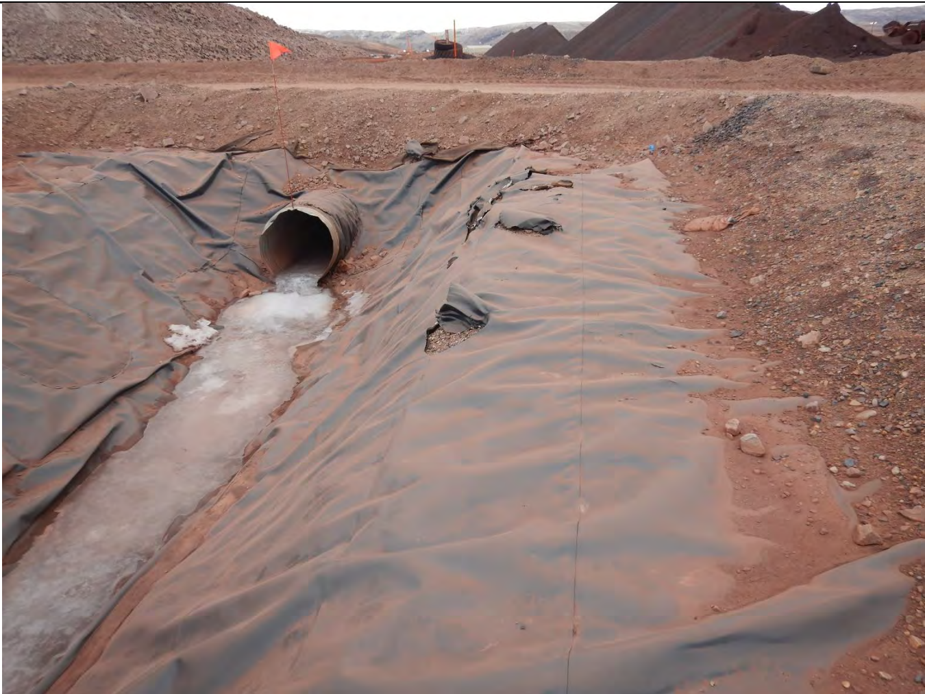
Description: damaged liner at MP-05
