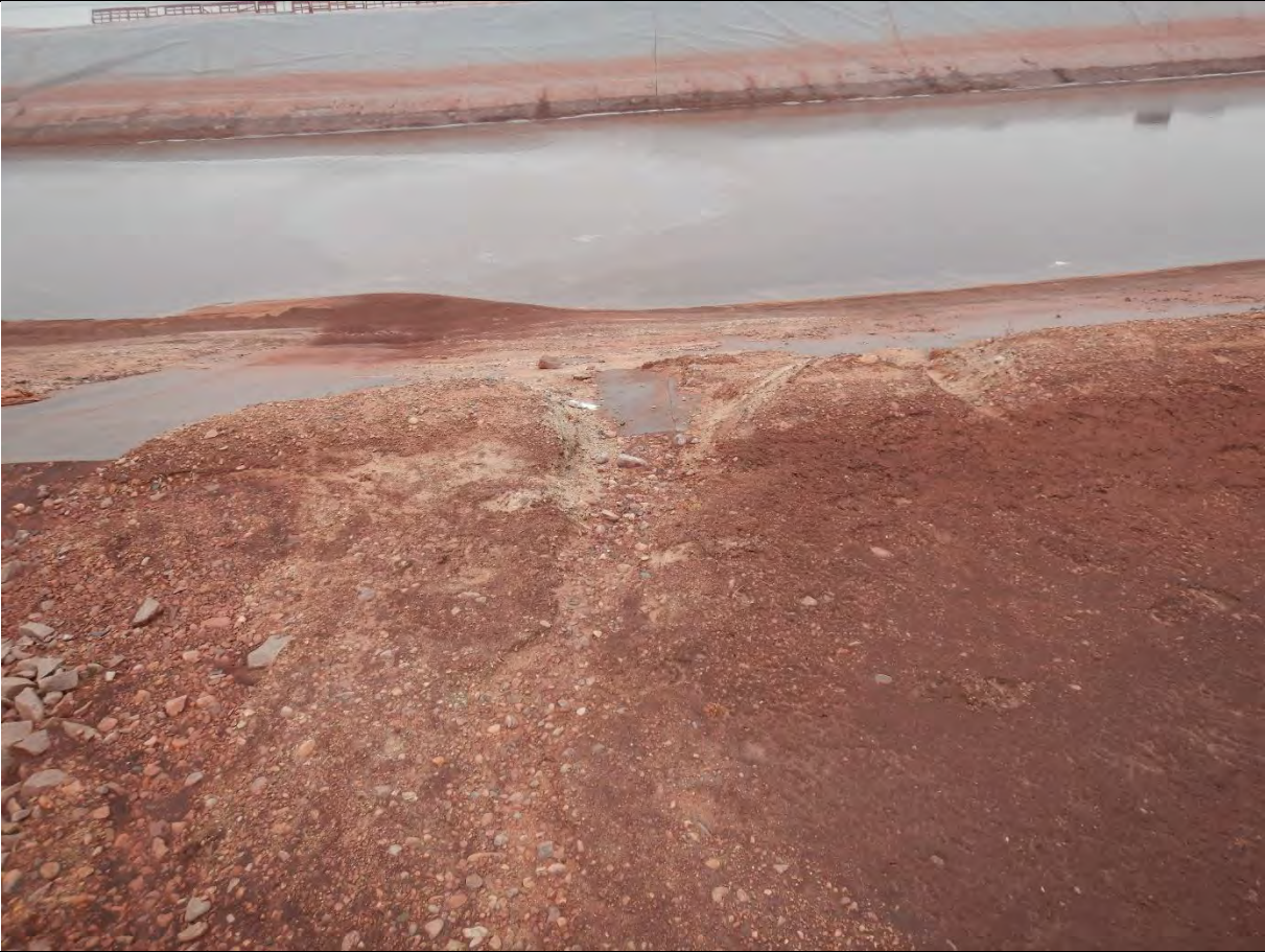
Description: erosion on the East inflow of MP-06
