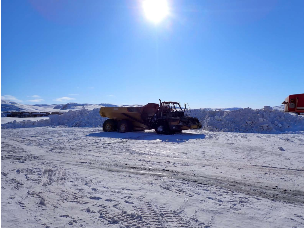
Photo 2: Articulated Haul Truck Temporarily Staged at LP3 Laydown at Milne Port – April 18, 2026
