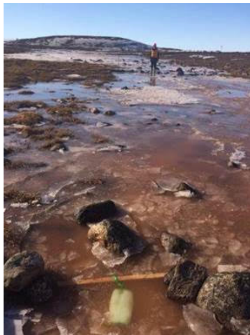
Looking upstream prior to discharge to Sheardown Lake. Flocculent blocks installed in the stream to help settle out sediment.
