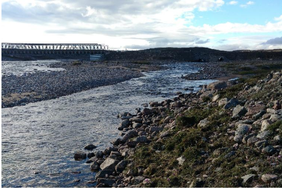
Photo 1 – Water flowing downstream of CV223 on July 31, 2016
