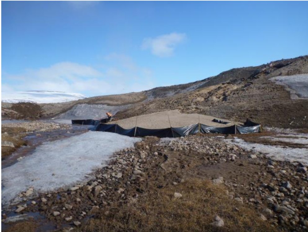
Photo 1 – May 29 th 2016. Silt fence installation around sediment deposit from slumping stream bank along Camp Lake Tributary #1.
