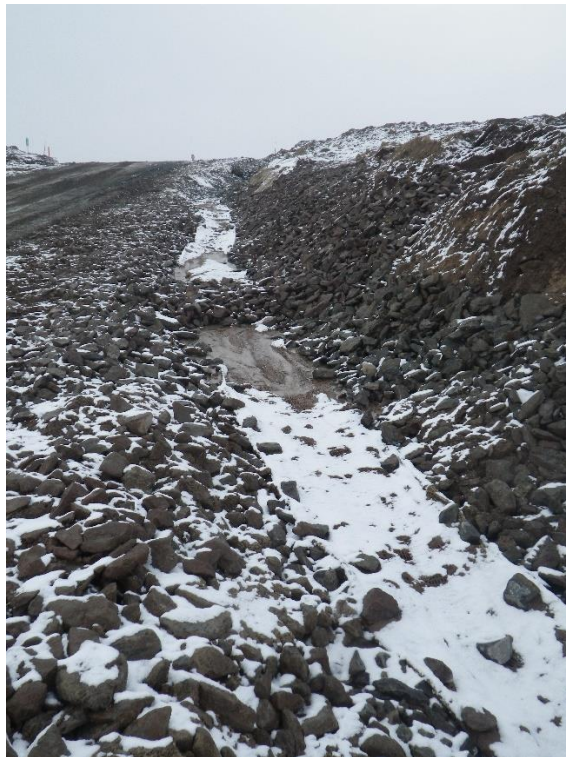
Photo 2 – Swale draining airstrip runoff lined with 6" aggregate and treated jute to capture sediments.
