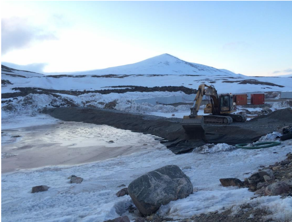
Photo 1– April 28 th 2016. Construction of Check Dam # 4 near the end of Magazine Access Road.
