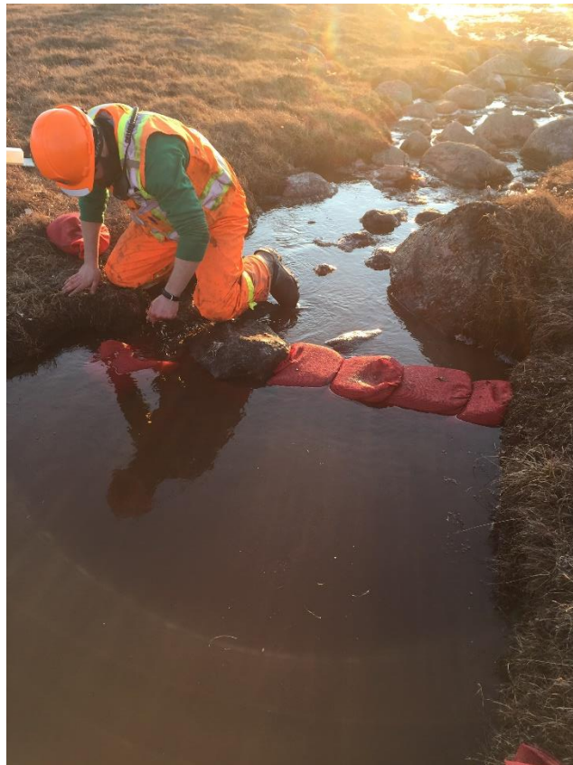
Photo 4 – Sand bag check dams installed along Sheardown Lake Tributary LDFG near landfill access road.
