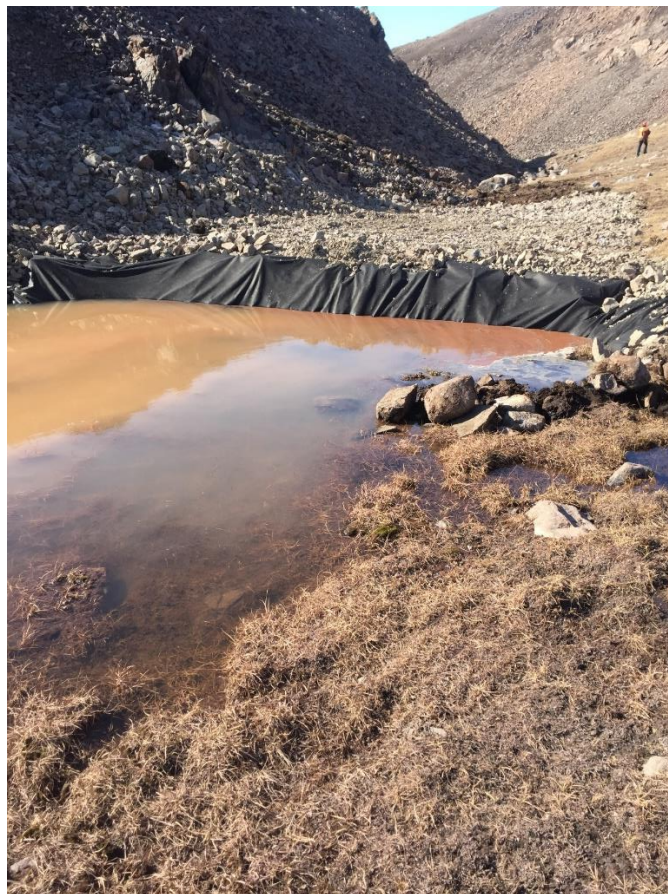
Photo 6 – Check dam constructed at outlet of Sheardown Valley along Mine Haul Road.
