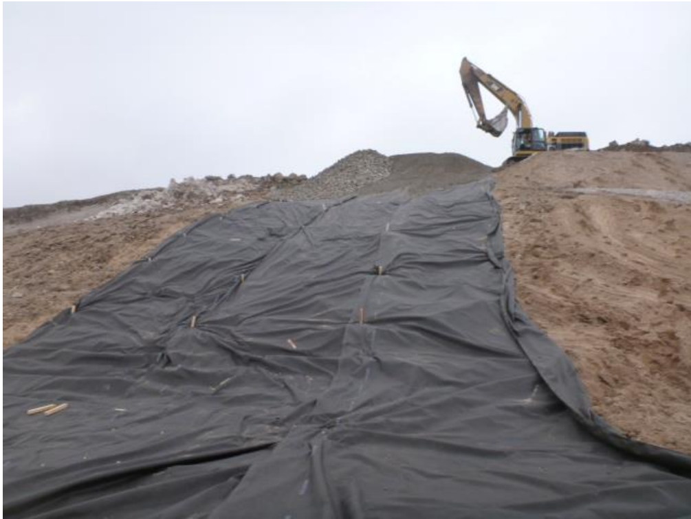
Photo 3 – June 3 rd 2016. Slumping stream bank lined with geotextile to protect underlying soil from erosion.
