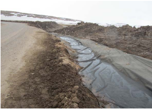
Constructed Drainage Controls Partially Implemented or Completed.
