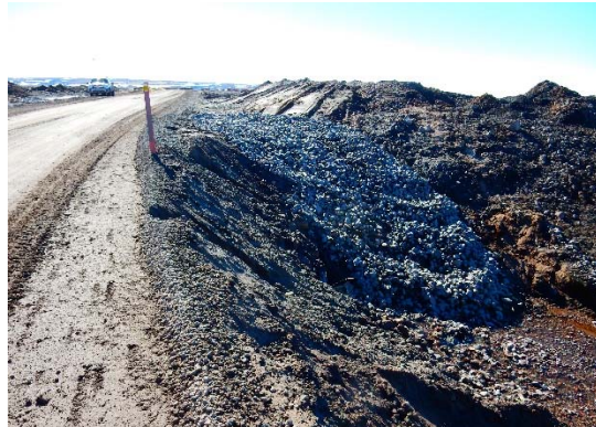
Constructed Drainage Controls Partially Implemented or Completed.
