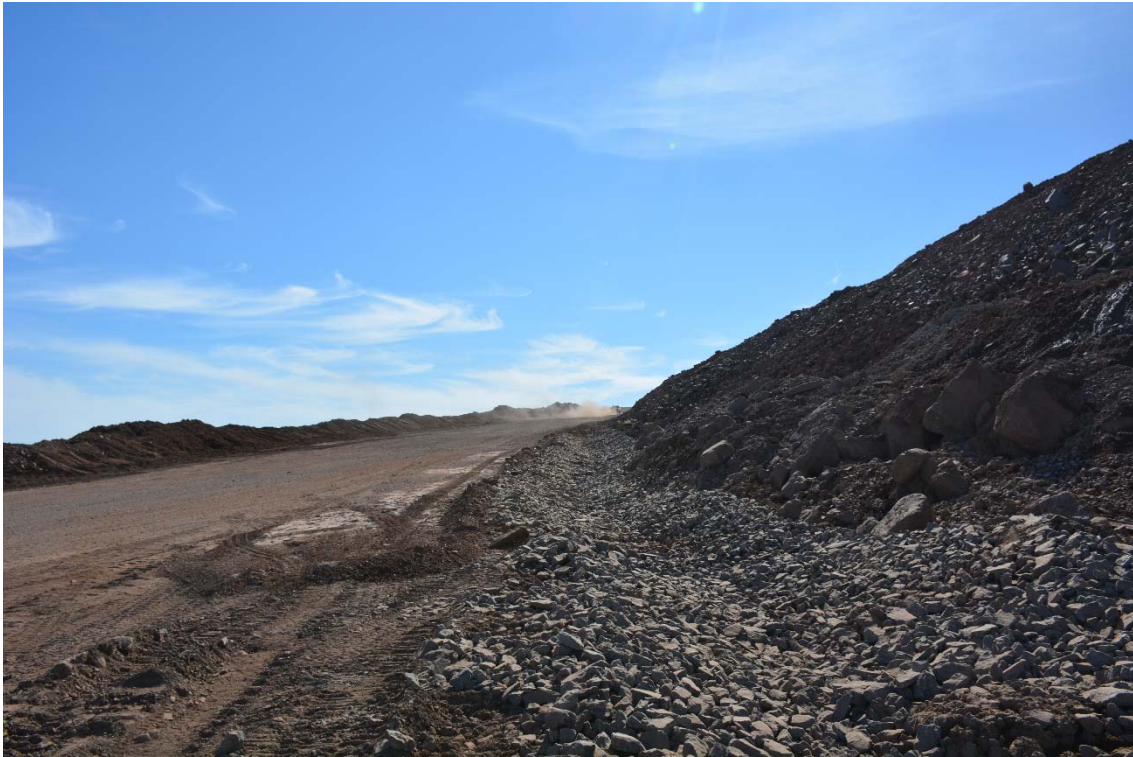
Photo 4 - New ditch with geotextile and rip rap up from Km 108.5. Picture taken on July 5, 2016
