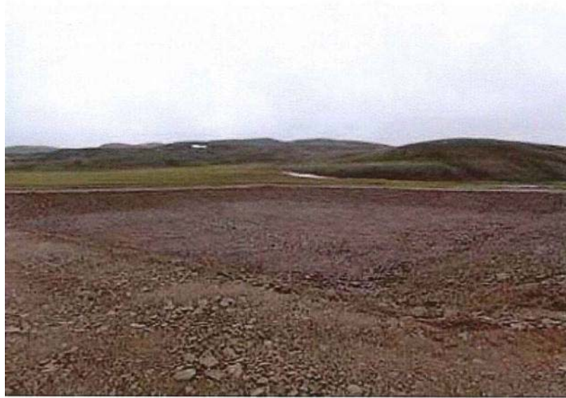
Figure 1: Before – Sub-grade Prepared
