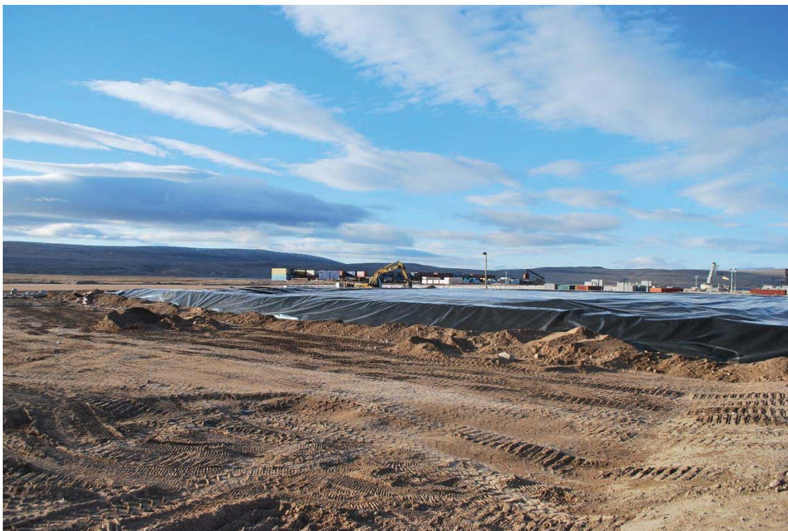
Photo 10 – Sealed Containment Berm on North End of the Facility
