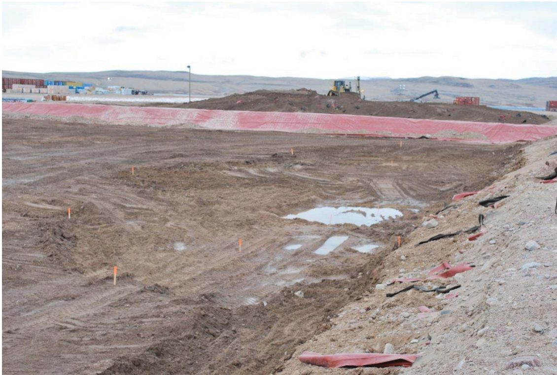
Photo 7 – Final Excavation of the Containment Berm Sump Area
