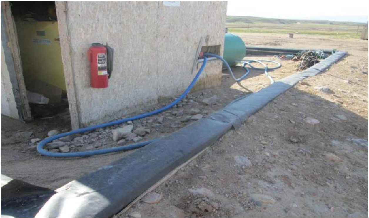
Helicopter Fuel Tank Containment.
