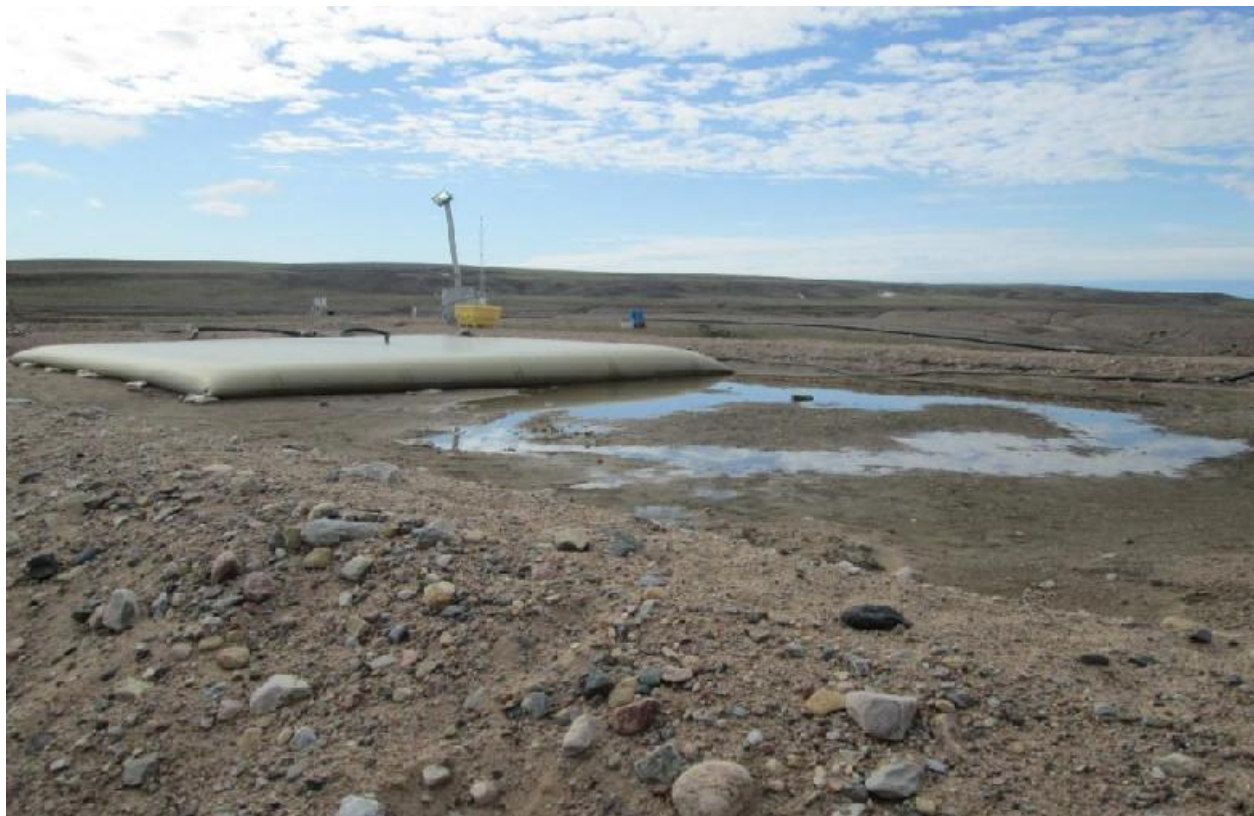
Generator Fuel Storage Facility Containment
