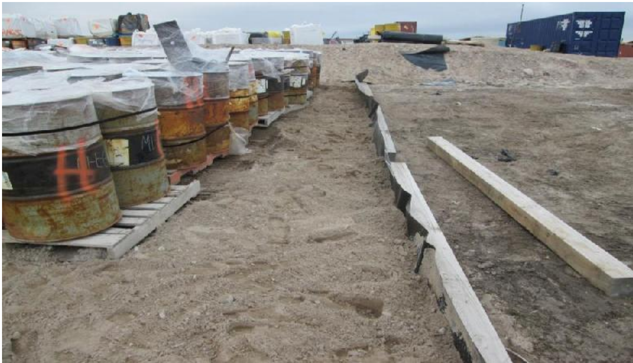
Photo shows temporary curbed area for hazardous waste awaiting immediate shipment.
