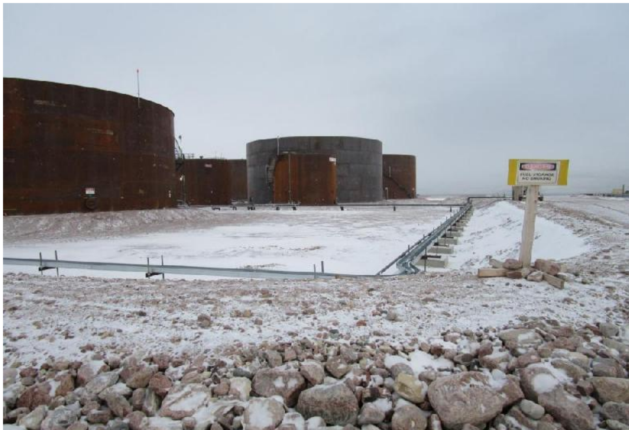
Fuel tank farm containment
