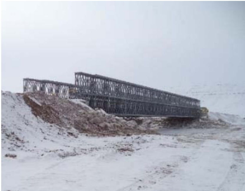
PHOTO 3 Completed bridge at km 17
