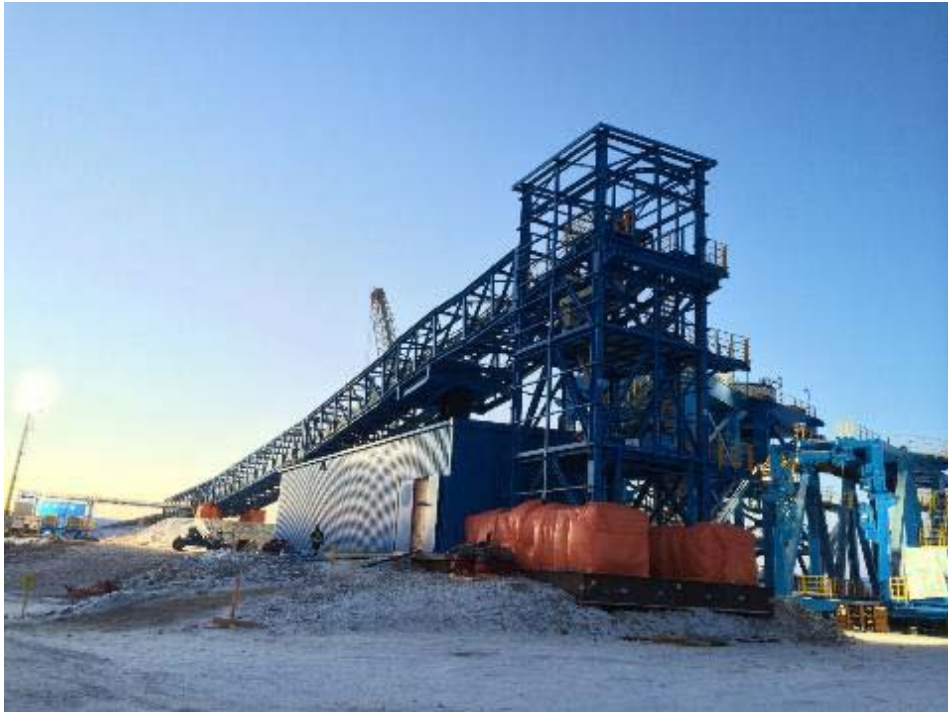
PHOTO 17 Conveyor Construction Early November 2014
