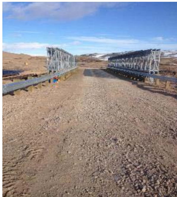
PHOTO 4 Completed bridge at km 17 during Freshet
