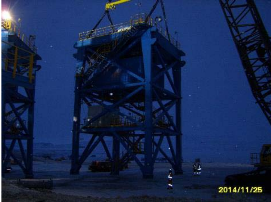
PHOTO 19 Conveyor Tower Moving November 2014
