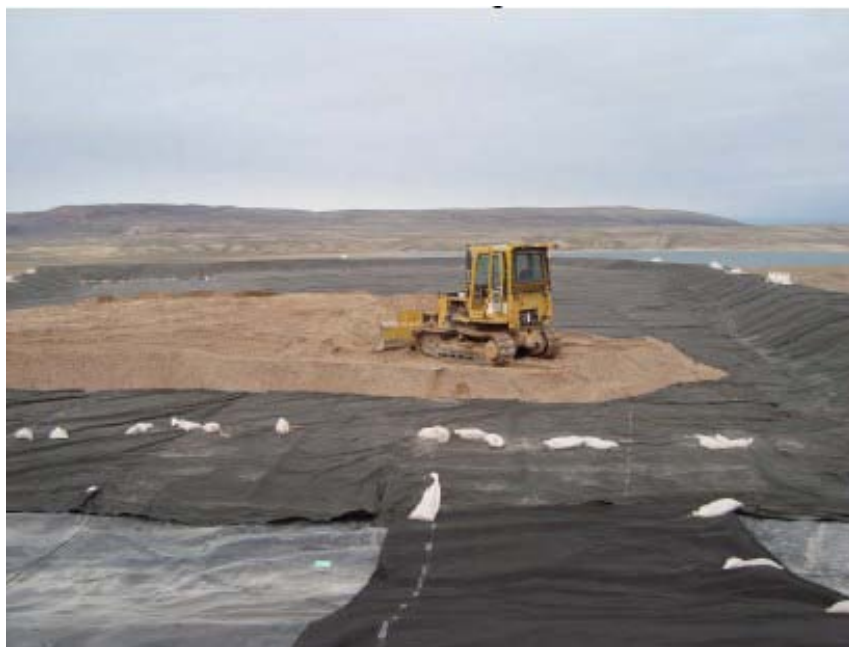
PHOTO 14 Landfarm □ Placing Liner Cover Fill
