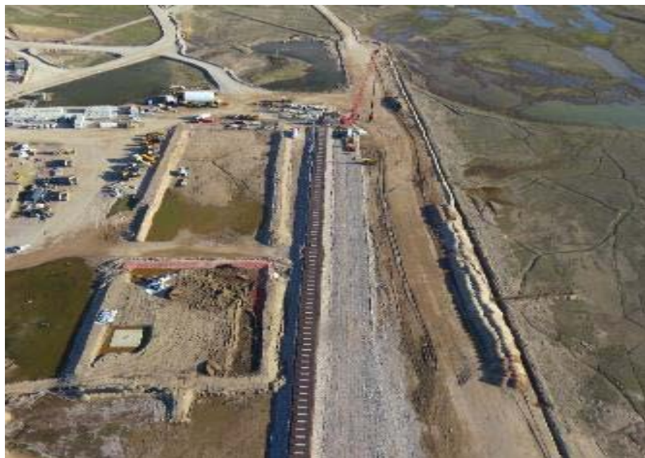
PHOTO 15 Aerial View □ Conveyor Construction and Bladder Farm Decommissioning August 2014
