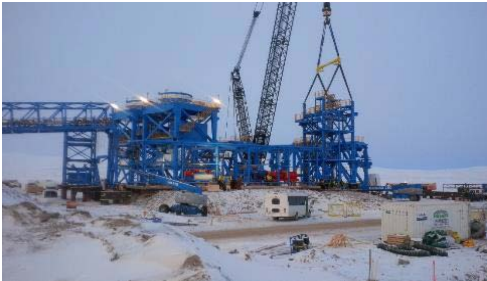
PHOTO 18 Drivehouse Construction November 2014
