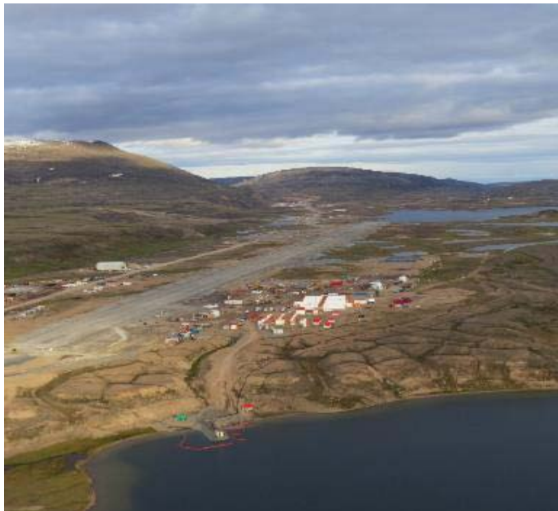
PHOTO 4 Mary River Mine Site Air Strip Construction Completed ᐸᓗᓕᓂ ᐅᓕᓕᓂᐸᓕᐸᐸᐸ ᐸᓕᐸᓕ ᓴᐸᓕᓂᓕ ᐱᓕᓕᓕᐸᓕᐸᓕ
