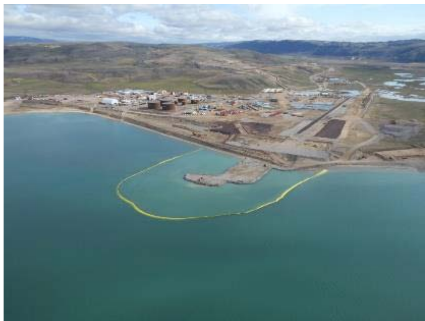
PHOTO 3 Aerial View □ Ore Dock Construction June 2014 ᐱᐃᐃᐃᐃᐃ 3 ᐃᐃᐃᐃ ᐃᐃᐃᐃ – ᐃᐃᐃᐃᐃᐃᐃᐃ ᐃᐃᐃᐃᐃᐃᐃ ᐃᐃᐃᐃᐃᐃᐃ ᐃᐃ 2014
