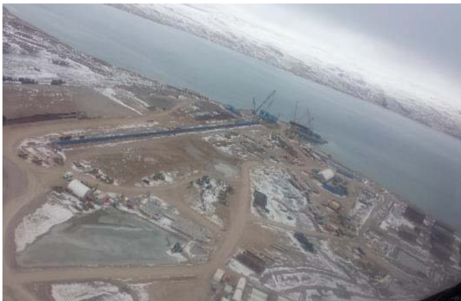
PHOTO 16 Aerial View □ Conveyor Construction □ Bladder Farm Decommissioning Complete September 2014
