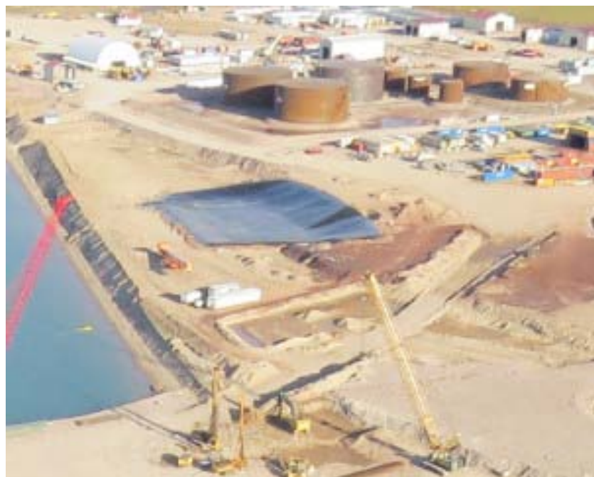
PHOTO 10 Settling Pond 2 (East pond) Aerial View ᐸᑦᓴᕈᖅ 10 ᐃᔪᒃᓱᓄᑦᐸᔭᐳᓂᓯᓵᑐᑦ ᐸᑦᓴᕈᖅ 2 (ᐆᕋᕋᑦᐸ ᐸᑦᓴᕈᖅ) ᓫᑦᑦᑦ ᐸᑦᓴᕈᖅ
