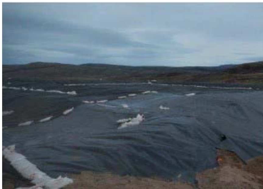
PHOTO 13 Landfarm □ Contaminated Snow Cell - Liner ballasted in place with sand bags ready for seam sealing
