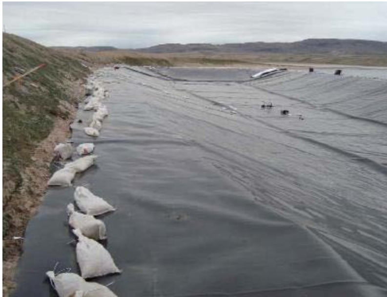
PHOTO 7 Settling Pond 1 (West pond) Construction ᐅᓂᔭᑦ ᐃᕈᒪᐱᖁᑎᓄᗇ ᐊᓚᓴᐸᓯᓰᓄᗛ ᐆᓵᐳᓴᓴᓄᗛ (ᐱᕋᓴᓴᓄᗛ ᐆᓵᐳᓴᓴᓄᗛ) ካᓚᓲᓶᑏᓴᓴ
