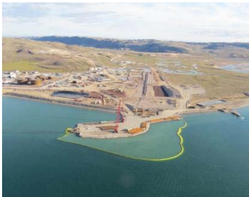
PHOTO 4 Aerial View □ Ore Dock Construction August 2014 ᐱᐃᐃᐃᐃᐃ 4 ᐃᐃᐃᐃ ᐃᐃᐃᐃ – ᐃᐃᐃᐃᐃᐃᐃᐃ ᐃᐃᐃᐃᐃᐃᐃᐃ ᐃᐃᐃᐃᐃᐃᐃ ᐃᐃᐃᐃ 2014
