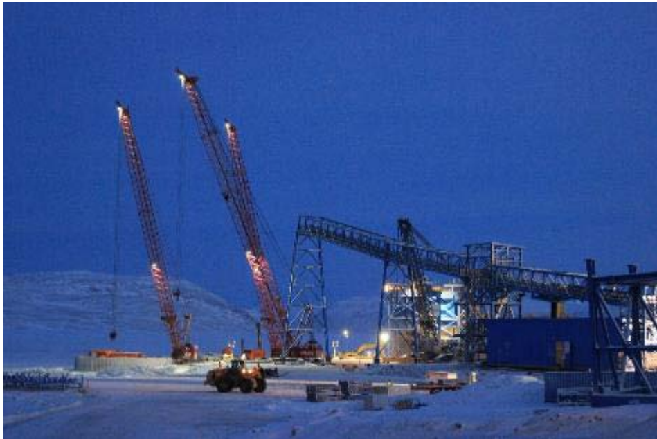
PHOTO 20 Conveyor Construction December 2014
