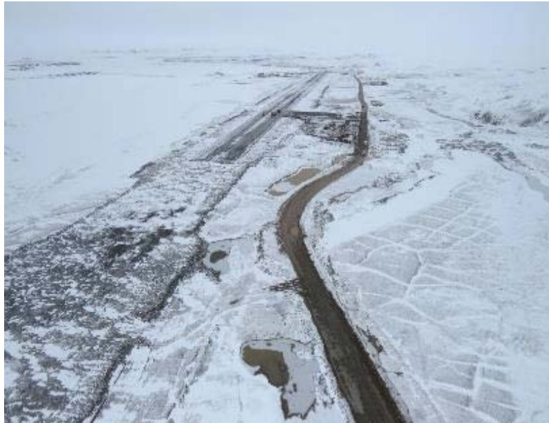
PHOTO 3 Mary River Mine Site Air Strip Construction ᐸᓗᓕᓂ ᐅᓕᓕᓂᐸᓕᐸᐸᐸ ᐸᓕᐸᓕ ᓴᐸᓕᐸᓕᐸᓕ
