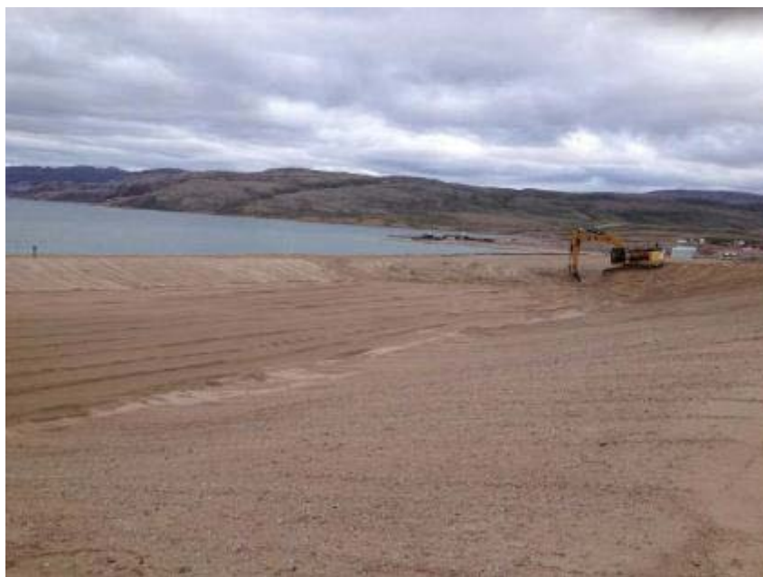
PHOTO 9 Settling Pond 2 (East pond) Construction ᐅᓄᑦᕈᑦ ᐱᓂᓃᑦᕈᑦ 2 (ᔭᒃᕆ ᐱᓂᓃᑦᕈᑦ) ᐸᓚᐸᓇᕐᑐᑦ (ᔭᒃᕆ ᐱᓂᓃᑦᕈᑦ) ᓴᓗᕐᕋᐸᓇᕐᑐᑦ
