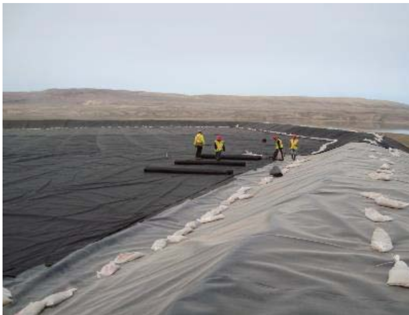
PHOTO 12 Landfarm □ installation of Liner
