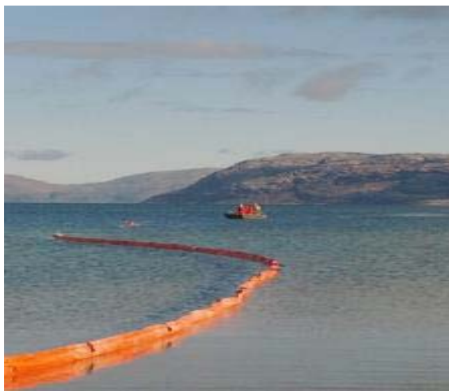
PHOTO 4 Deploying a containment boom during the Marine Spill Response Training August 2014
