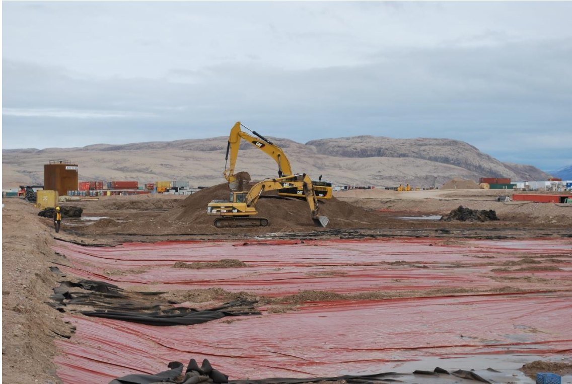
Photo 5 – Transferring the Contained Contaminated Soil to the North End of the Containment Berm
