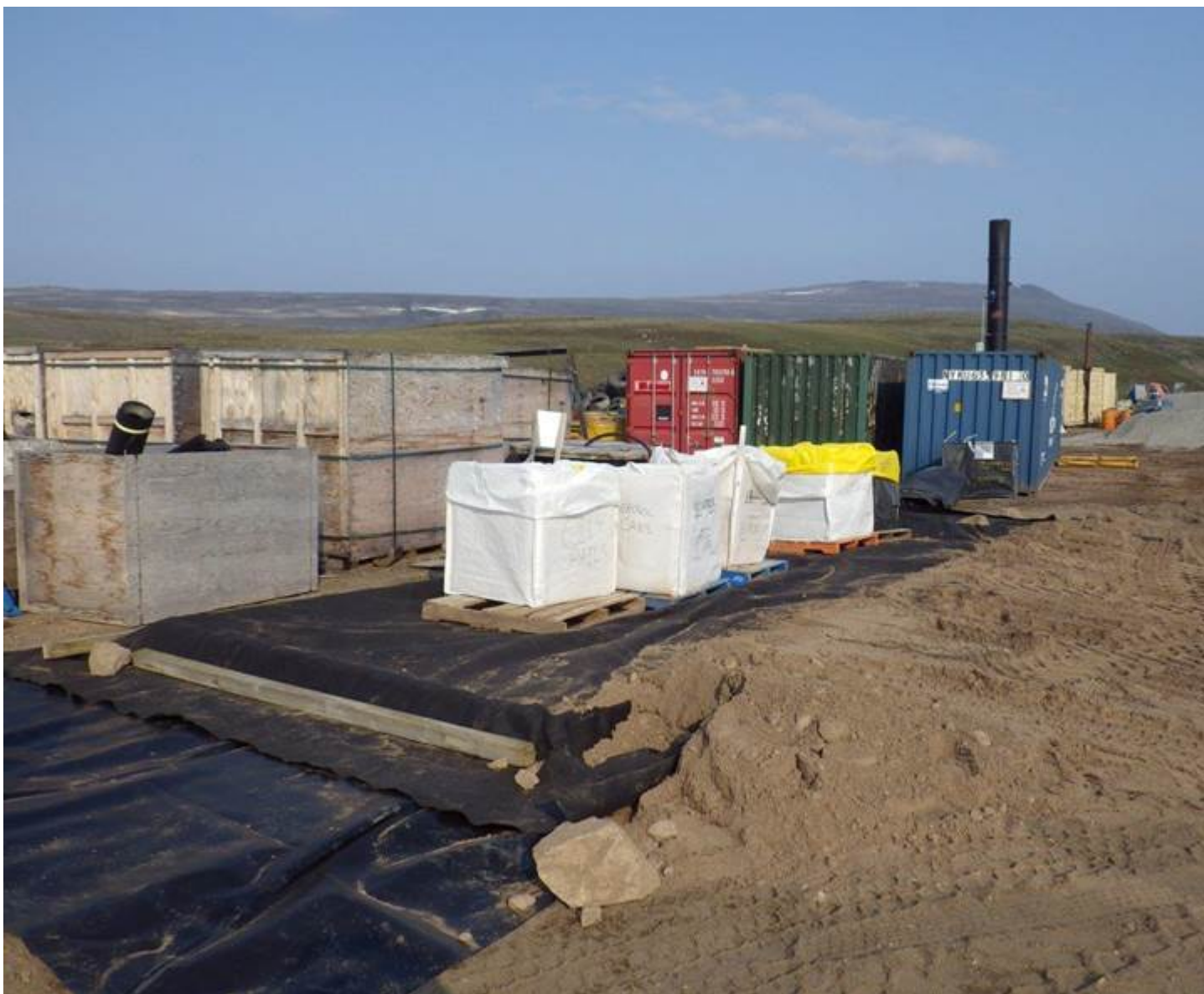
Photo 4: Hazardous Waste Sorting Area near the Incinerator in Lined Secondary Containment
