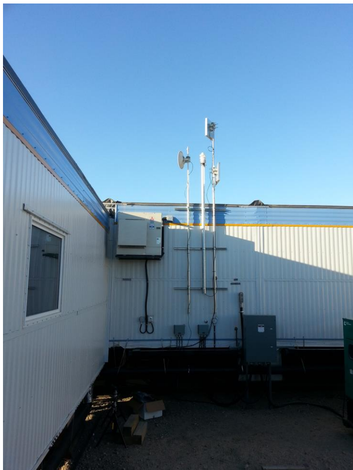
Figure 12: Mary River camp WS600-UMB sensor installed on outside wall of server room trailer
