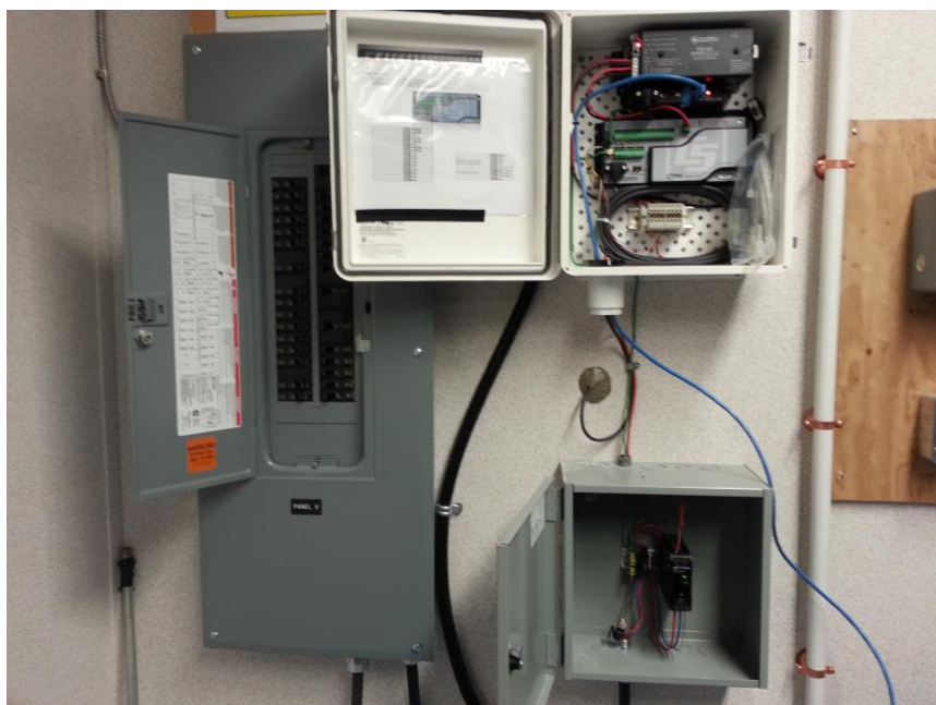
Figure 13: Inside Mary River camp datalogger enclosure and sensor power supply enclosure
