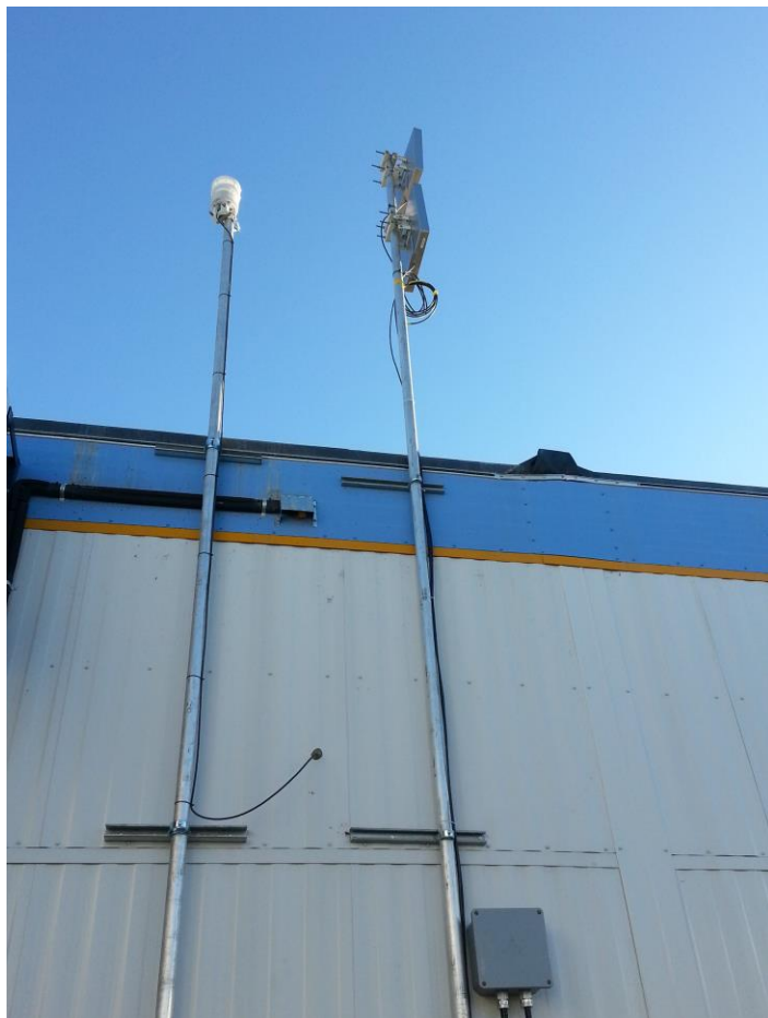
Figure 9: Milne camp WS600-UMB sensor installed on the outside wall of server room trailer
