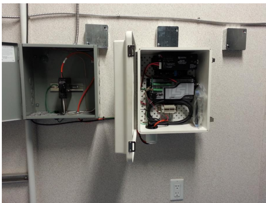
Figure 10: Inside Milne camp datalogger enclosure and sensor power supply enclosure
