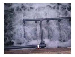
Proper air scouring in membrane tank
