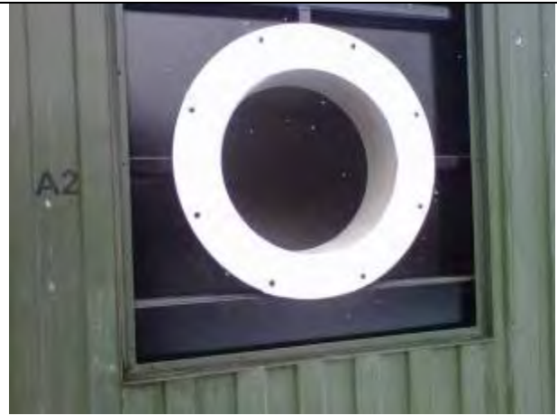
Correctly Installed Gasket
