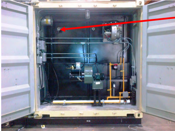
1. Primary Thermocouple (TC1)
