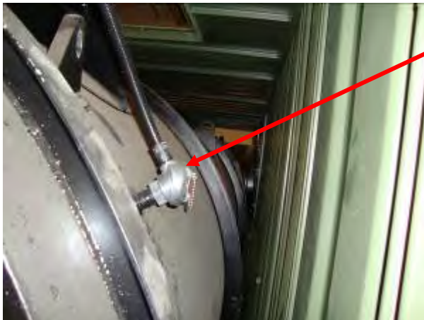
2. Secondary Thermocouple (TC2) on Secondary Chamber Container
