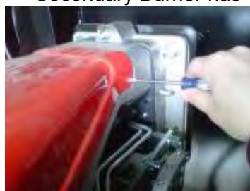
Secondary Burner has 4 screws (2 on each side)
