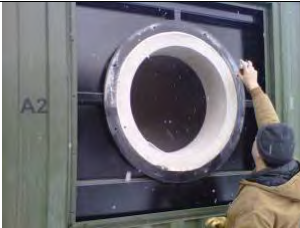
Gasket adhesive spray being applied
