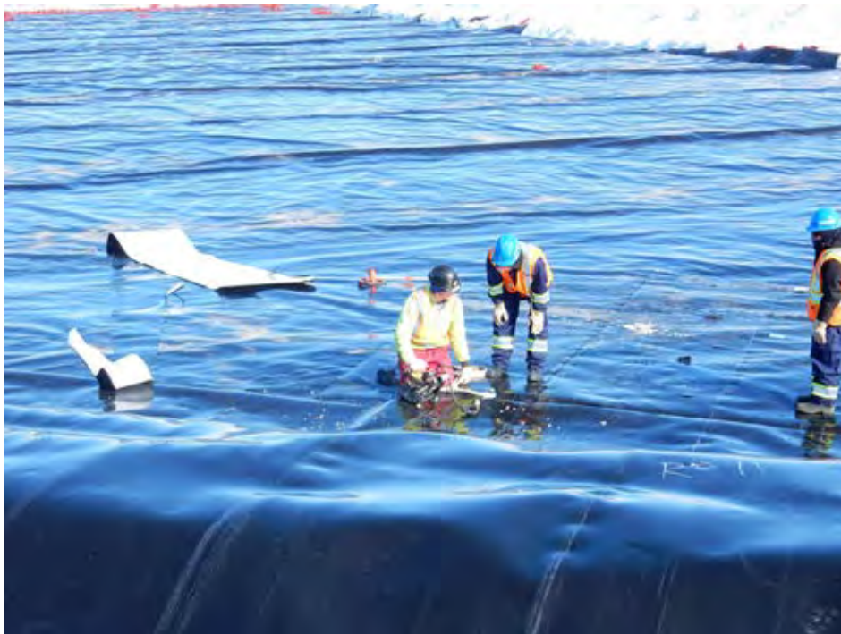
Figure 7: Seam Welding Liner
