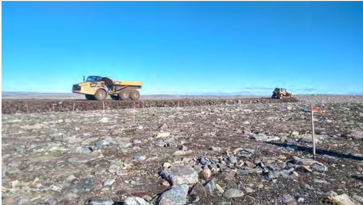
Figure 2: Fill Placement for Berm Construction
