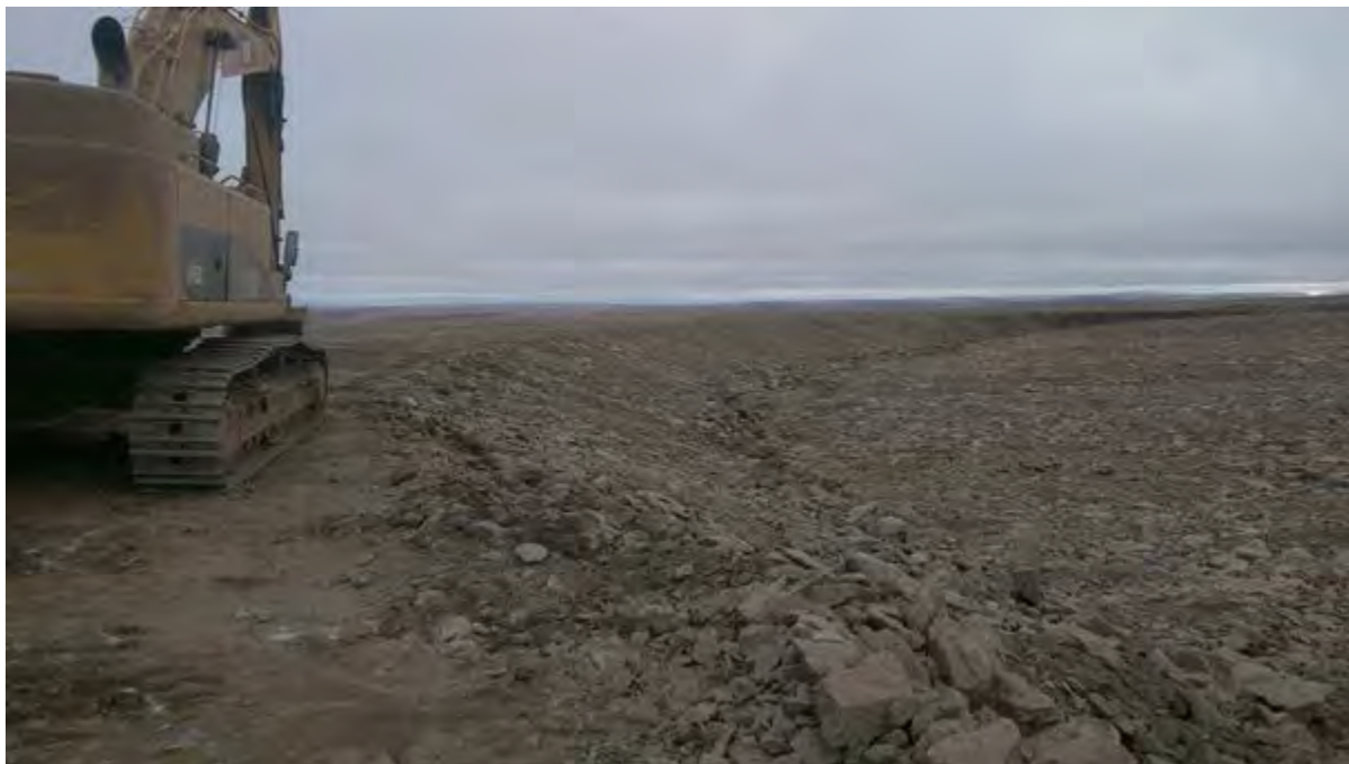
Figure 3: Berm after Fill Placement
