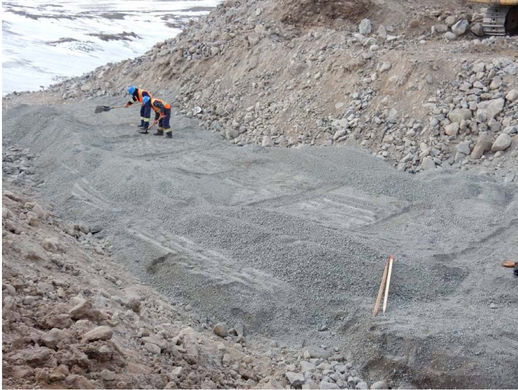
Culvert CV-1 Construction and Installation Photos – May 2016
