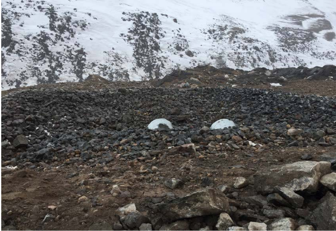
Culvert CV-1 Construction and Installation Photos – May 2016
