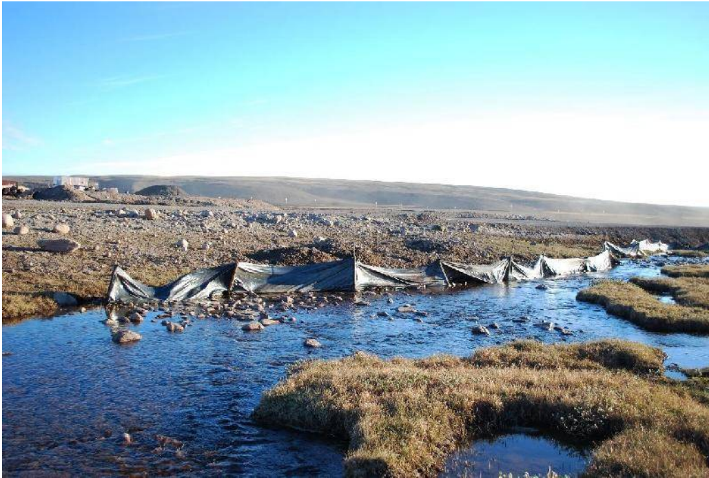
Photo 1 – Silt fence installation along road to prevent road runoff from directly discharging into Sheardown Lake Tributary (SDLT) near CV186.
