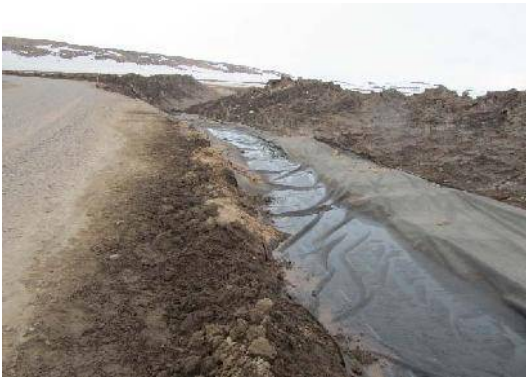
Constructed Drainage Controls Partially Implemented or Completed.
