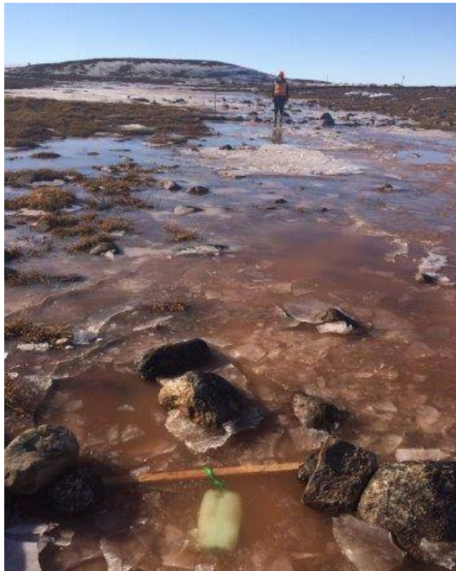
Photo 2 – May 9 th 2016. Floculant stations installed along Sheardown Lake Tributary SDLT and LDFG.
