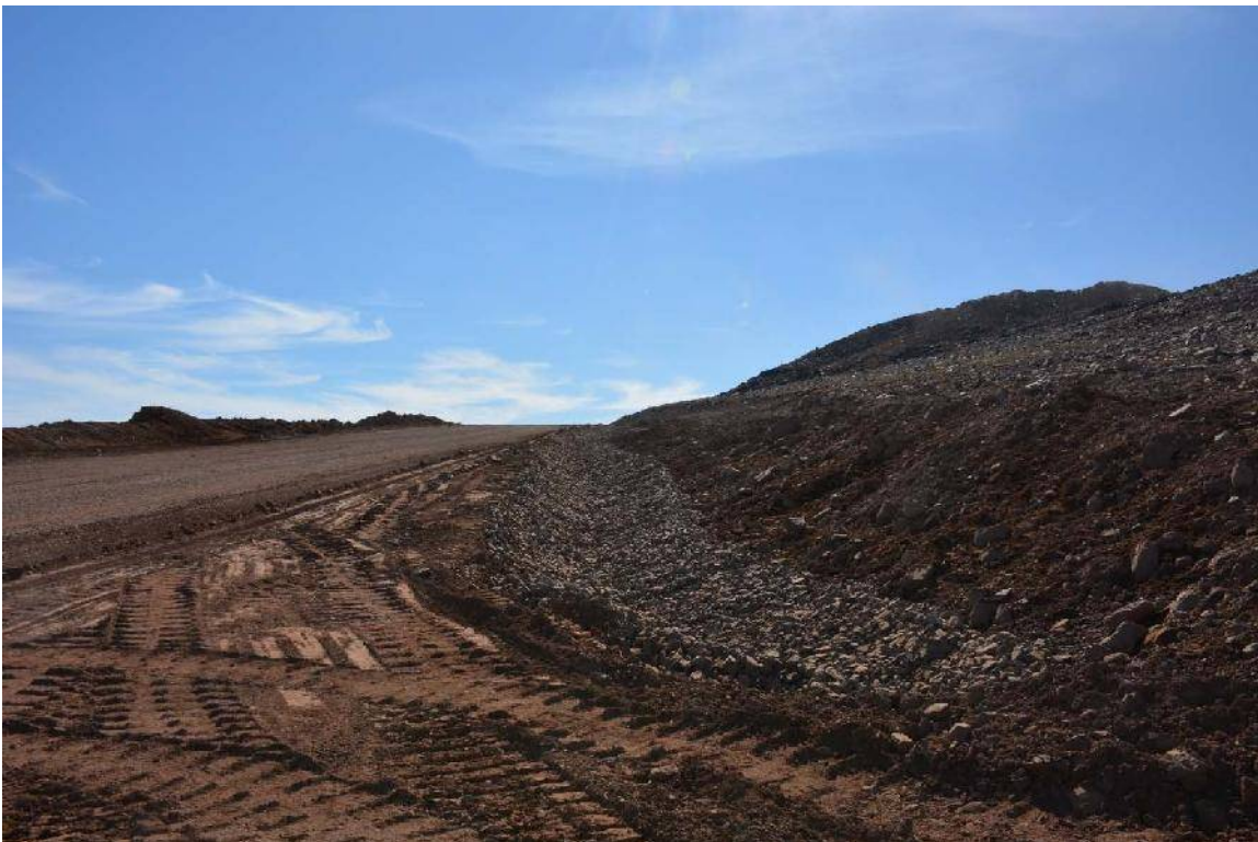
Photo 4 - New ditch with geotextile and rip rap at downhill from Km 108.5. Picture taken on July 5, 2016
