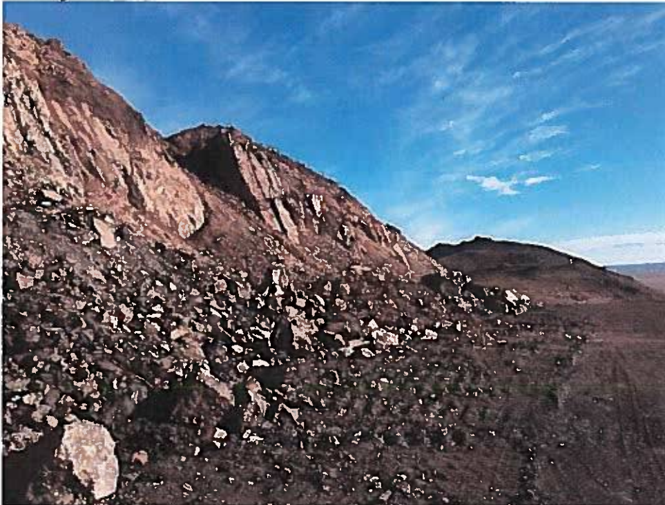
Photo 4: 10m high internal wall on outside edge of 640 Bench. Overburden across top of bench is raveling now that it has thawed.
