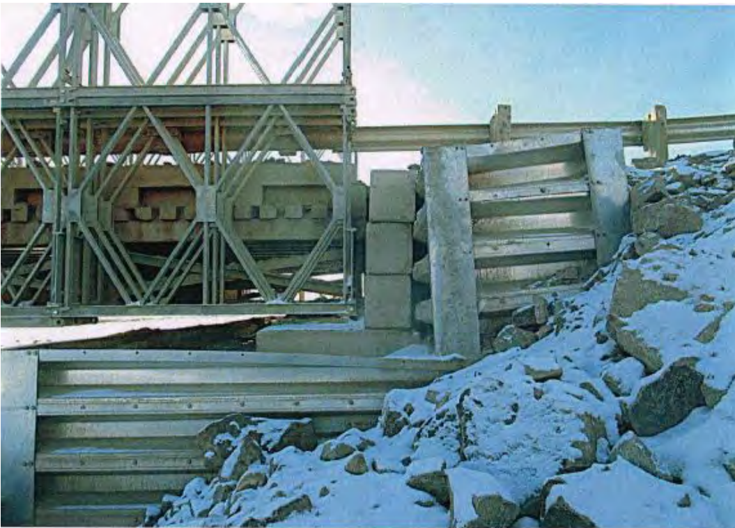
33. Bridge Abutment @ km 63 (Note Space)
