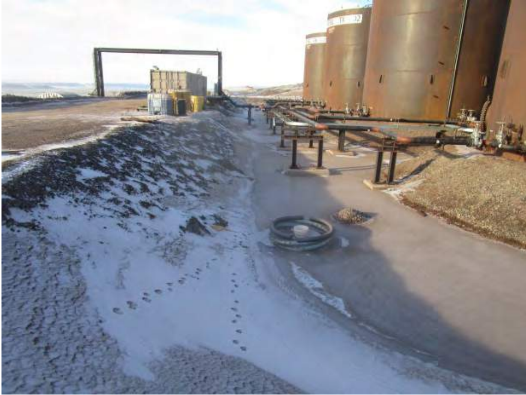
15. Mine Site Steel Fuel Tank Farm Containment.
