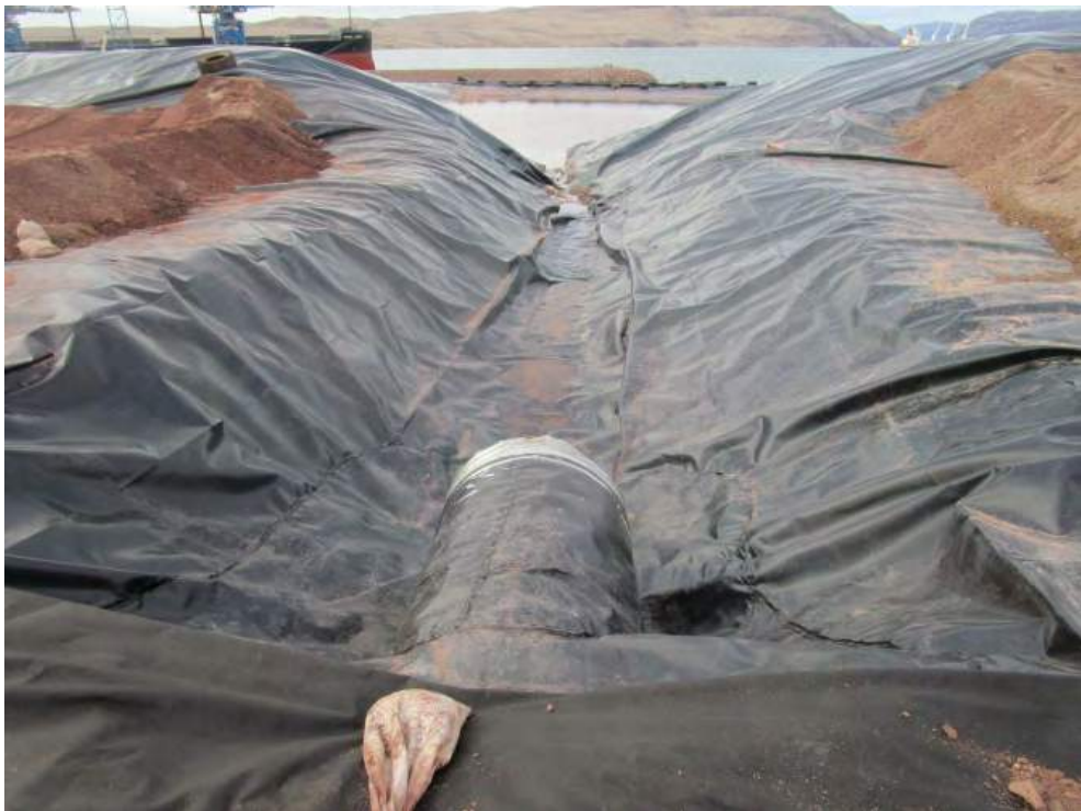
28. Sedimentation Pond East - Liner at south inlet
