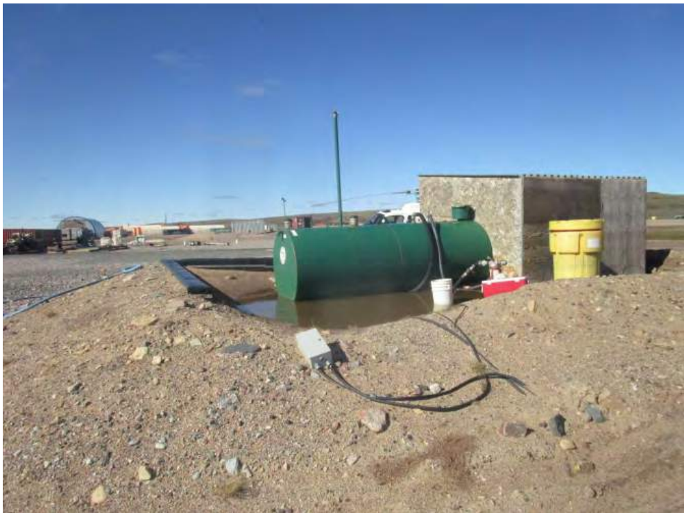
6. Helicopter Fuel Tank Containment
