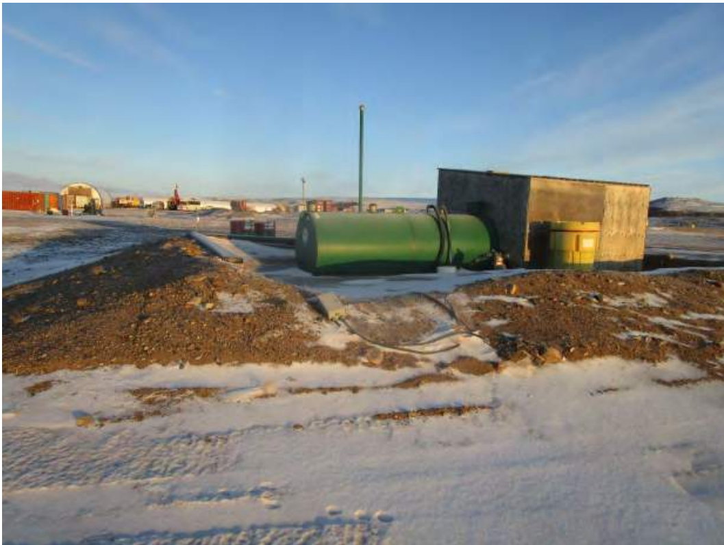
6. Helicopter Fuel Tank Containment.
