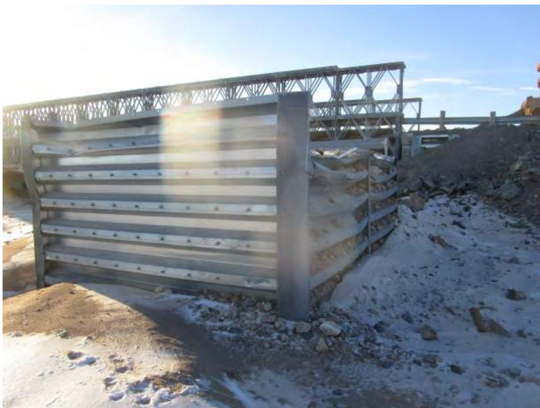
39. Sea can bridge abutments no longer in use. Note there is no deformation.
