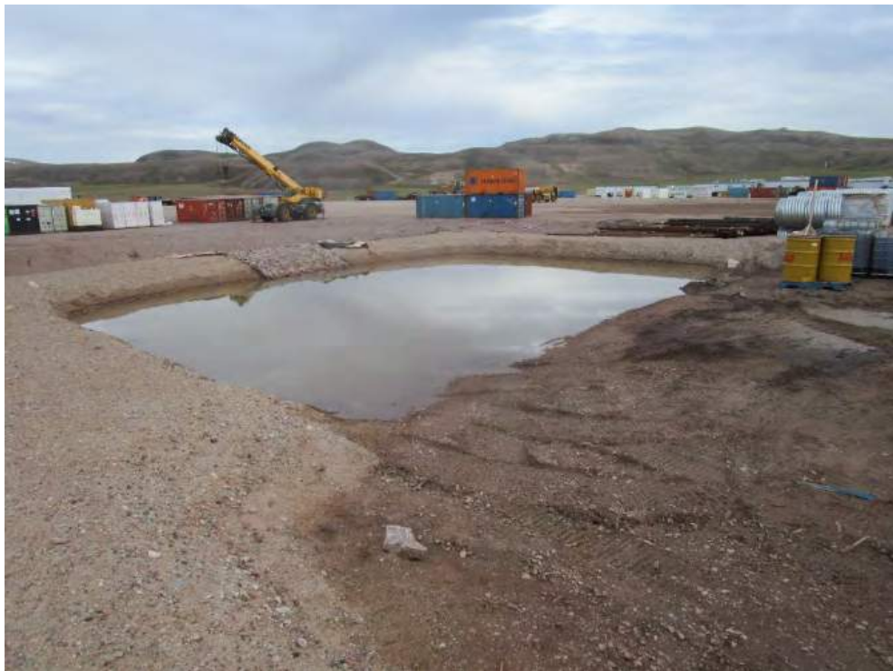
2. Generator Fuel Containment
