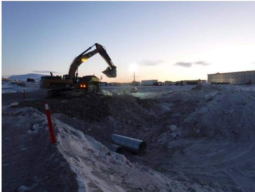
Figure 21. CV186 DS culvert installation 17-11-27
