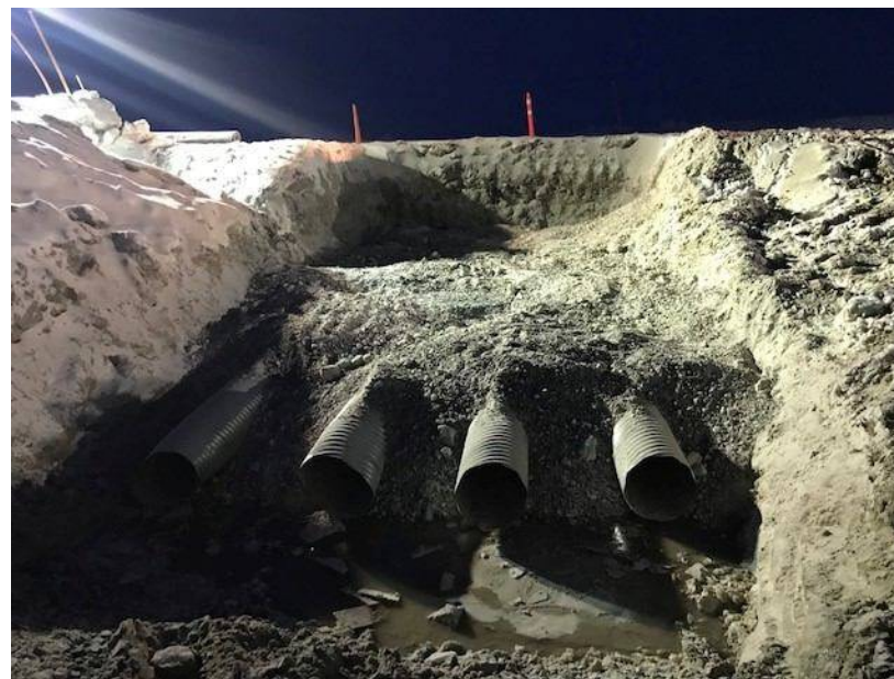
Figure 11. CV059 DS during culvert replacement 17-12-18
