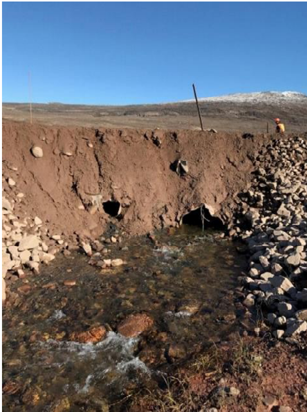
Figure 19. CV186 DS pre-culvert extension 17-09-02
