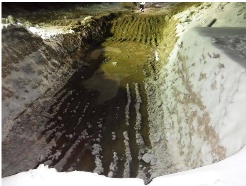
Figure 10. CV059 DS after historical culvert removal 17-12-09
