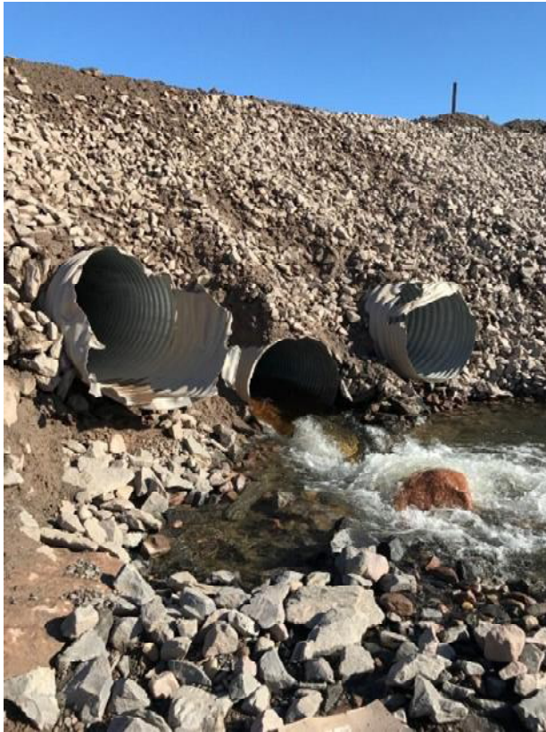
Figure 1. BG01 DS pre-construction 17-09-02
