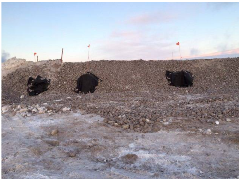
Figure 18. CV112 DS post-culvert extension 17-11-04
