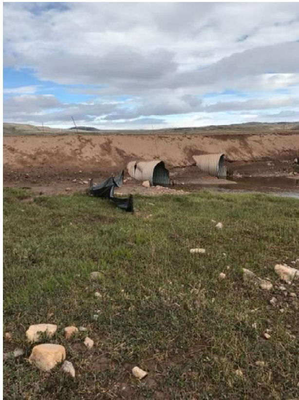
Figure 7. BG32 DS pre-culvert extension 17-07-24
