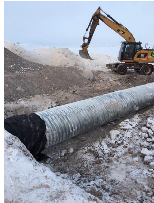
Figure 17. CV112 DS culvert extension installation 17-11-04
