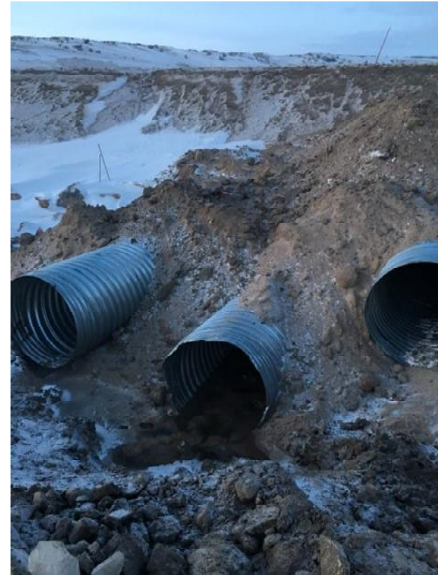
Figure 2. BG01 US mid-installation 17-10-05
