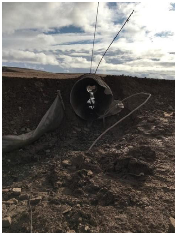
Figure 14. CV106 DS pre-culvert extension 17-09-11
