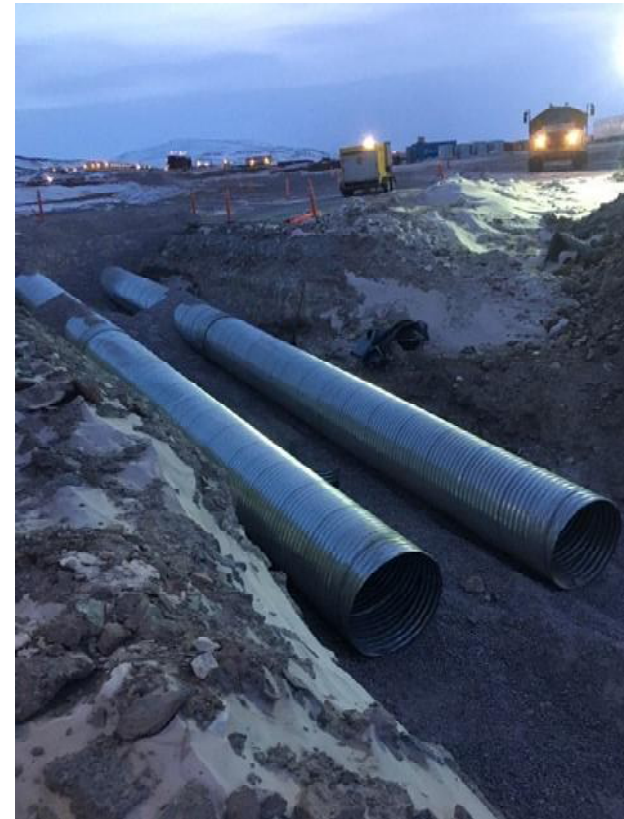
Figure 20. CV186 DS culvert extension 17-11-28
