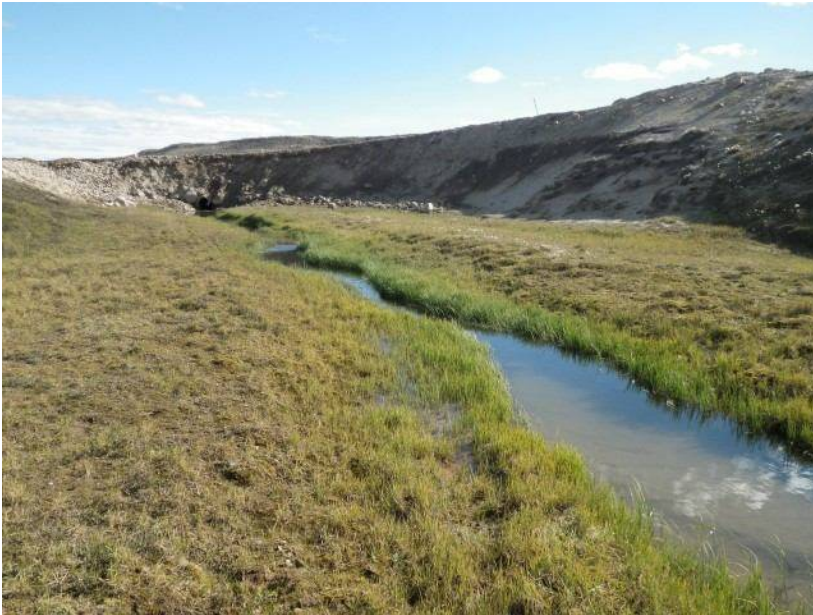
Figure 4. BG29 DS pre-culvert extension 16-08-12
