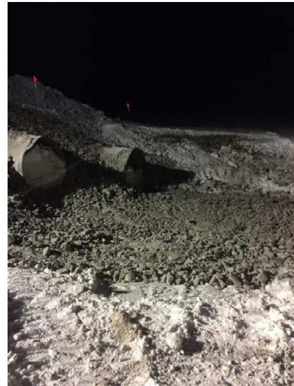
Figure 13. CV099 DS post slope embankment reinforcement 17-12-03
