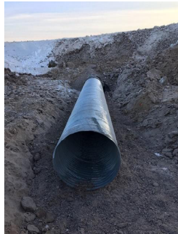
Figure 5. BG29 DS culvert extension installation 17-11-07
