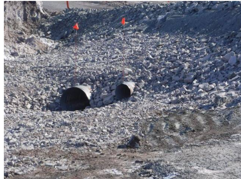
Figure 26. CV187 DS culvert extension completed 17-04-24
