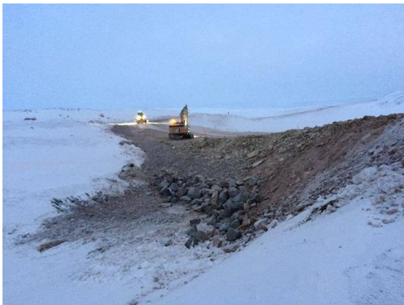
Figure 6. BG29 DS culvert extension installed 17-11-09
