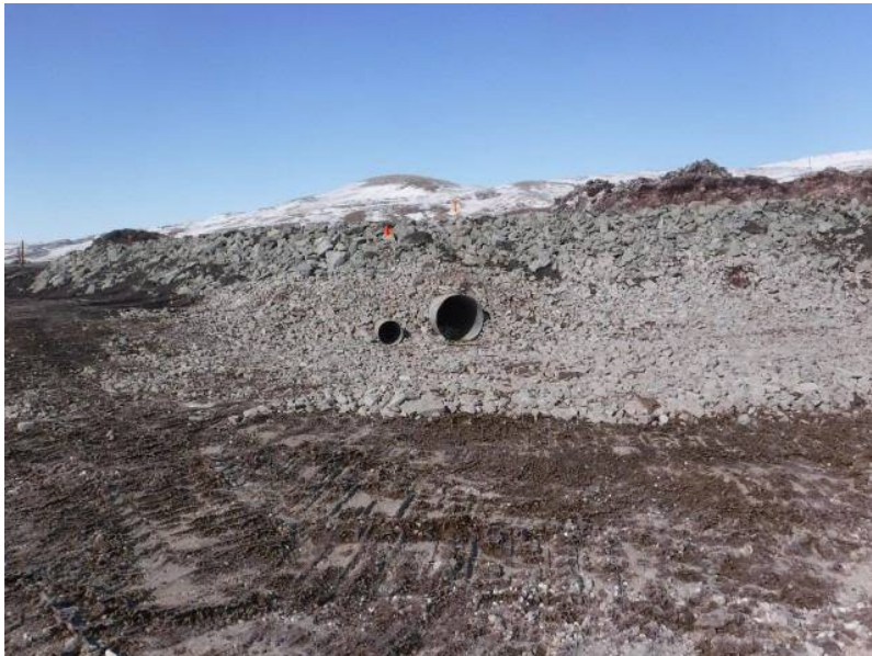
Figure 25. CV187 US culvert extension completed 17-04-24
