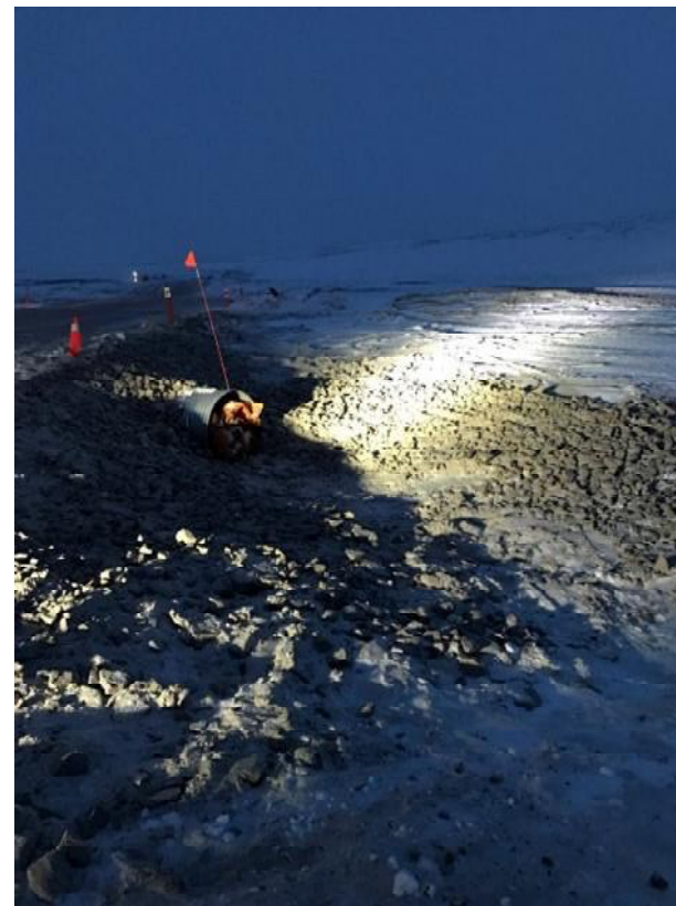
Figure 15. CV106 DS post-culvert extension 17-12-03
