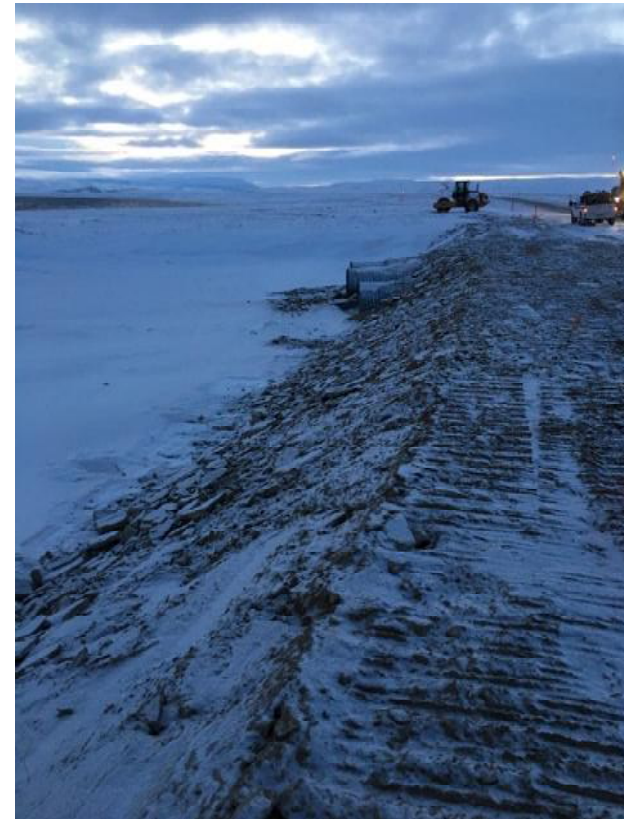
Figure 28. CV216 DS post-culvert extension 17-10-05
