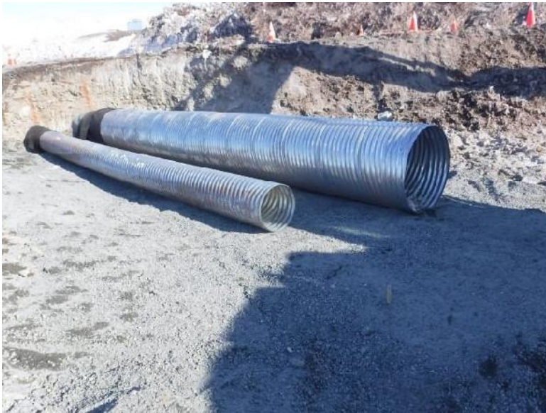
Figure 23. CV187 US culvert extension 17-04-23
