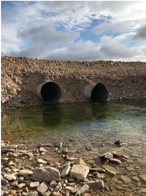
Figure 12. CV099 DS pre slope embankment reinforcement 17-09-11
