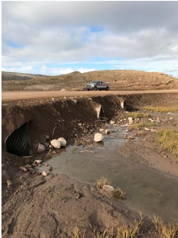
Figure 16. CV112 DS pre-culvert extension 17-09-11
