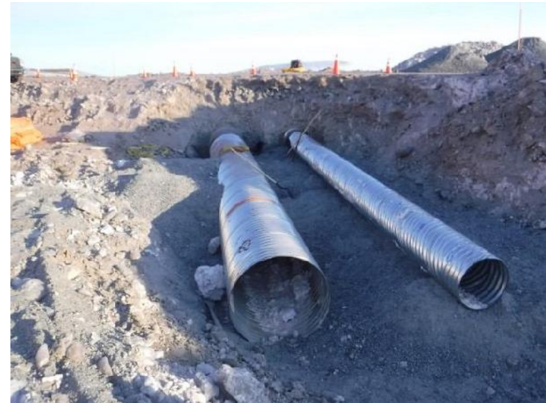
Figure 24. CV187 DS culvert extension 17-04-20
