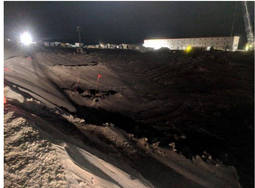
Figure 22. CV186 DS culvert extension completed 17-12-01
