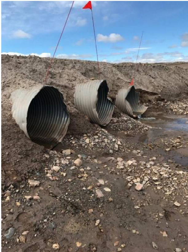
Figure 27. CV216 DS pre-culvert extension 17-07-24
