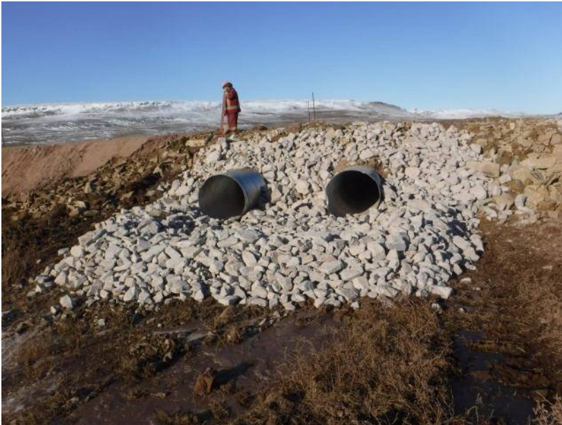
Figure 9. BG 32 DS culvert extension completed 17-09-23
