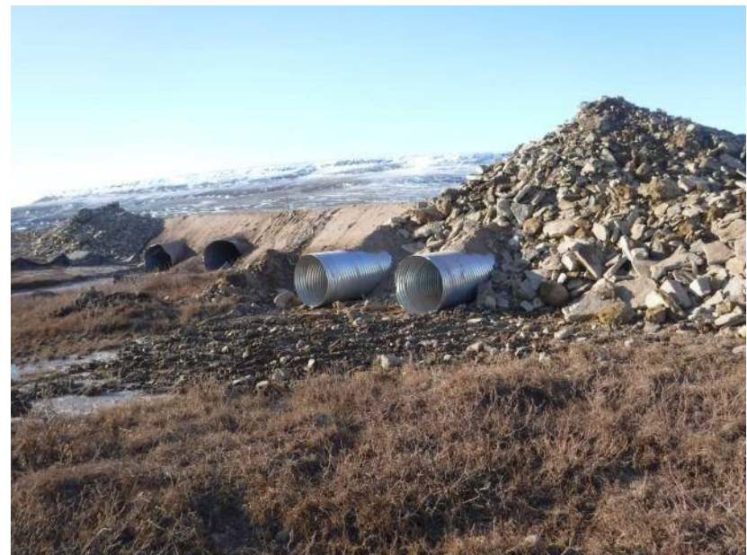
Figure 8. BG32 DS mid-culvert extension installation 17-09-22
