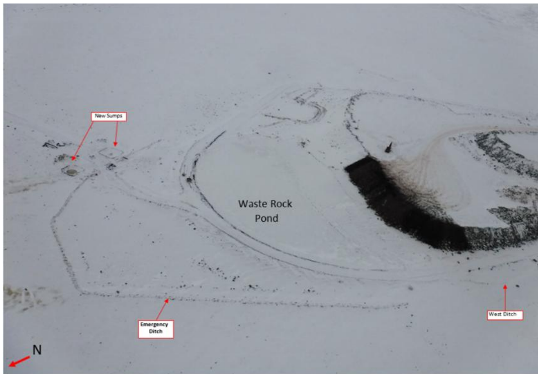
PHOTO 15 – Waste Rock Facility with emergency ditches/sumps constructed down-gradient to contain observed seepage – September 2017
