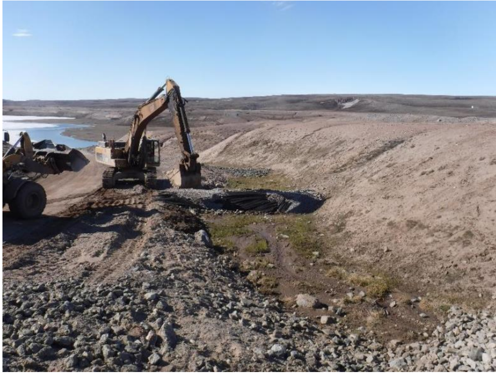
PHOTO 9 – Construction of check dams along Camp Lake Access Road – June 2017
