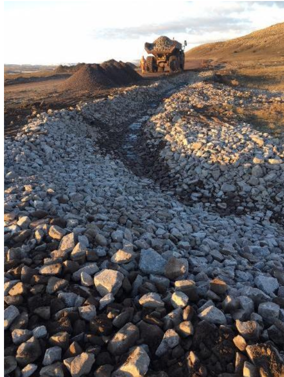
PHOTO 6 – Armouring of roadside ditching near Km 85.5 – June 2017
