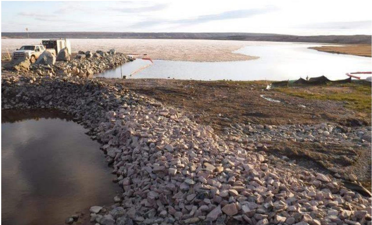
PHOTO 11 – Maintenance work completed on Camp Lake check dams – June 2017
