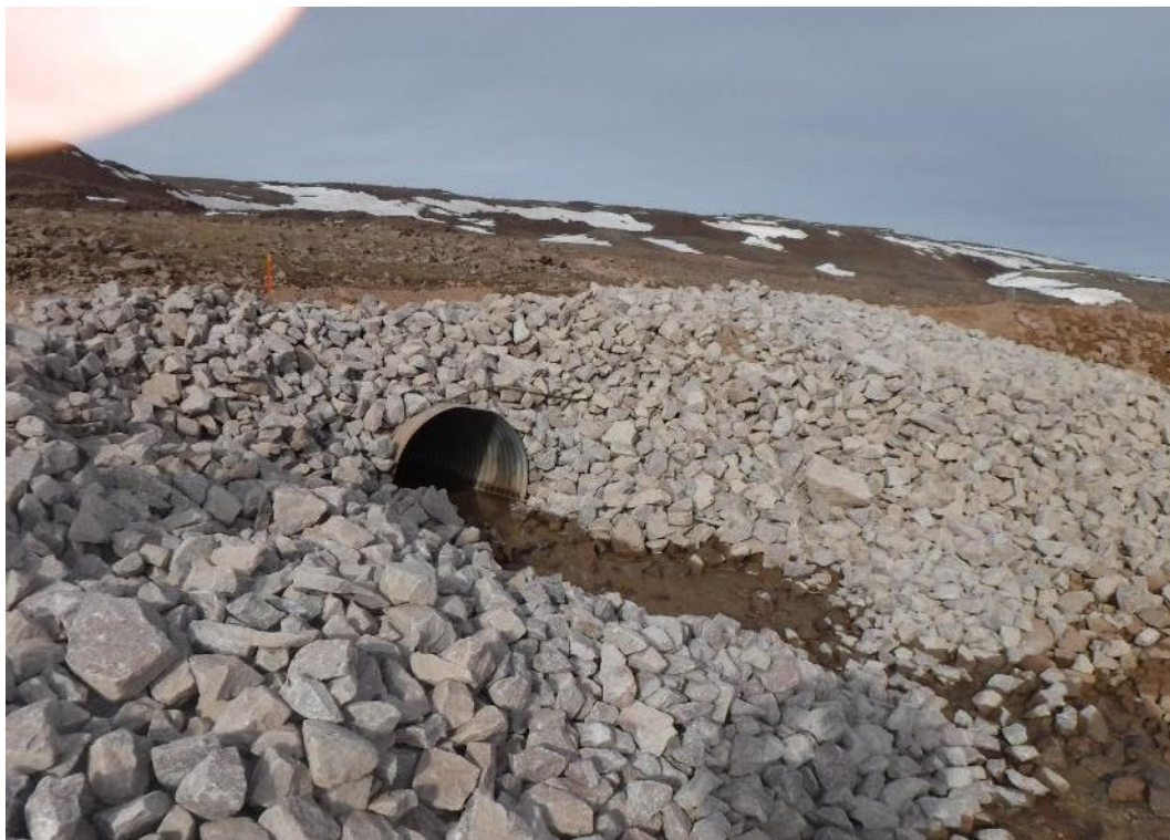
PHOTO 2 - Placement of aggregate to reinforce embankment near CV-174 outlet - June 2017
