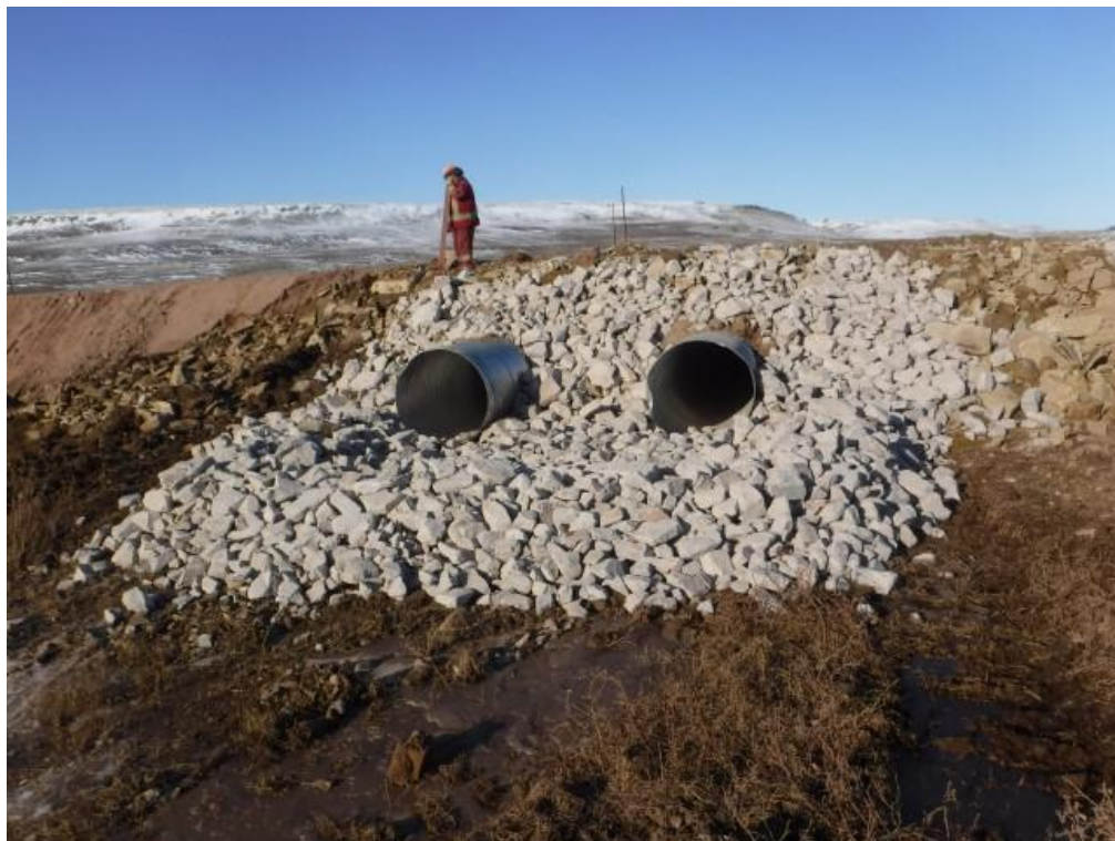
PHOTO 4 – Replacement of culverts at BG-32 - September 2017
