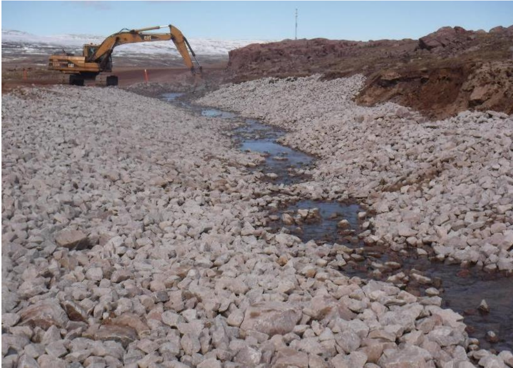
PHOTO 3 – Armouring of ditching near CV-174 – June 2017
