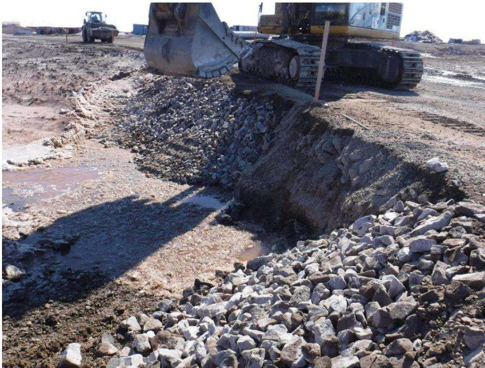
May 23, 2017 – Armouring road embankment near culvert CV-186 (Sheardown Lake Tributary)
