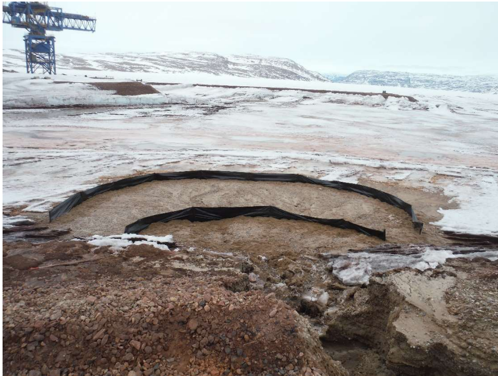
May 26, 2017 – Silt fences installed to contain sediment released from bank erosion as a result of Milne Port East Sedimentation Pond (MP-05) overflow on May 25, 2017
