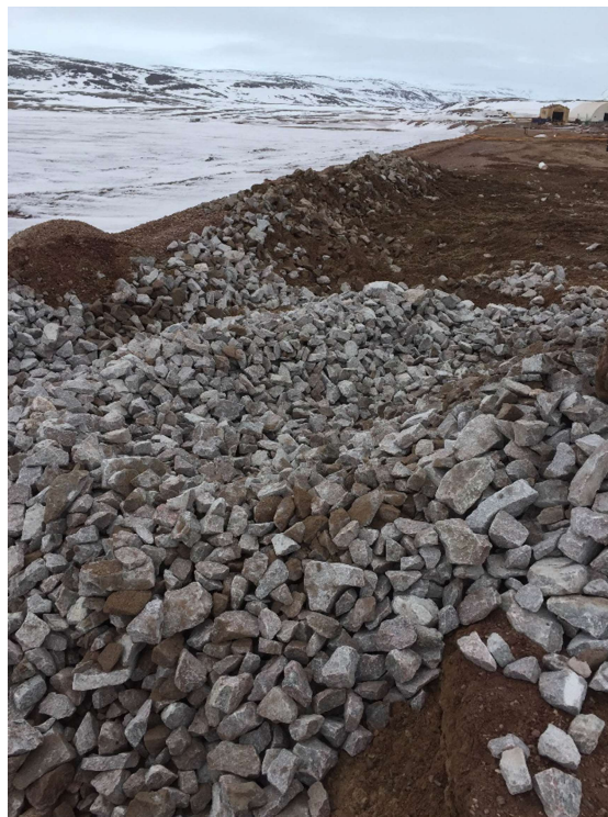
May 26, 2017 – Areas of bank erosion armoured with aggregate (rip-rap)
