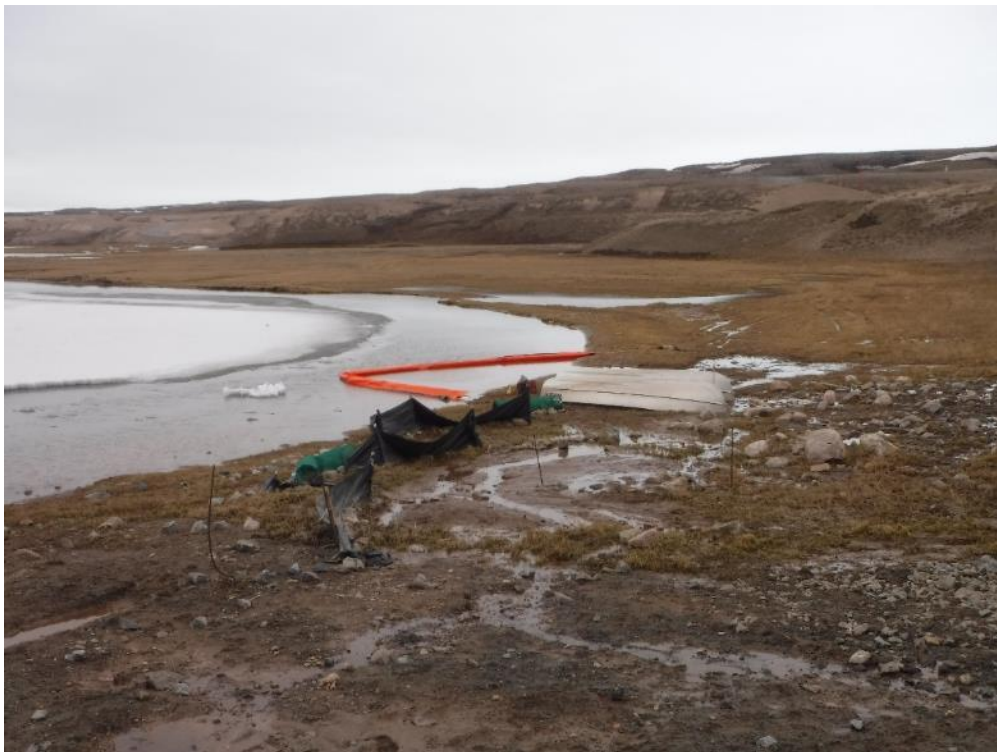
June 11, 2017 – Installation of silt curtain and additional silt fences and spring berms at the outlet of Camp Lake Sedimentation Ponds
