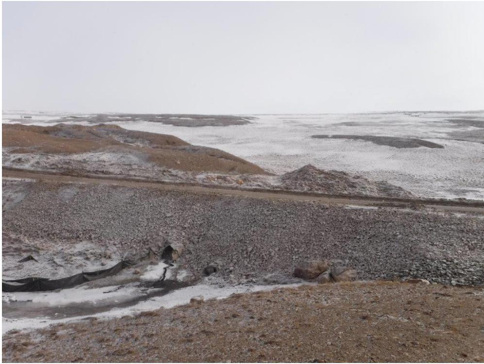
May 21, 2017 – Armouring of road embankments near culvert BG-01 (Camp Lake Tributary 1)
