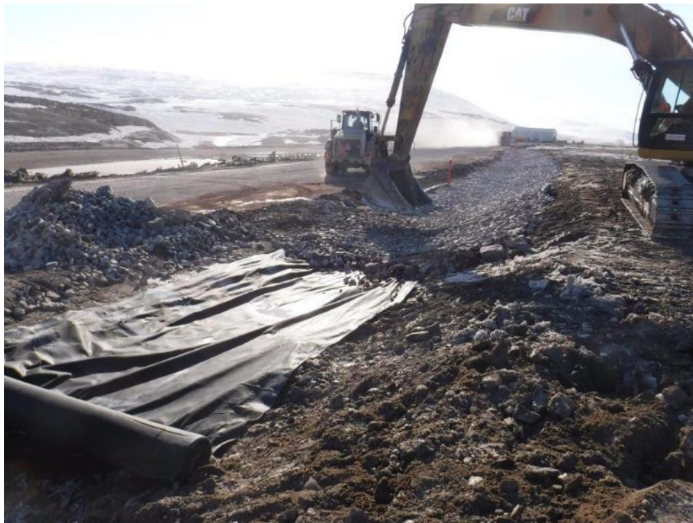
May 23, 2017 – Armouring of drainage ditch on north end of Mine Site airstrip near Km 100 (upstream of Camp Lake Tributary 1)
