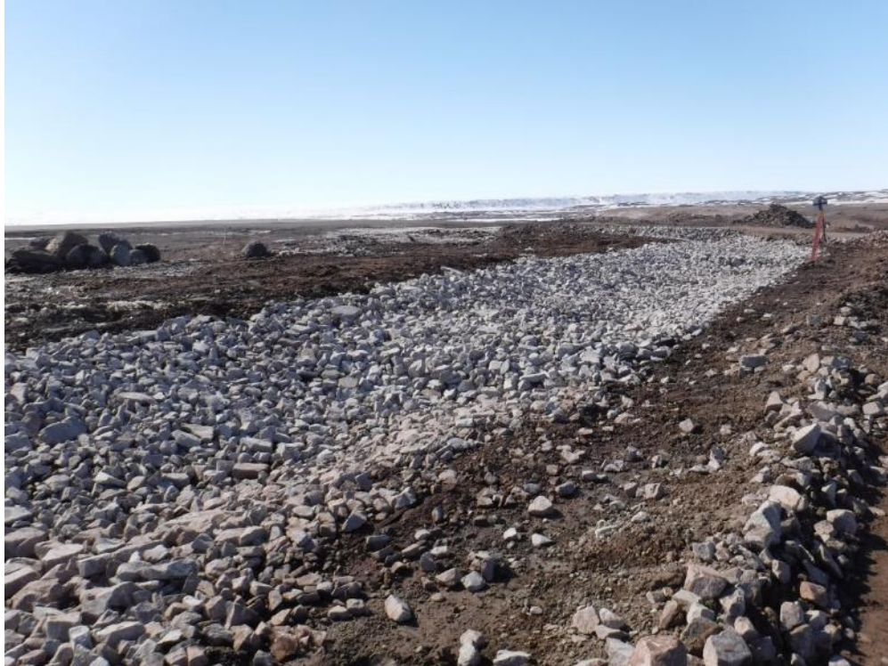
May 23, 2017 – Completion of drainage ditch armouring on the north end of Mine Site airstrip near Km 100 (upstream of Camp Lake Tributary 1)
