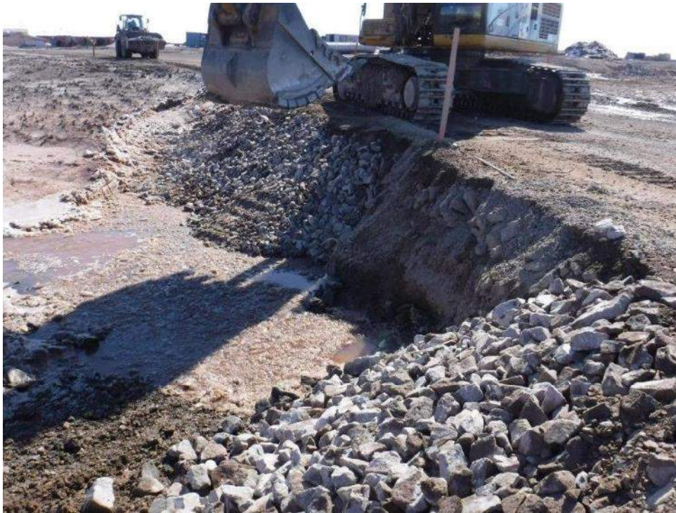
May 23, 2017 – Armouring road embankment near culvert CV-186 (Sheardown Lake Tributary 1)
