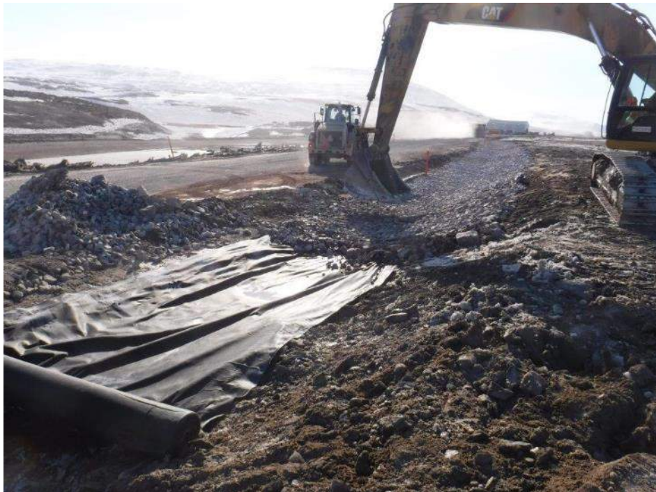
May 23, 2017 – Armouring of drainage ditch on South end of Mine Site airstrip near Km 100 (Upstream of Camp Lake Tributary 1)
