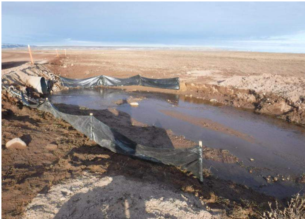
June 25, 2017 – Silt fences installed near CV-001 (downstream)
