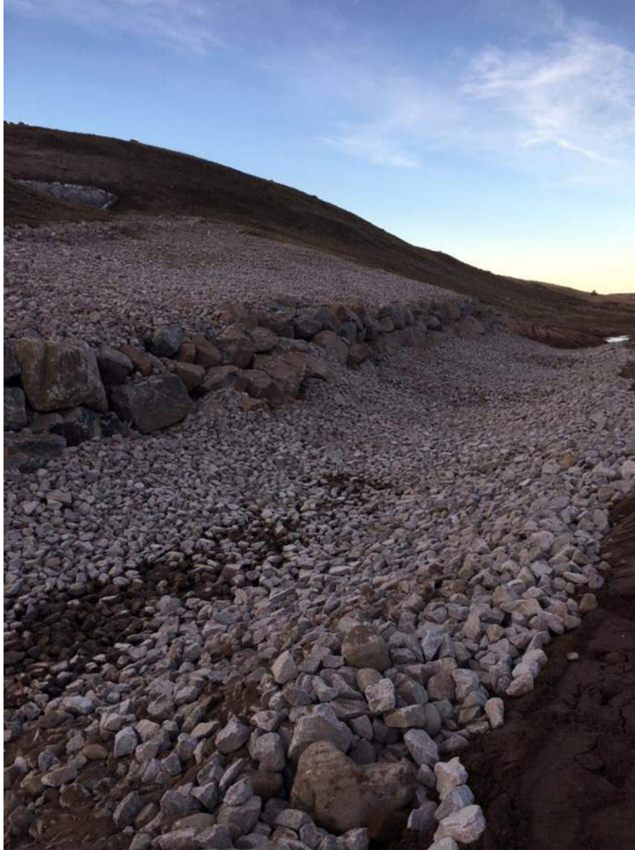
July 4, 2017 – Completion of ditch and slope armouring near Km 90
