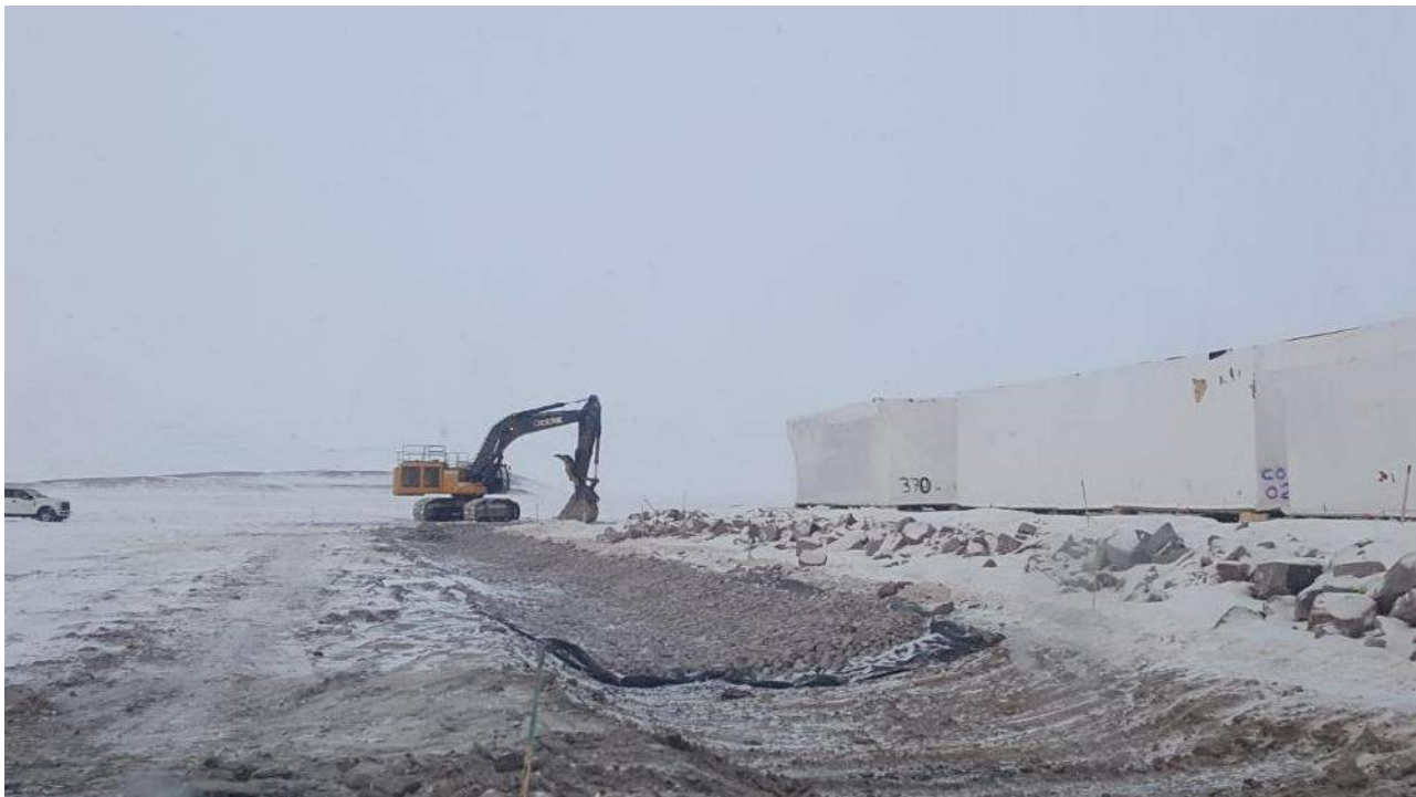
October 2017 – Construction of Milne Port Camp Pad Diversion Ditch
