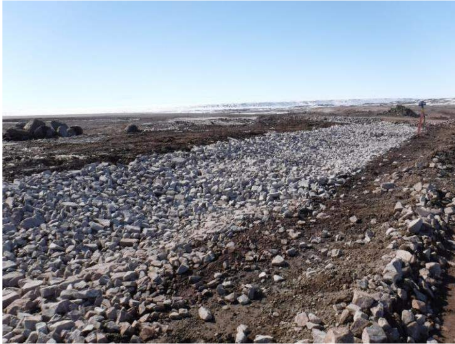
May 23, 2017 – Completion of drainage ditch armoring on South end of Mine Site airstrip near Km 100 (Upstream of Camp Lake Tributary 1)
