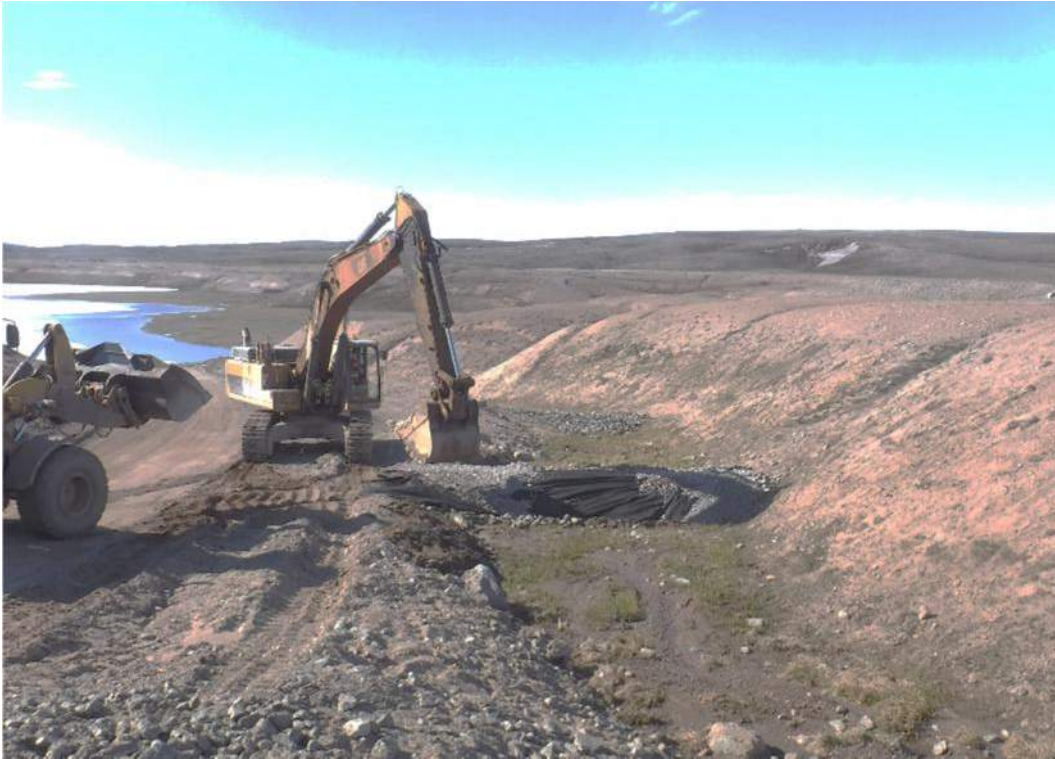
June 22, 2017 – Geotextile installation at check dams in ditch along Camp Lake Water Jetty Access Road
