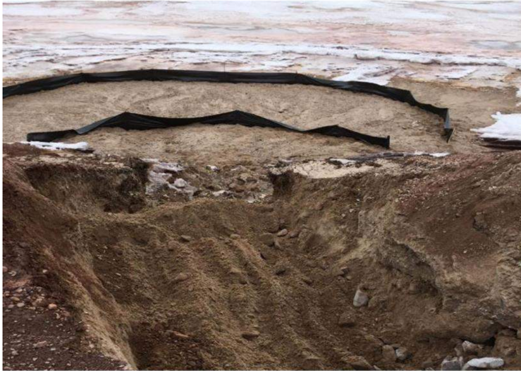
May 26, 2017 – Silt fences installed to mitigate sand washed out from MP-05 overflow
