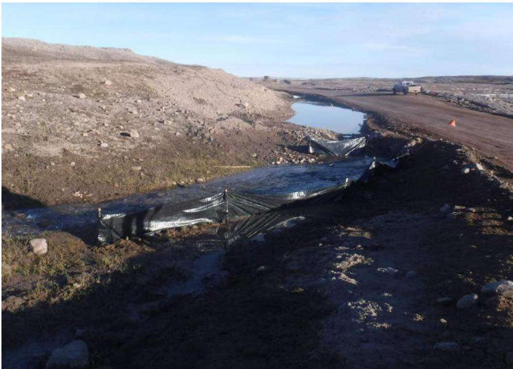
June 25, 2017 – Silt fences installed near BG-17 (upstream)
