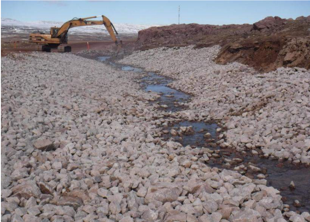
June 17, 2017 – Armouring of ditching near CV-174
