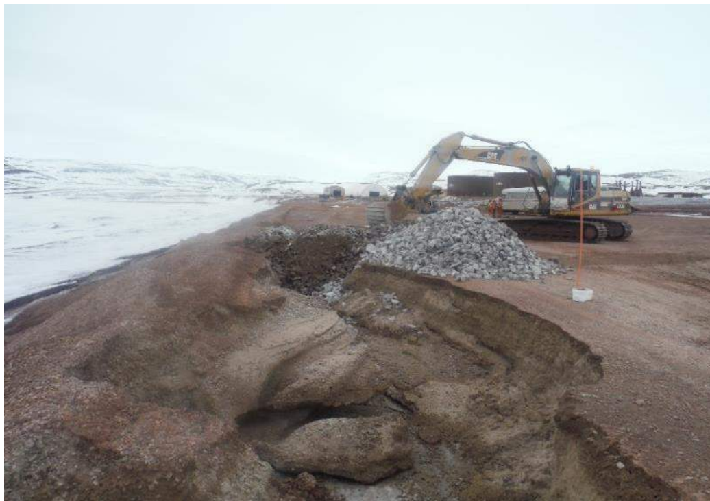
May 26, 2017 – Rip rap used to fill in beach area that was eroded by MP-05 overflow
