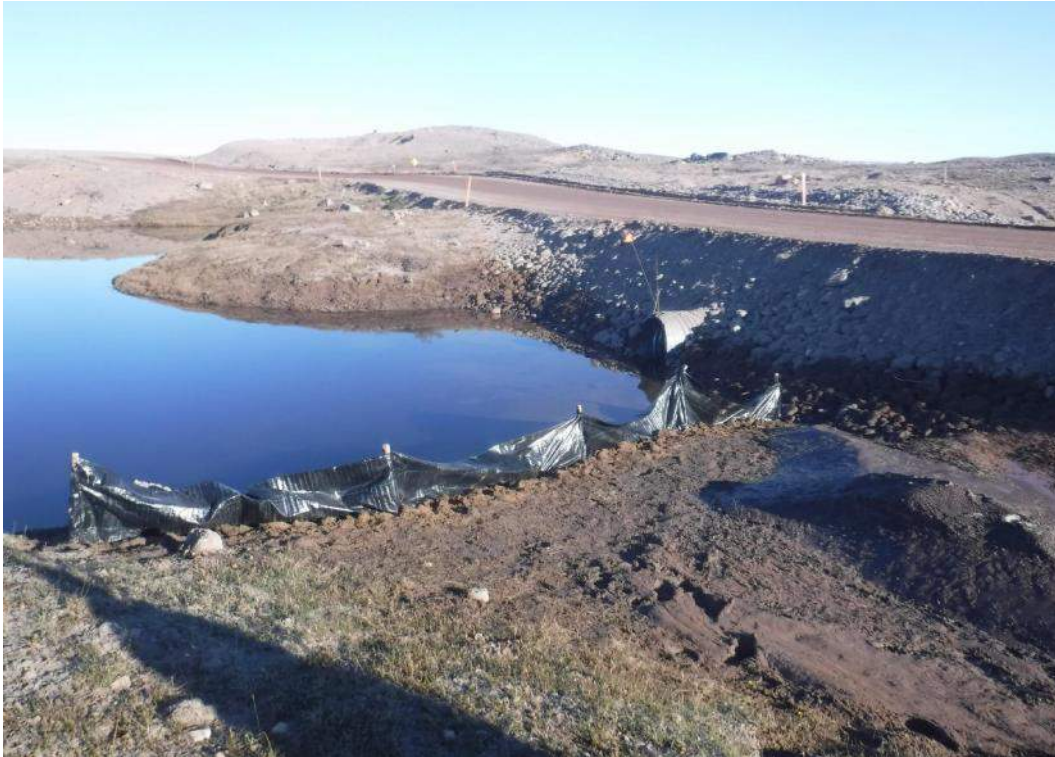
June 26, 2017 - Silt fences installed near BG-30 (upstream)
