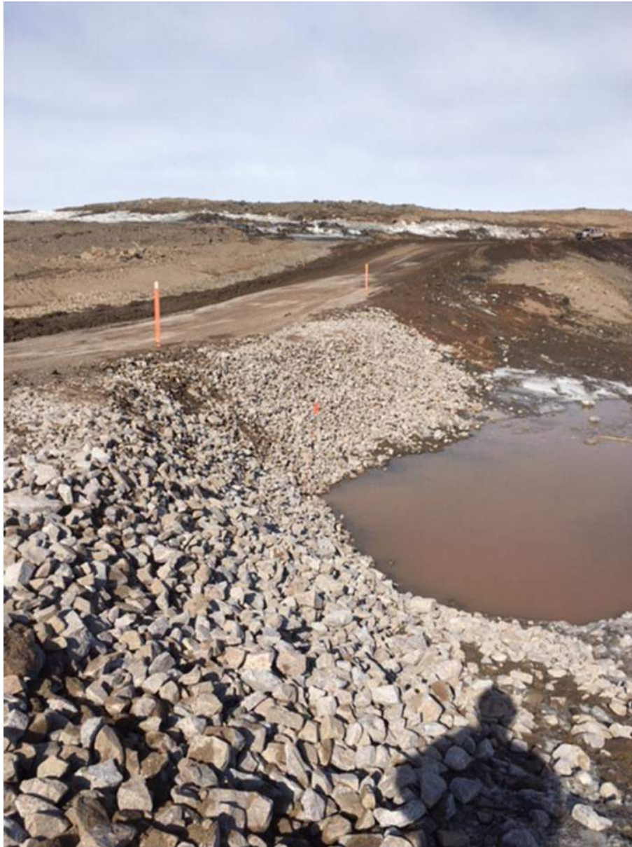
May 30, 2017 – Armouring of road embankments near BG-29
