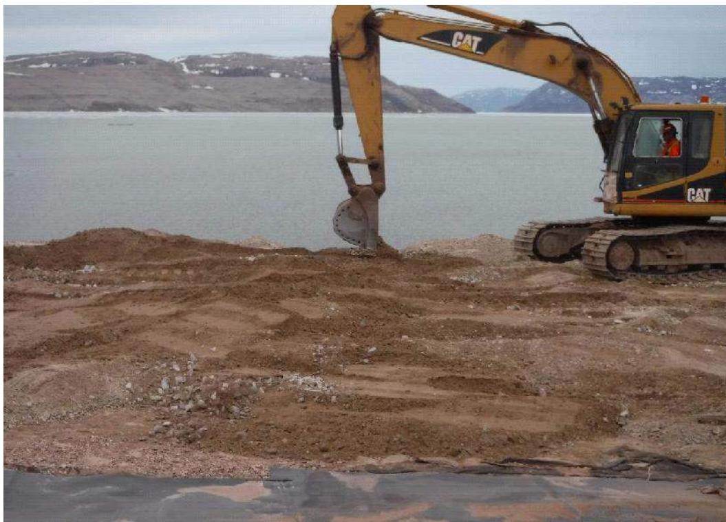
June 29, 2017 – Additional re-grading of locations that experienced erosion during MP-05 overflow
