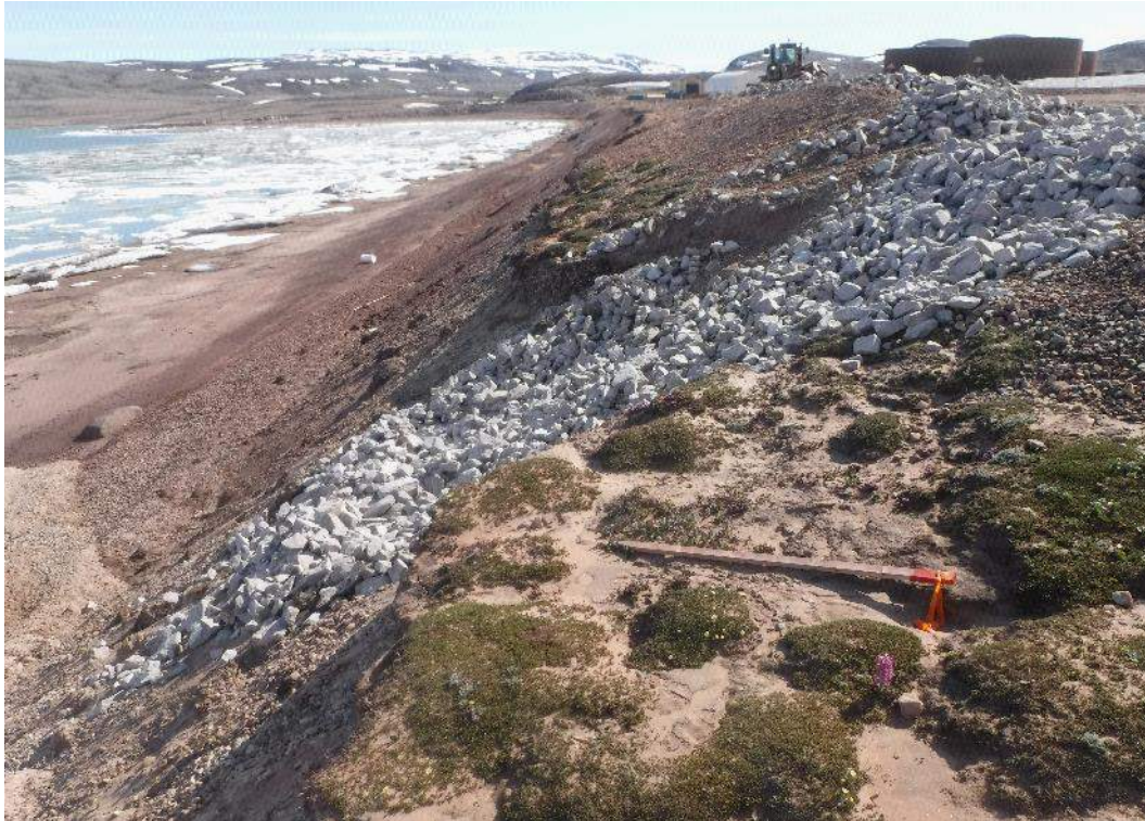
July 1, 2017 - Additional rip-rap placed downstream of MP-05
