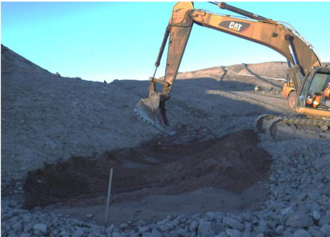
June 23, 2017 – Removing sediment from Camp Lake Sedimentation Ponds
