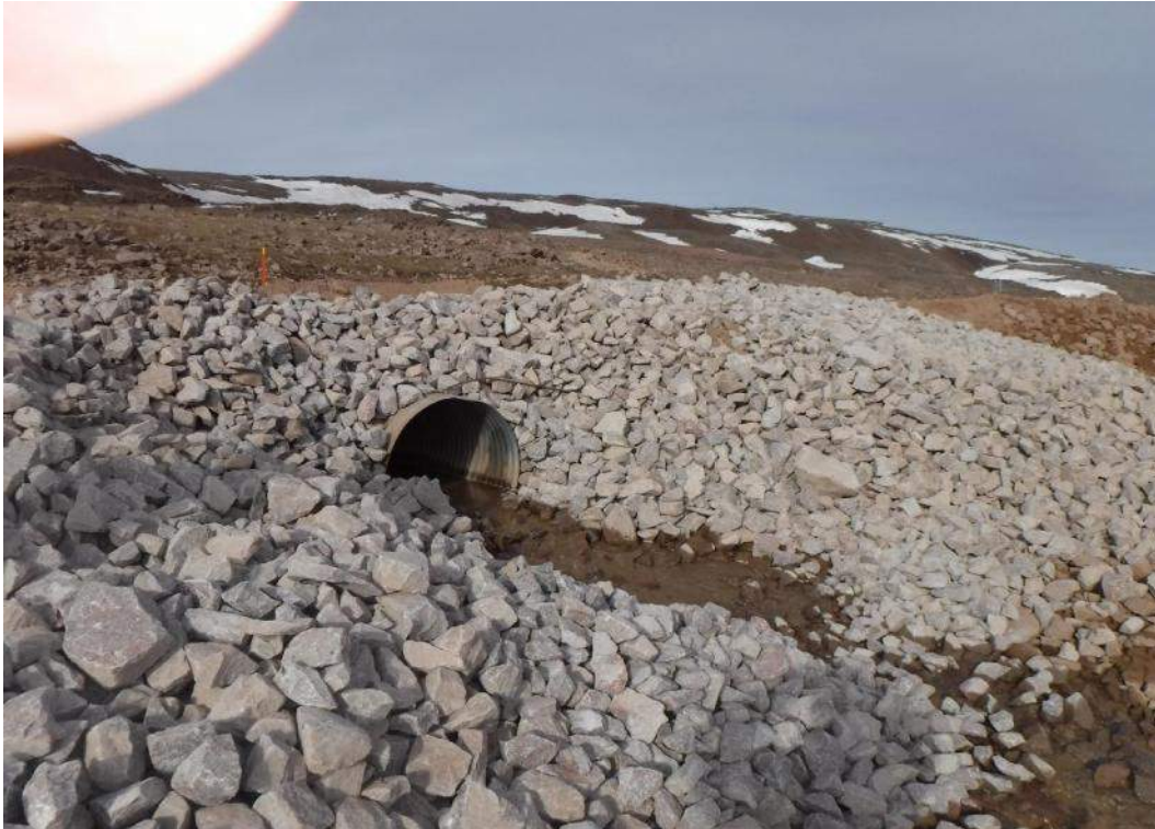
June 10, 2017 – Placement of aggregate (rip rap) near outlet of CV-174
