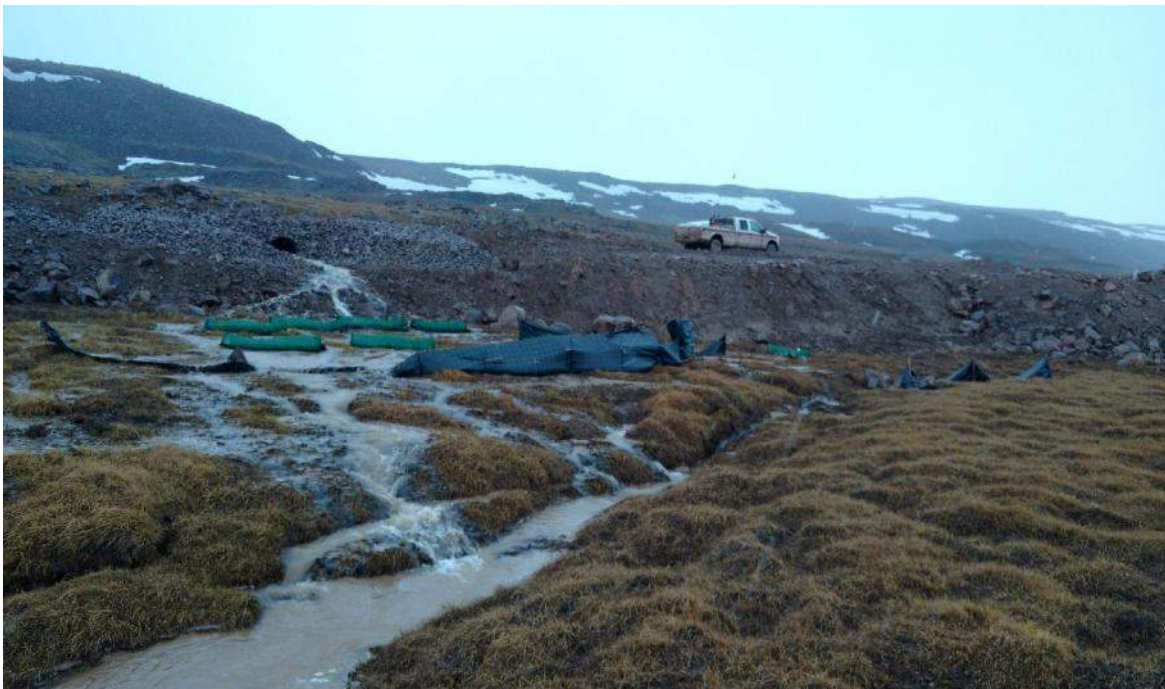
June 15, 2017 - Sedimentation control measures installed at CV-174
