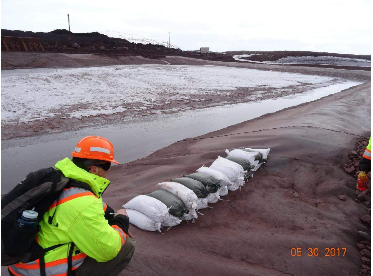
Figure 6: sandbags improperly installed
