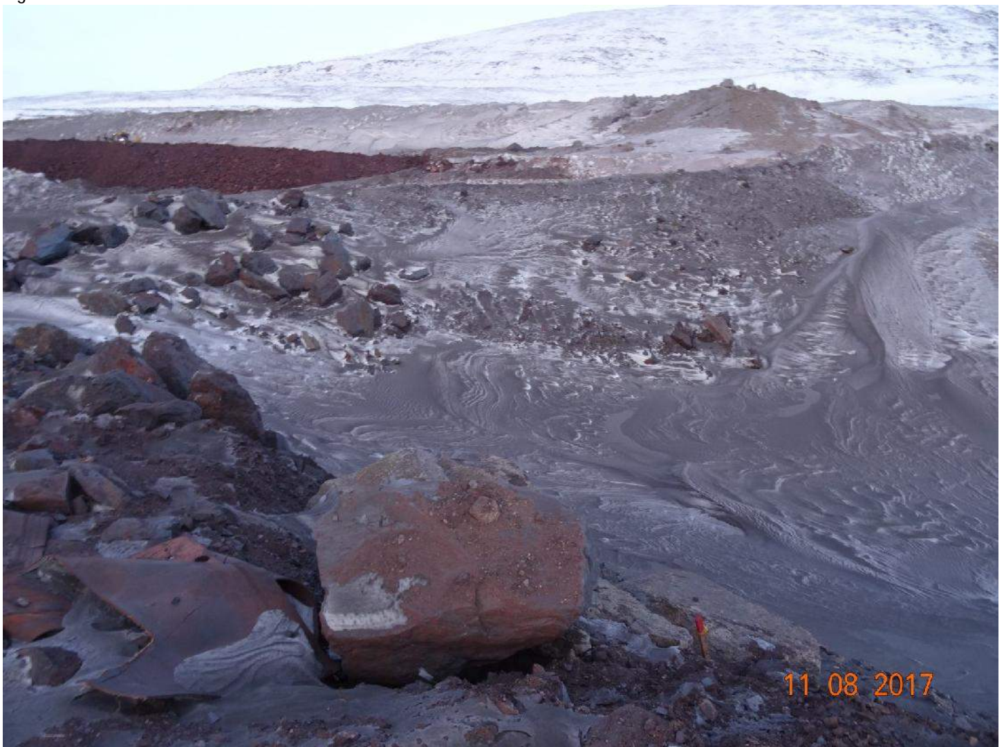
Figure 4: Crusher pad-There is no diversion ditches below this “oversize” ore.
