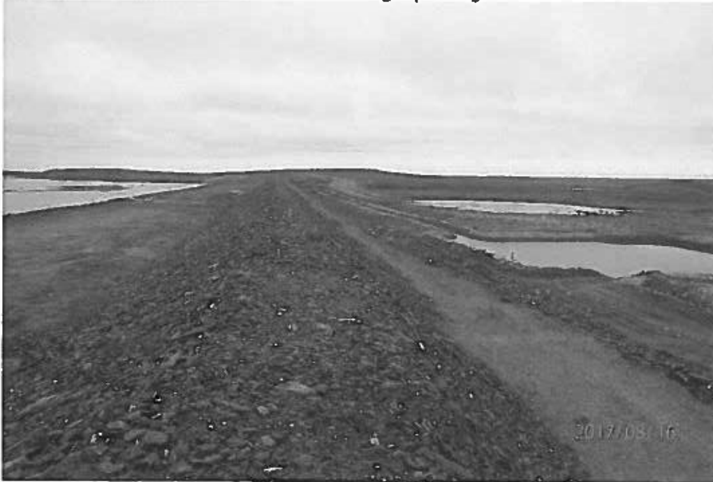
Photo 3: DCP-1, Thermistors indicated core is freezing as per design
