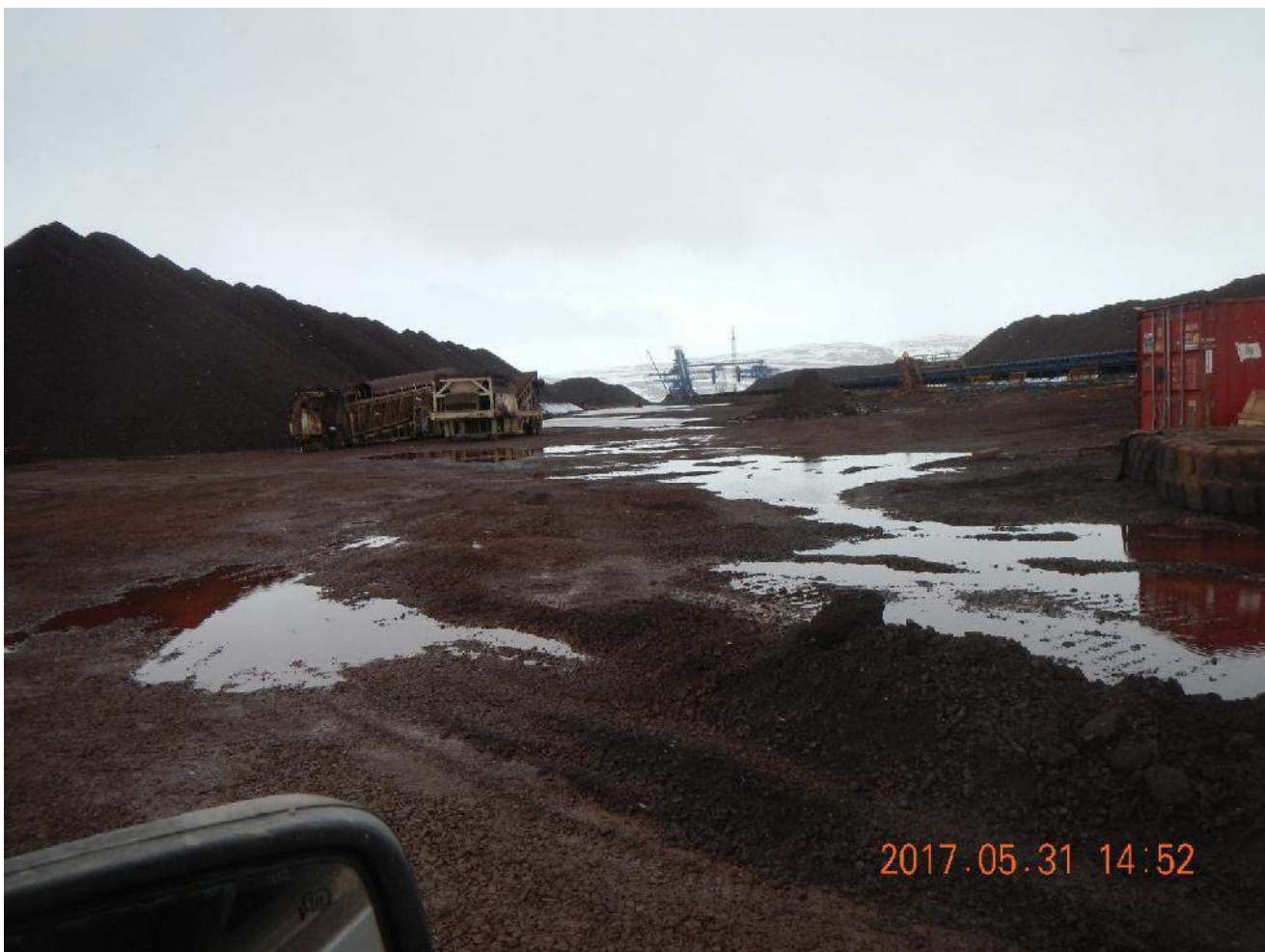
Figure 5: water pooling inside the ore stockpile pad
