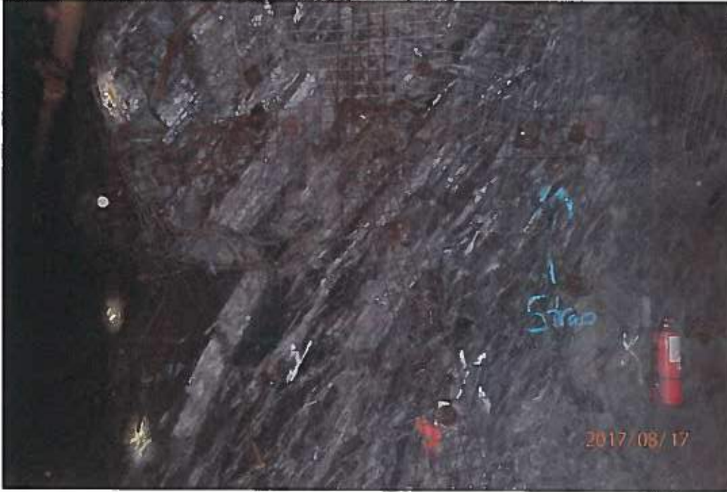
Photo 2. Box cut for Portal 2. Supported as per design. A multi-plate culvert will be socketed into the rock and then backfill placed.
