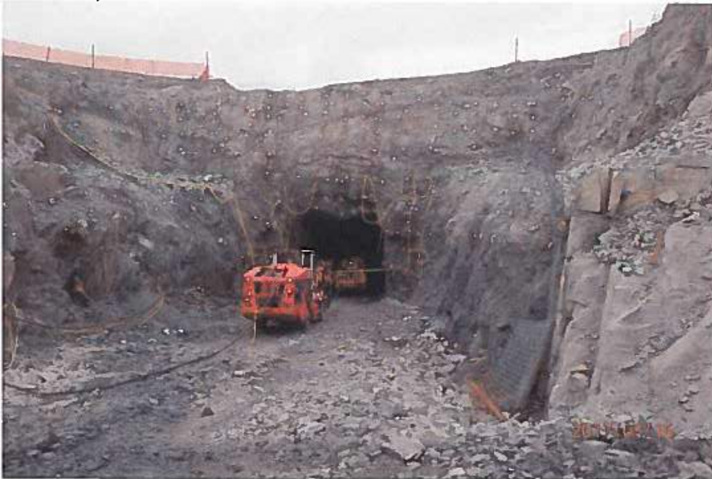
Photo 2. Box cut for Portal 2. Supported as per design. A multi-plate culvert will be socketed into the rock and then backfill placed.
