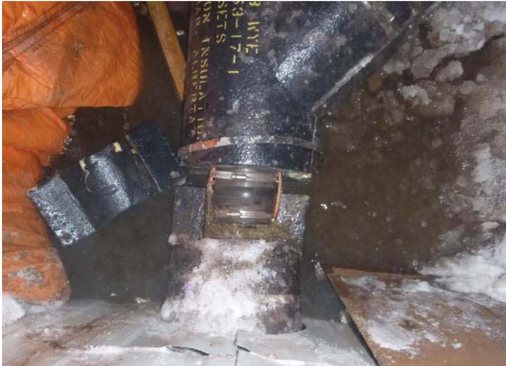
Photo 1: Separated coupling on the gravity line feeding the lift station
