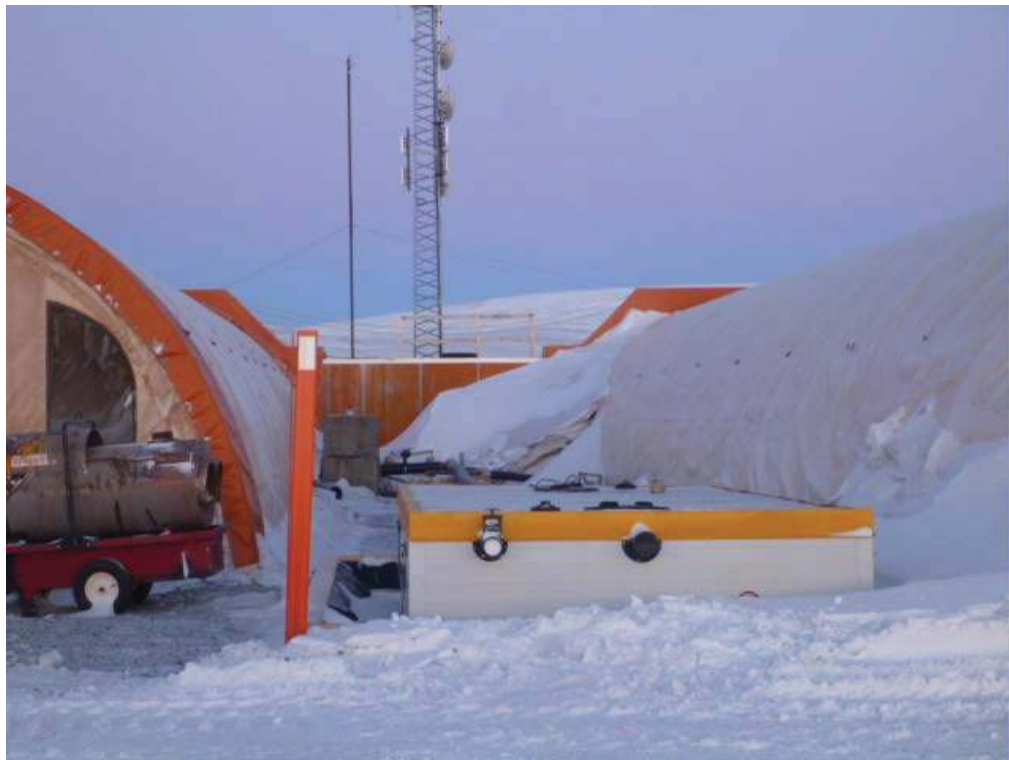
Photo 3 – New Lift Station and Discharge Line
