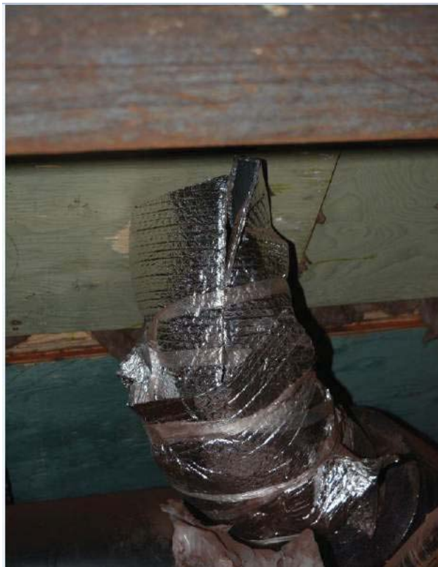
Photo 2 - Repaired elbow on discharge line of industrial washing machines
