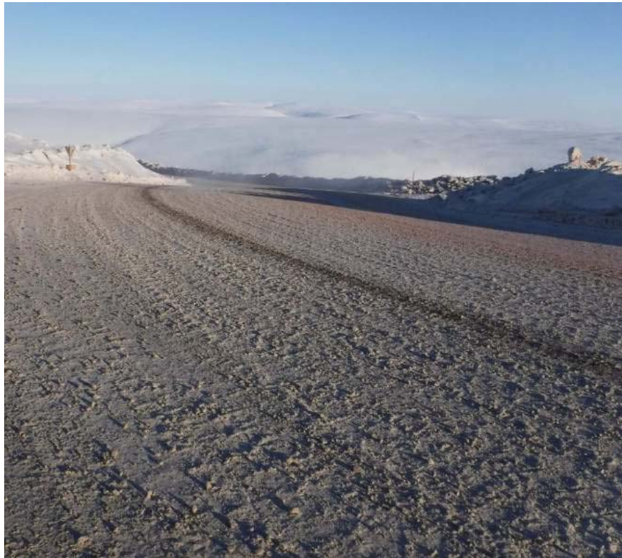
Photo 1 – Trail of coolant 30 cm wide on the Mine Haul Road
