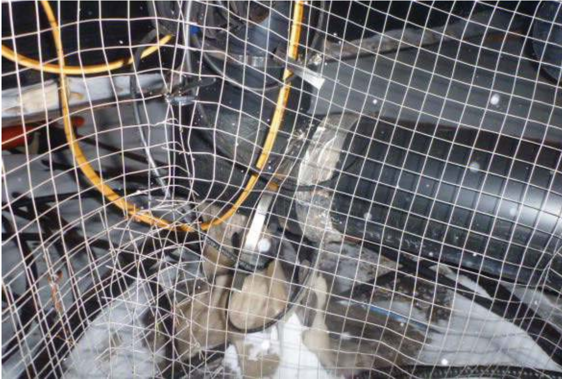
Photo 1 – Discharge line separated at elbow
