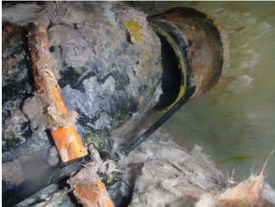
Photo 1 – Separation of elbow on discharge line of industrial washing machines
