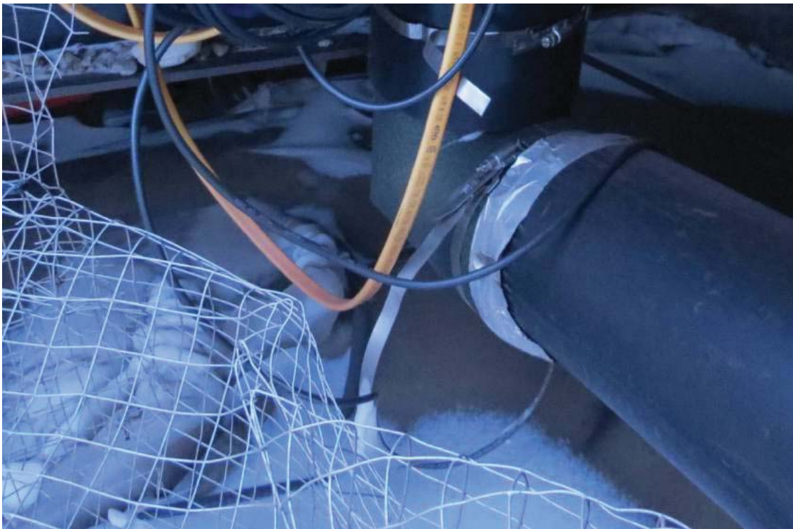
Photo 2 – Discharge Line Elbow Repaired
