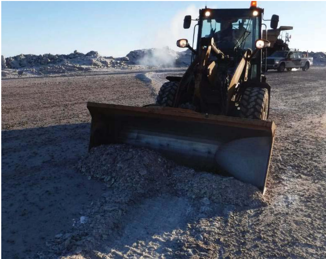
Photo 3 – Contaminated snow being removed from the surface of the Mine Haul Road
