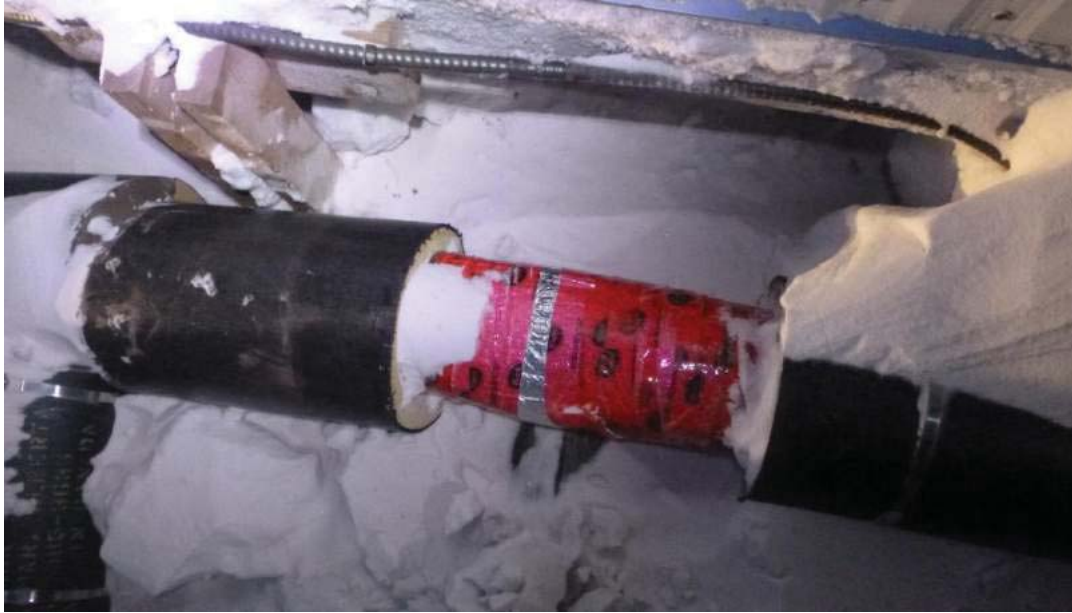
Photo 1 – Repaired and insulated coupling prior to fiberglass insulation being installed.
