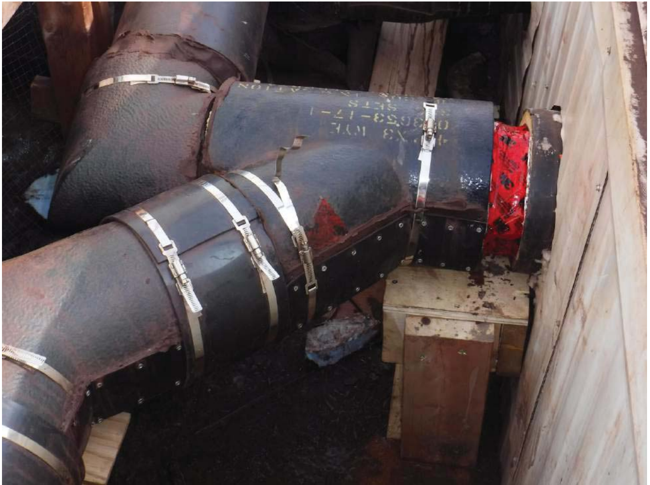
Photo 3 – New coupler and wood support installed on 4" gravity line
