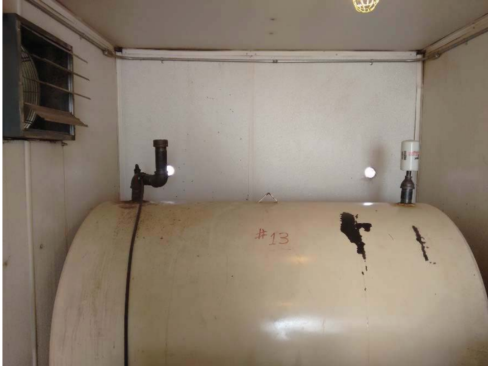
Photo 3 – Tank set up with hose inside secondary containment
