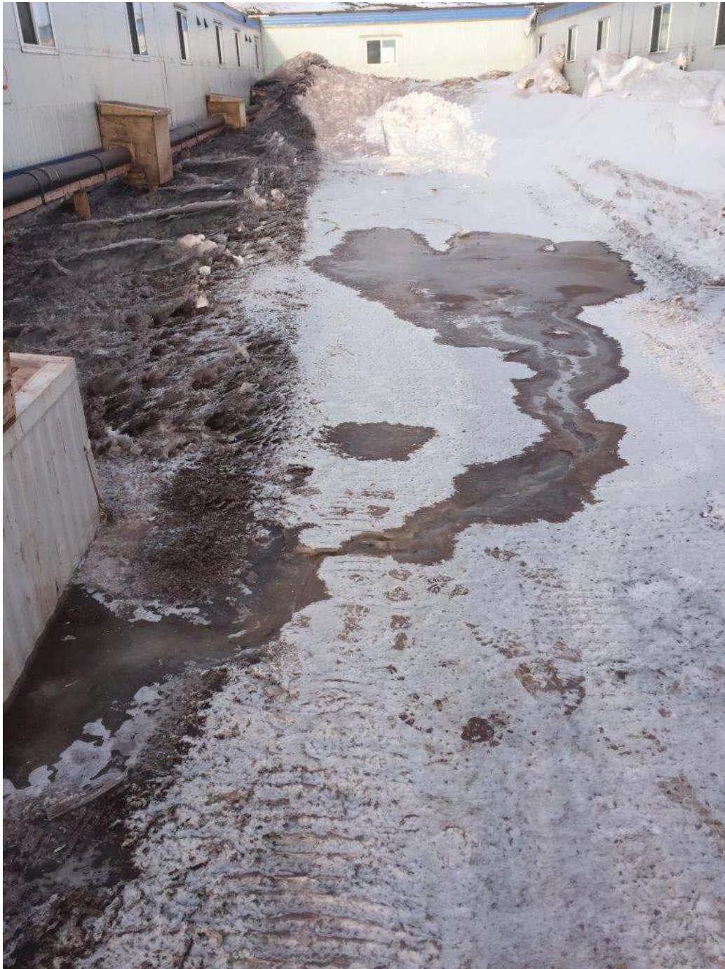
Photo 2 – Raw sewage released to the adjacent ground south of MSC AF Wing
