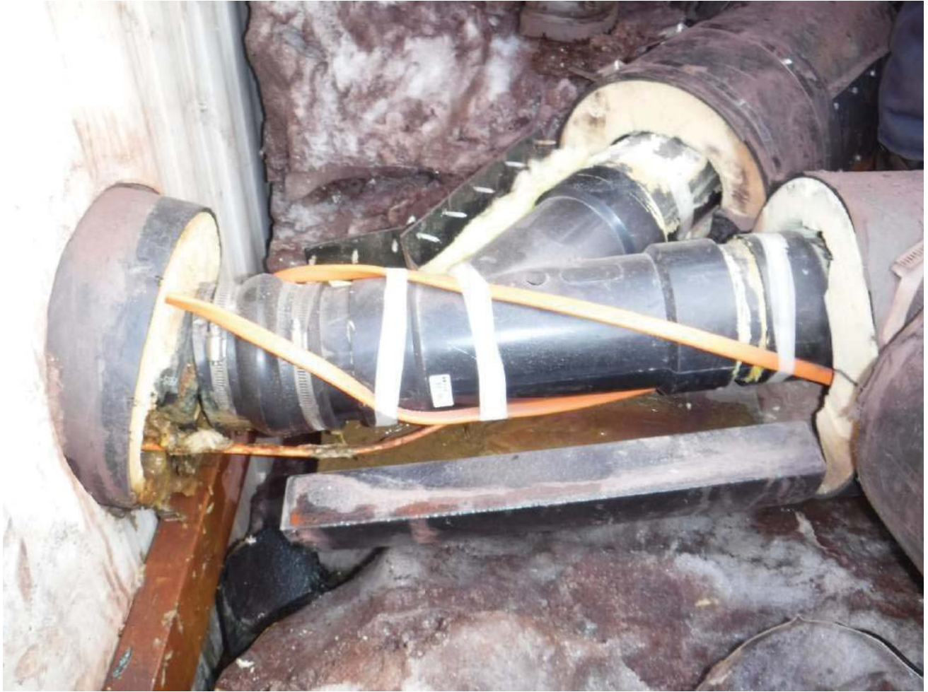
Photo 1 – Fernco coupler separated on the 4" gravity line into the lift station
