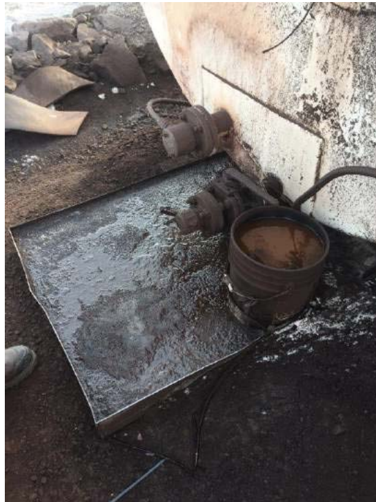
Figure 2 – Leaking Wiggins Nozzle into drip tray that mixed with snow melt overtopping
