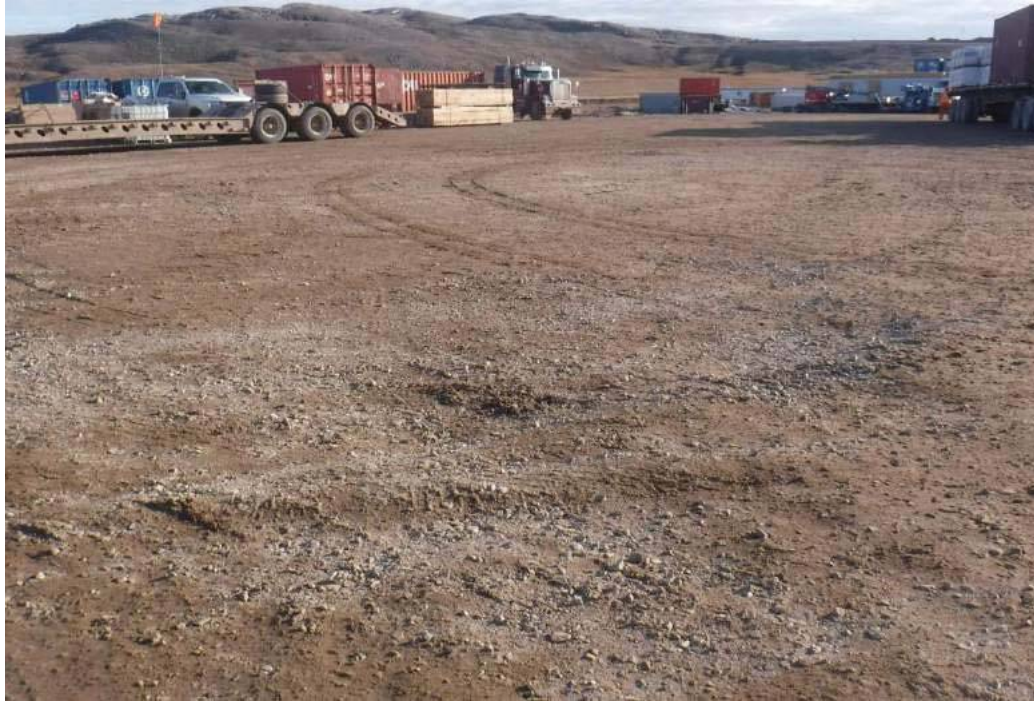
Figure 3: Soil Excavated and clean fill replaced and leveled.
