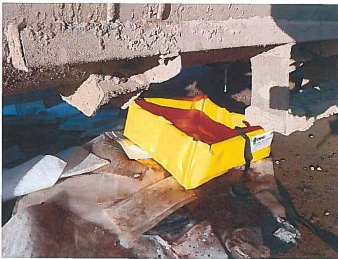
Photo 1: Plugged fuel leak and berm to contain fuel.
