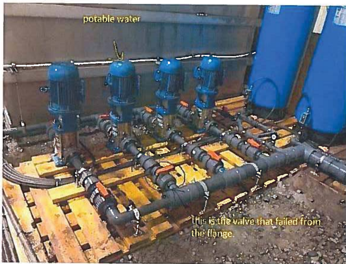
Photo 1: Distribution pumps with broken valve on #2 that released the water.
