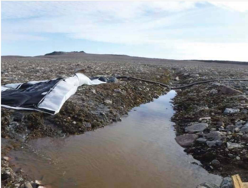
Photo 1: Geotube filtration system downstream of the FDP on the discharge line installed to mitigate TSS exceedances
