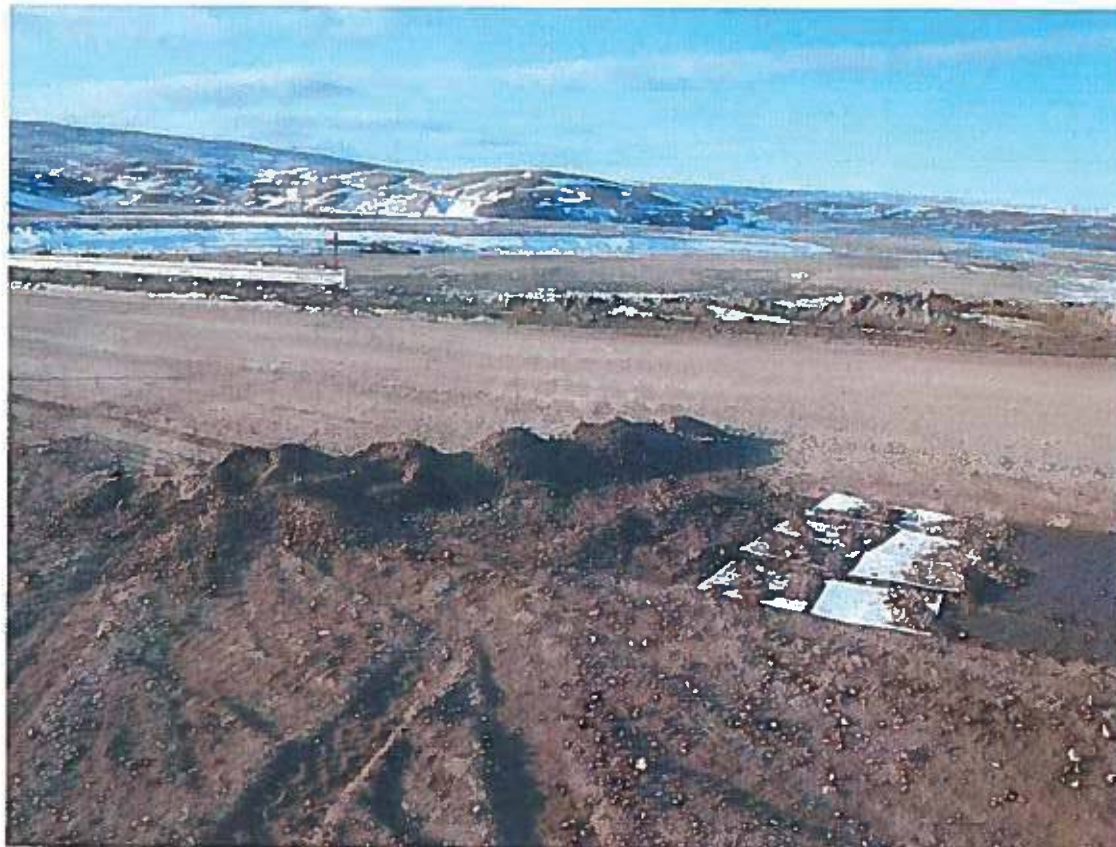
Photo 2: Contained Fuel Spill with Absorbent Pads
