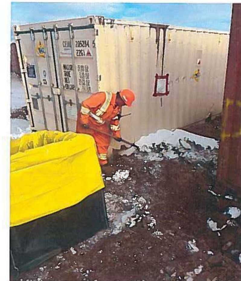
Photo 2: Ammonium Nitrate and contaminated soil being removed and placed into Quatrex bags
