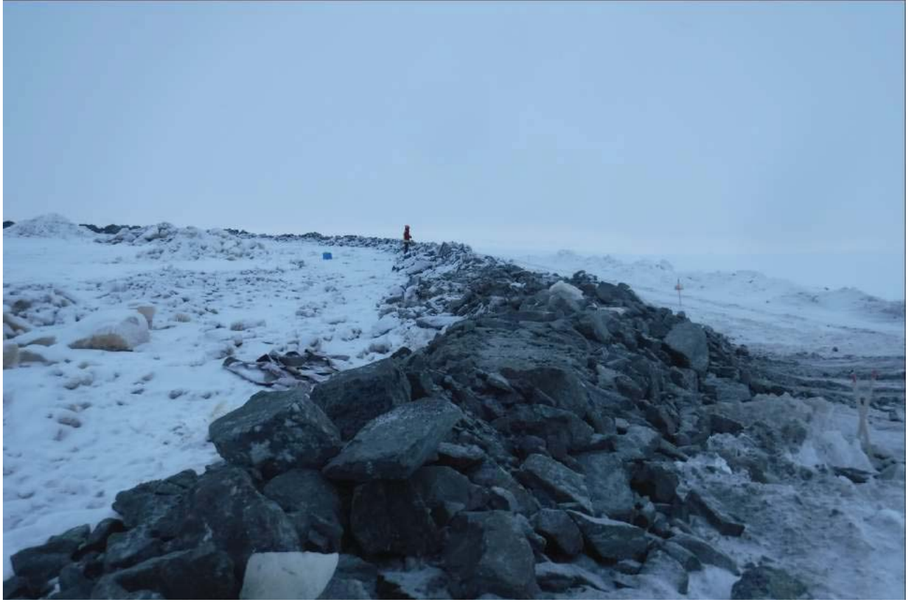
Photo 2: New Berm Being Constructed beside Existing Emergency Ditch
