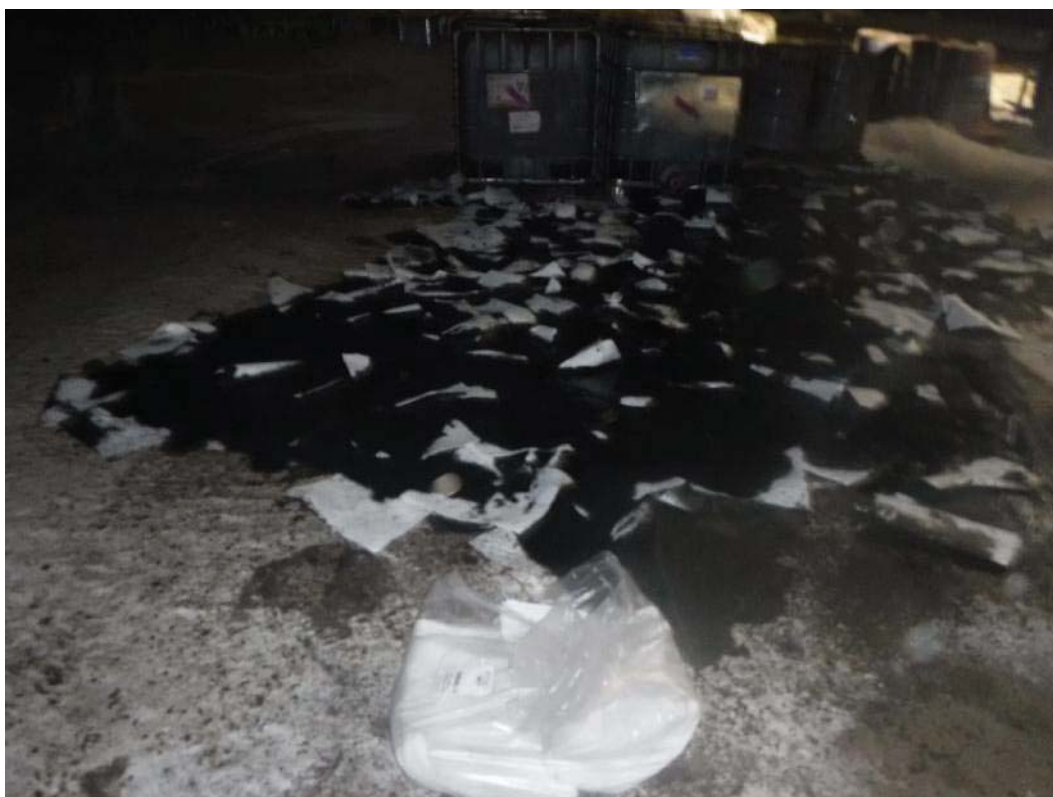
Photo 2. Absorbent booms and pads to prevent migration of the used oil
