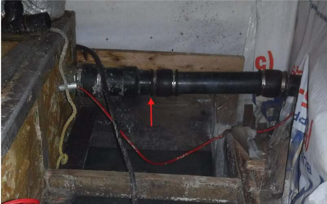
Photo 1. Repaired coupling at lift station.
