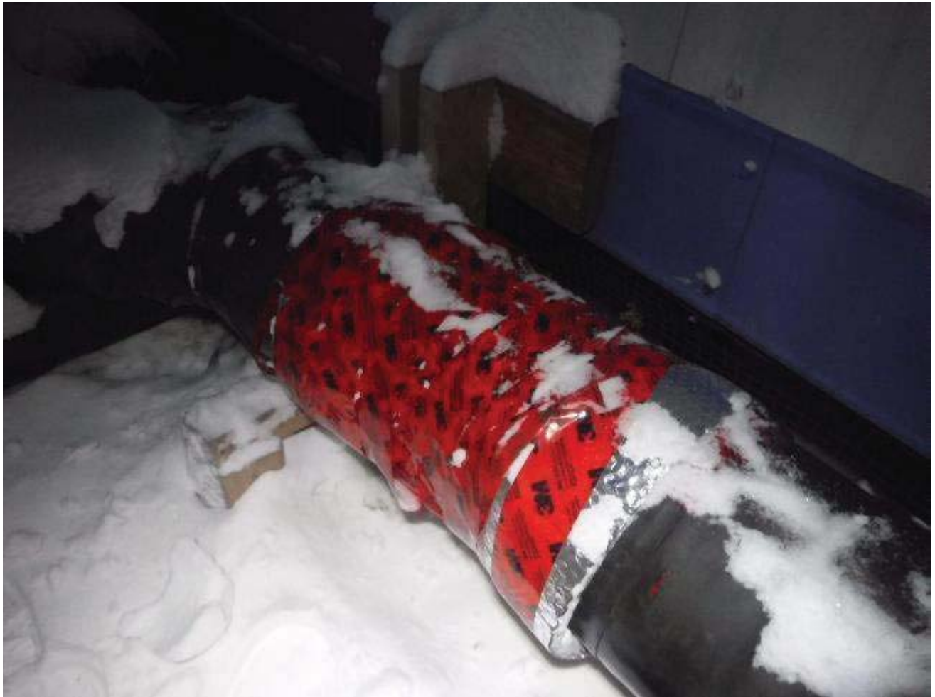
Photo 2 – New coupler and wood support installed on 4” gravity line
