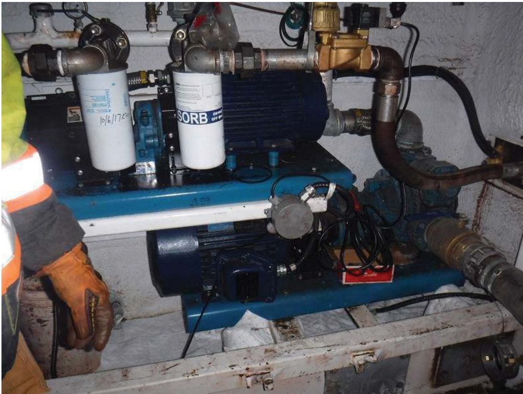
Photo 2. Fuel pump, switch, and valve
