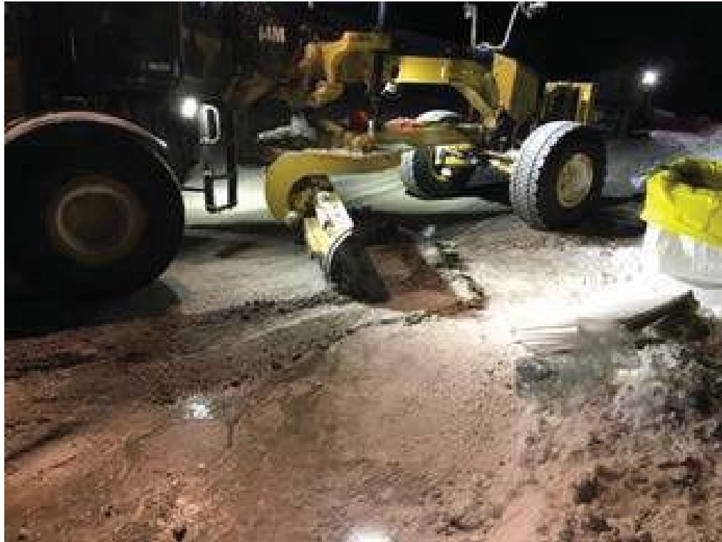
Photo 3: Grader removing contaminated snow for placement into Quatrex Bags
