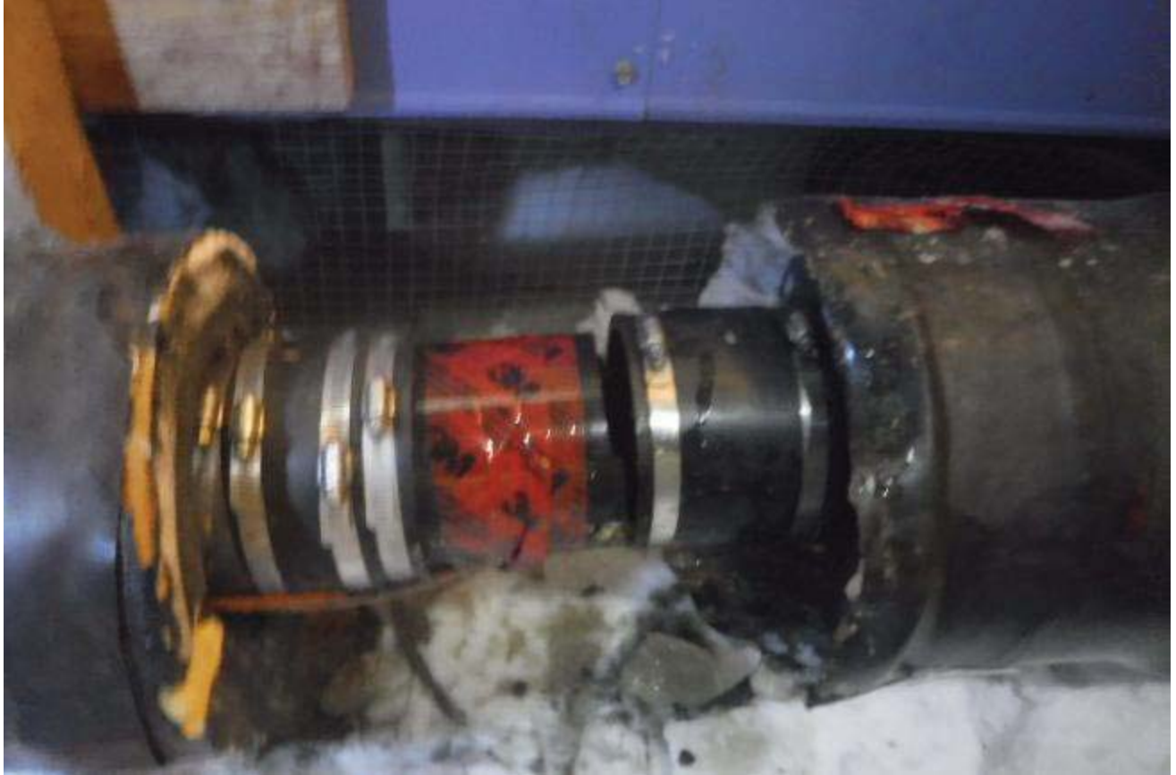
Photo 1 – Fernco coupler separated on the 4" gravity line into the lift station
