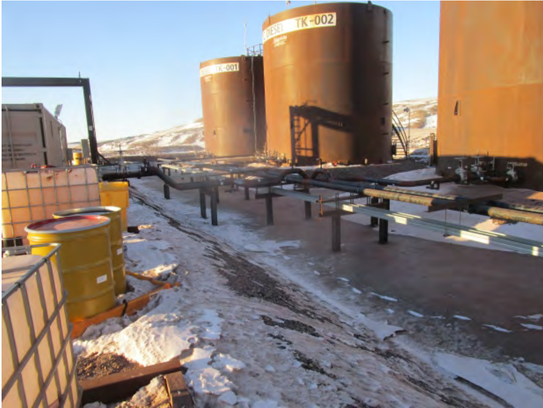
M. Mine Site Fuel Tank Farm Containment
