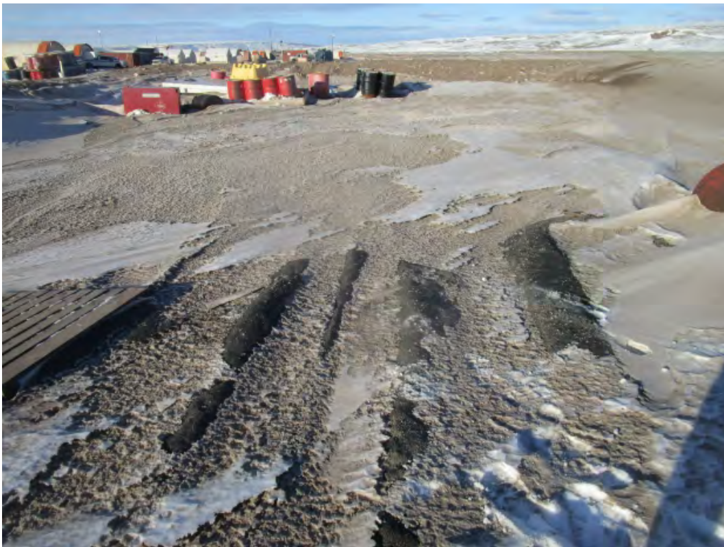
H. MS-HWB-2 – Hazardous Waste Storage – Exposed Liner
