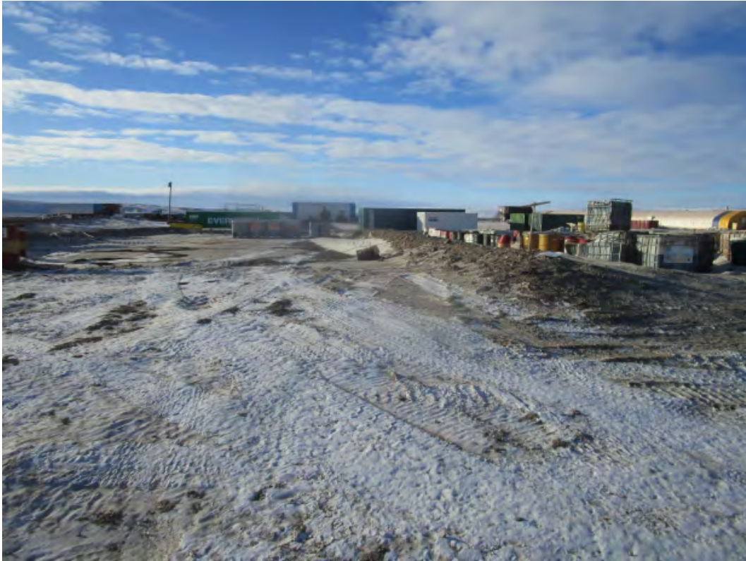
G. MS-HWB-3 – Barrel Fuel Containment
