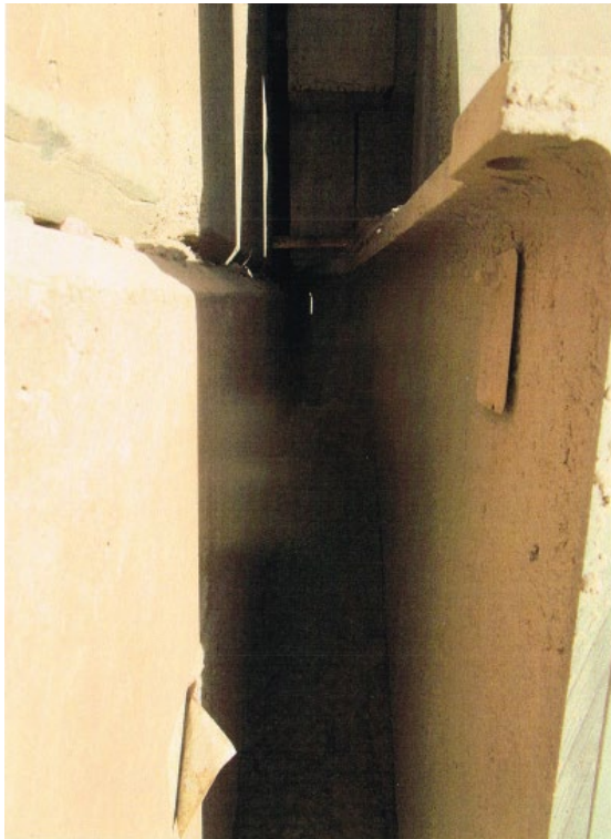
Photo 2 - North Abutment - NW Corner
