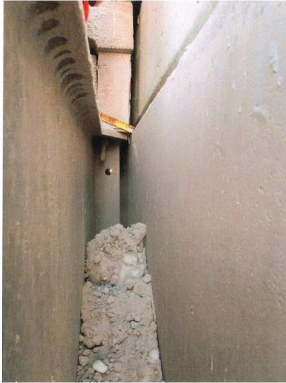
Photo 1 - North Abutment - NE Corner
