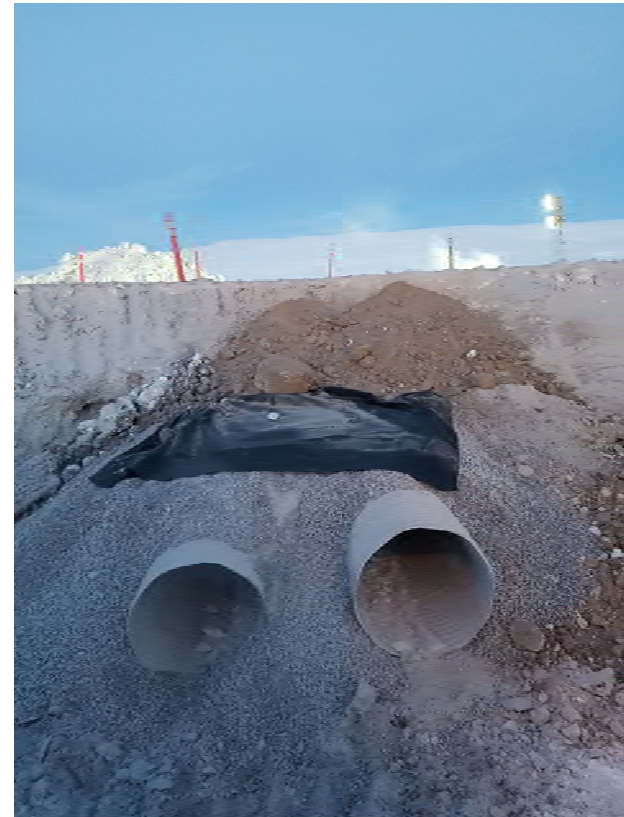
Figure 8. CV224 construction activities
