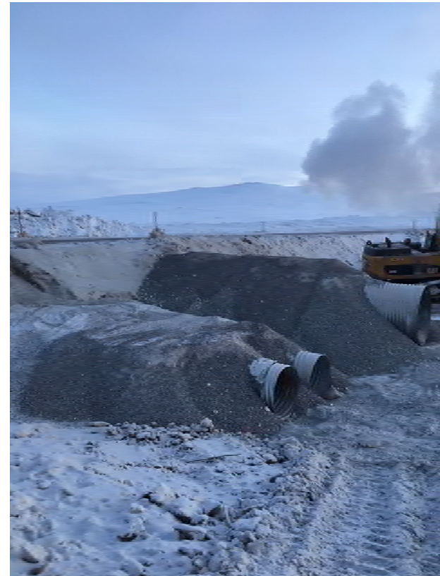
Figure 8. BG04 construction activities
