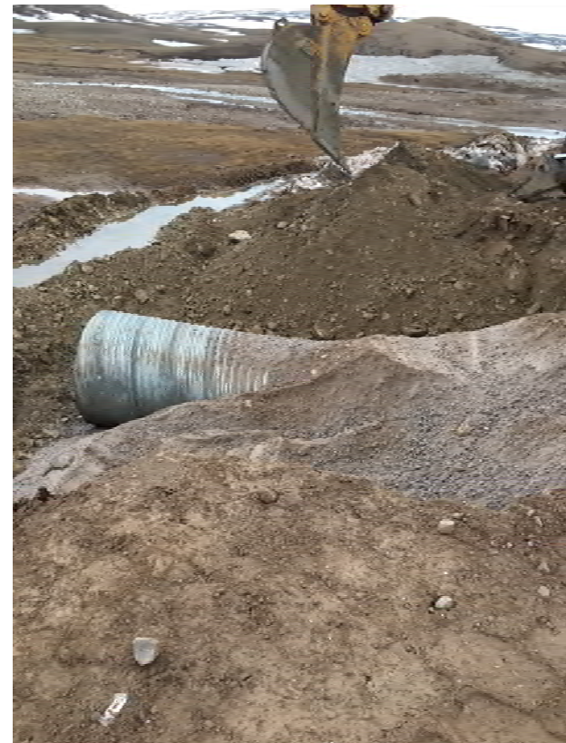
Figure 2. CV079 construction activities
