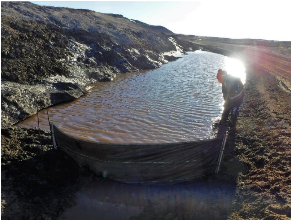
PHOTO 4 – Sediment control measures at culvert BG-27 – June 2018
