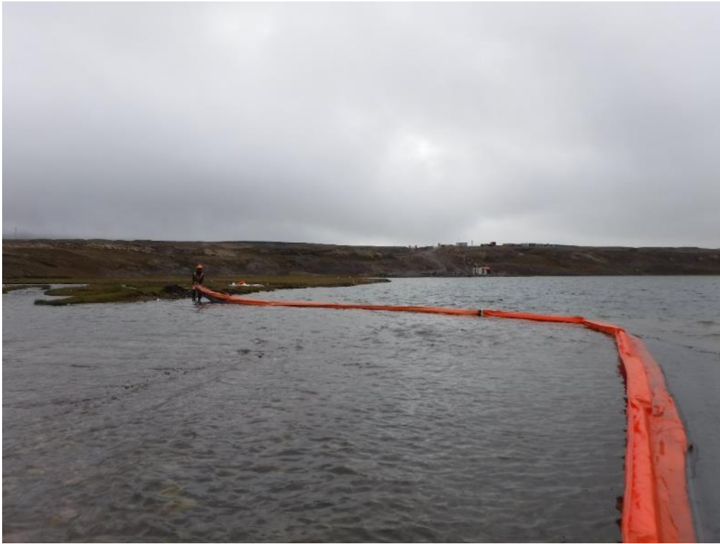
PHOTO 21 – Camp Lake Tributary silt curtain installation –June 2018
