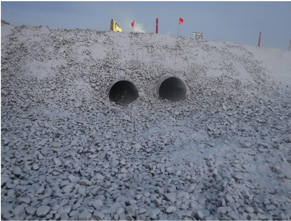
PHOTO 3 – Culvert CV-244 replacement – January 2018
