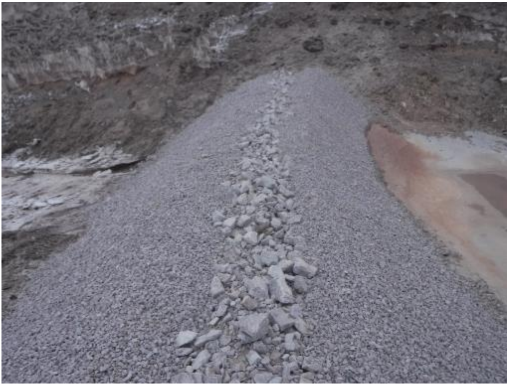
PHOTO 15 – Camp Lake drainage channel check dam – May 2018
