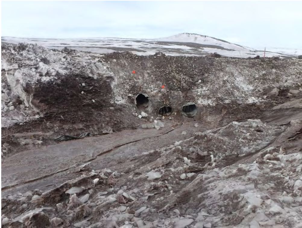
May 13, 2018: BG-01-DS Road Crossing Upstream of CLT-OUT After Snow Removal
