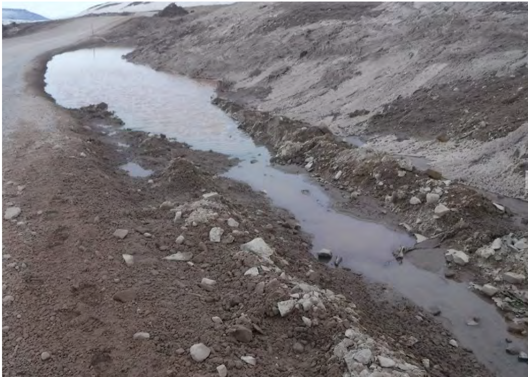
May 30, 2018: Upstream View of BG27 Looking Downstream
