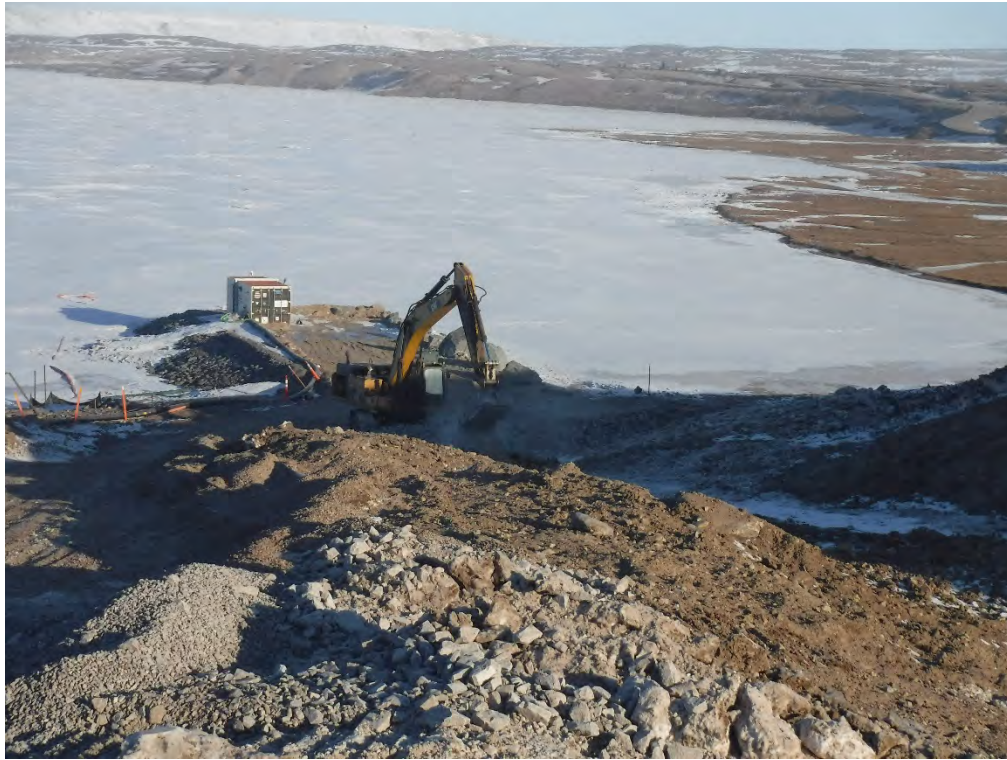
May 21, 2018: Berm Expansion of Camp Lake Settling Ponds During Construction Upgrades
