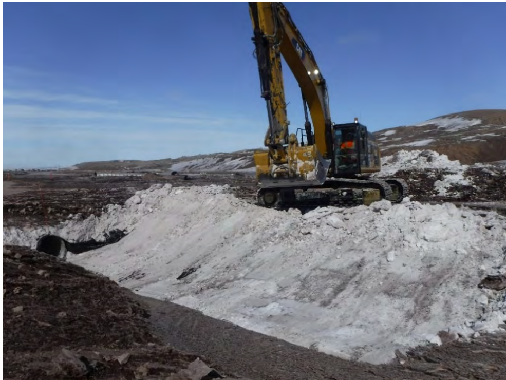
May 9, 2018: CV-186-US Road Crossing Upstream of SDLT-OUT After Snow Removal
