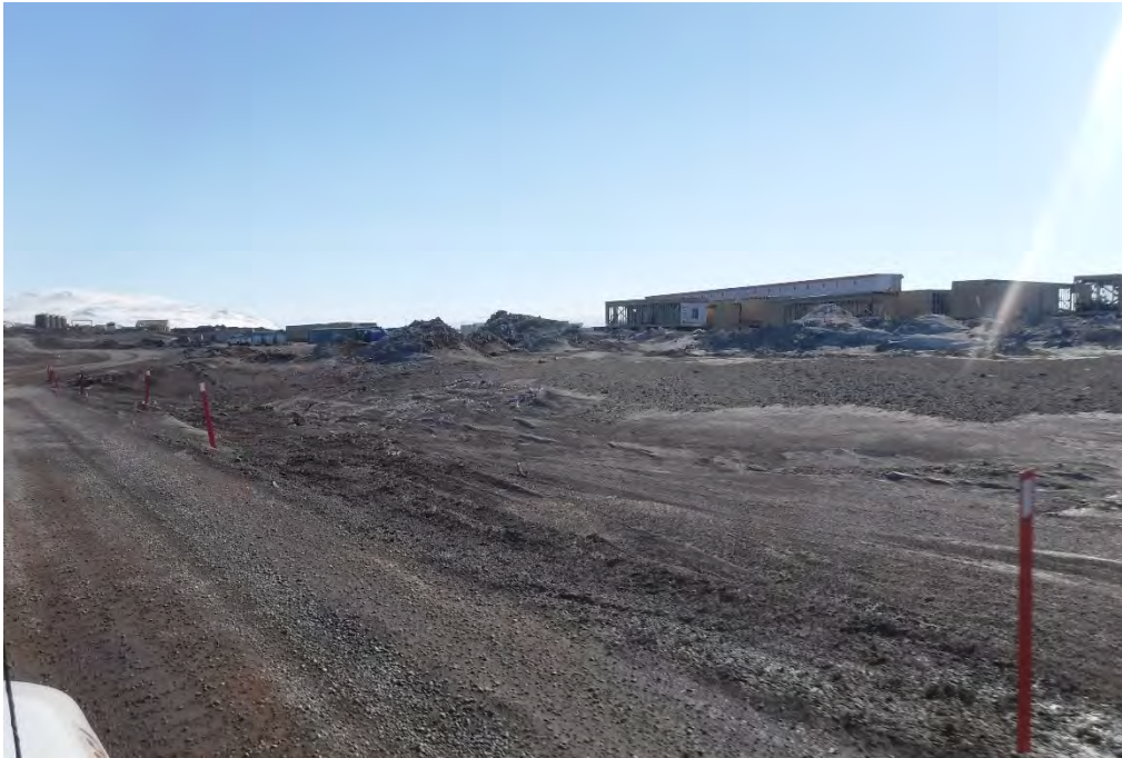
May 8, 2018: CV-186-DS Road Crossing Upstream of SDLT-OUT Before Snow Removal
