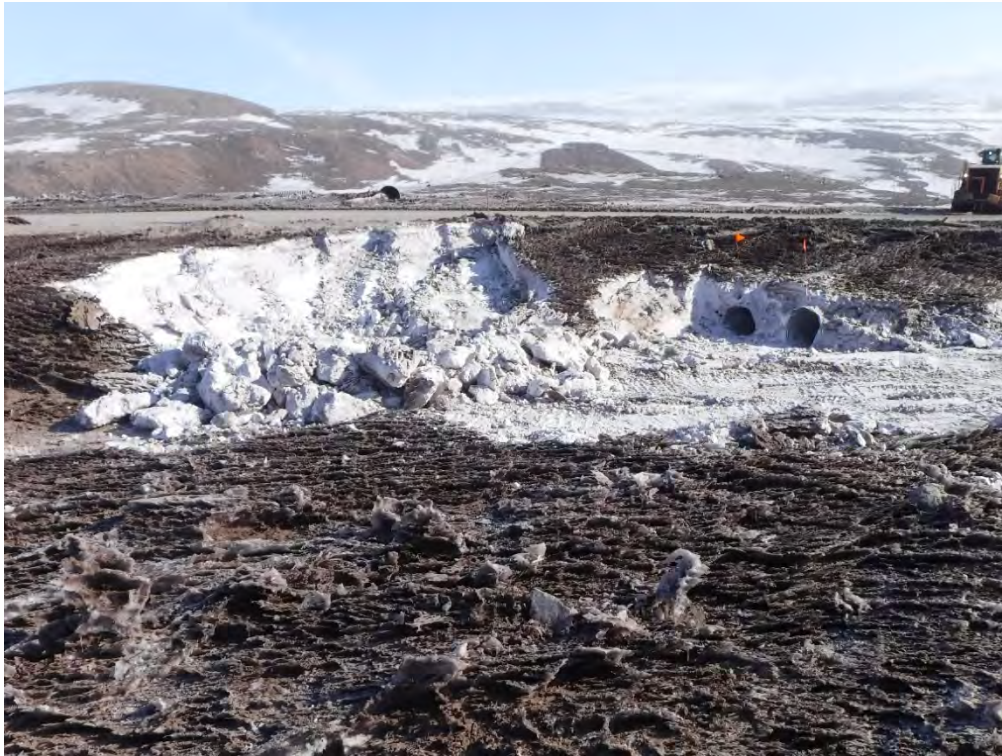
May 9, 2018: CV-186-DS Road Crossing Upstream of SDLT-OUT After Snow Removal
