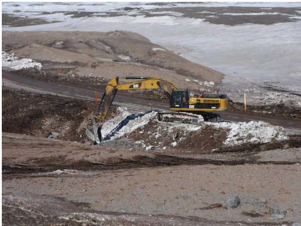
May 13, 2018: BG-01-DS Road Crossing Upstream of CLT-OUT During Snow Removal
