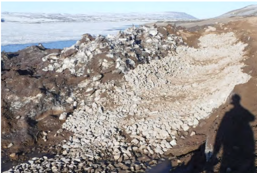
June 6, 2018: Bank Armoring with Riprap Downstream of Crossing
