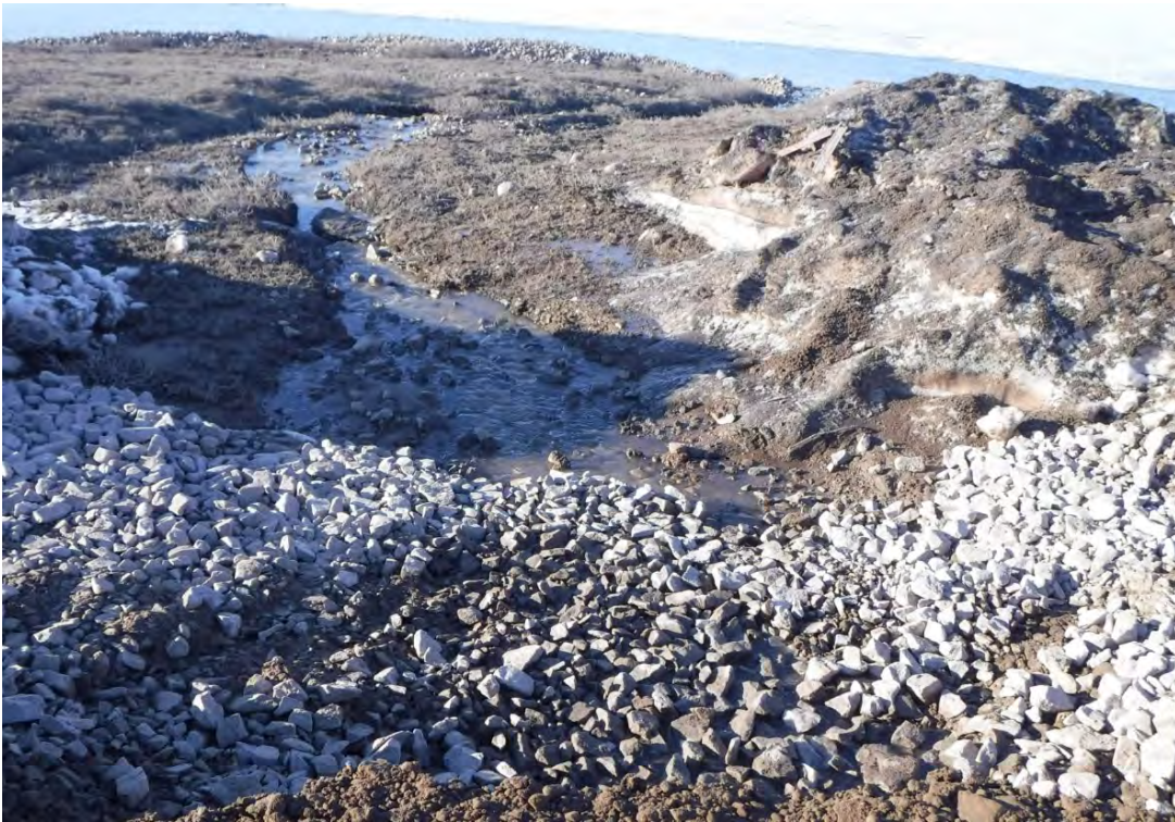
June 6, 2018: Bank Armoring with Riprap Downstream of Crossing
