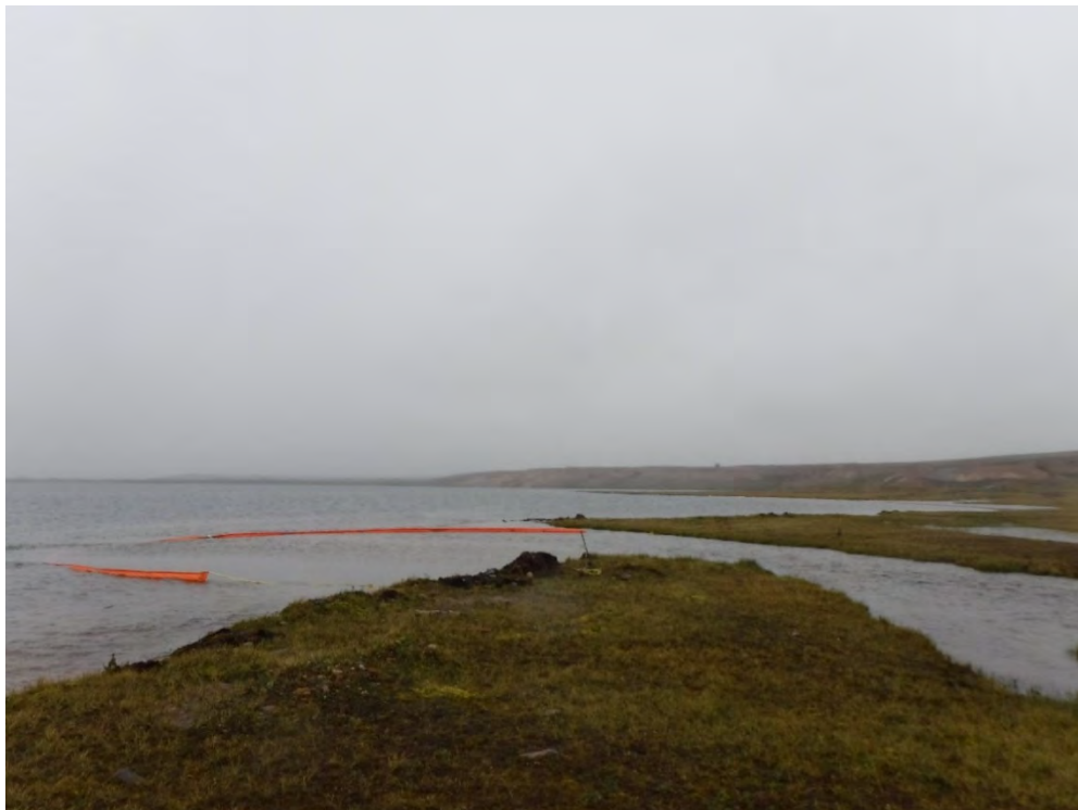
August 7, 2018: Silt Curtain Installation at CLT-OUT
