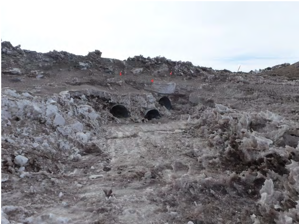
May 13, 2018: BG-01-US Road Crossing Upstream of CLT-OUT After Snow Removal
