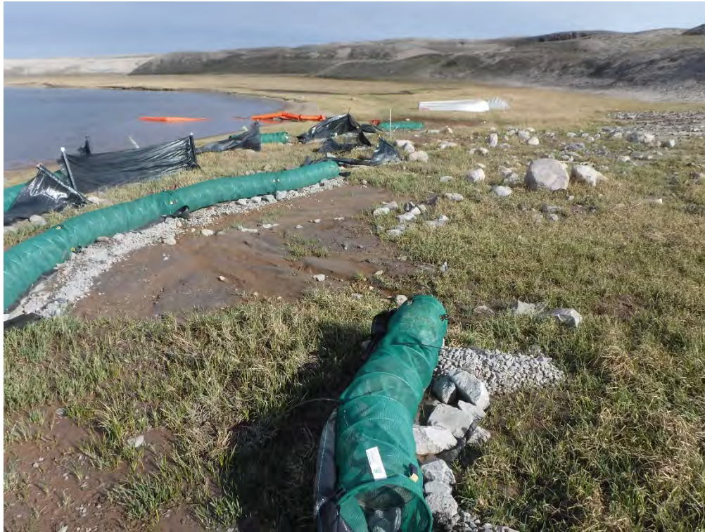
June 23, 2018: Downstream view of CLSP-OUT
