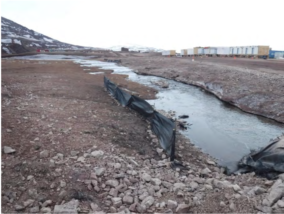
June 2, 2018: Silt Fence Installation at Road Crossing Upstream of SDLT-OUT
