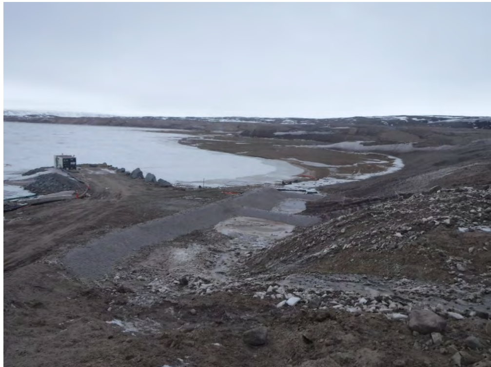
May 22, 2018: Camp Lake Settling Ponds After Construction Upgrades
