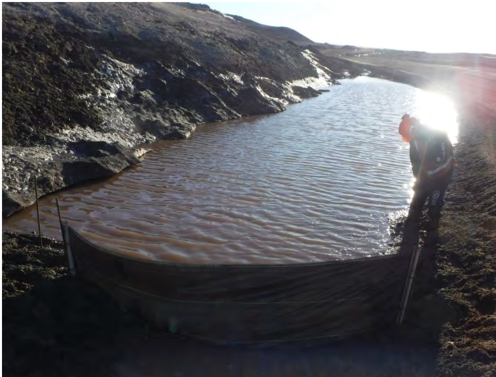
June 6, 2018: Silt Fence Installation Upstream of Crossing
