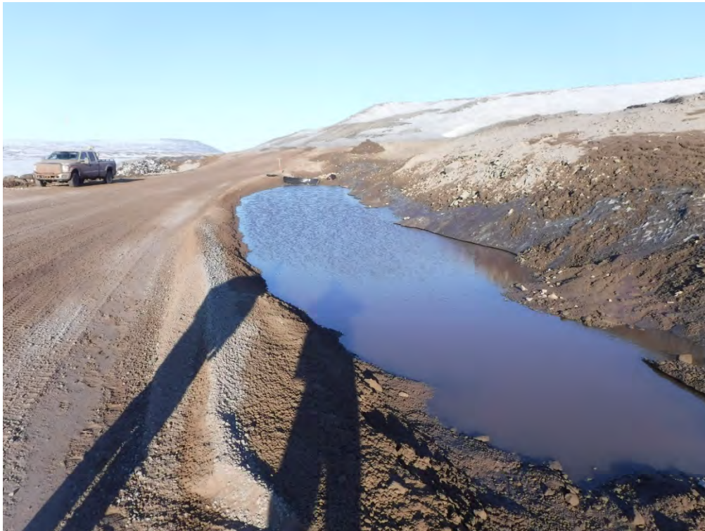
June 6, 2018: Upstream View of BG27 Looking Downstream After Silt Fence Installation
