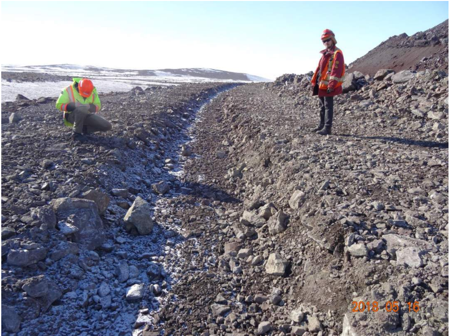
Figure 1: Ditch surrounding Ore Stockpile
