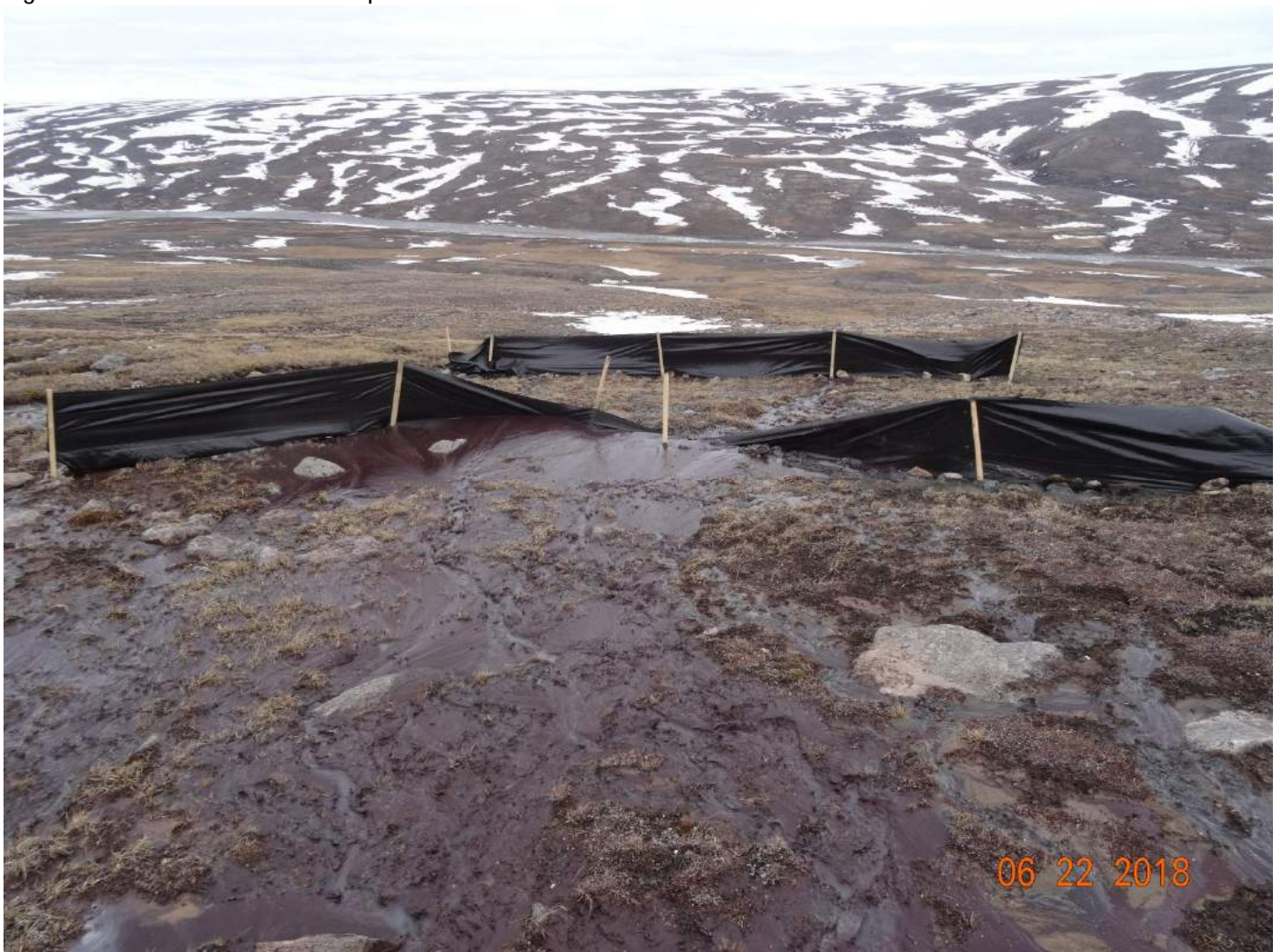
Figure 13: Lack of a sump as required in the licence.
