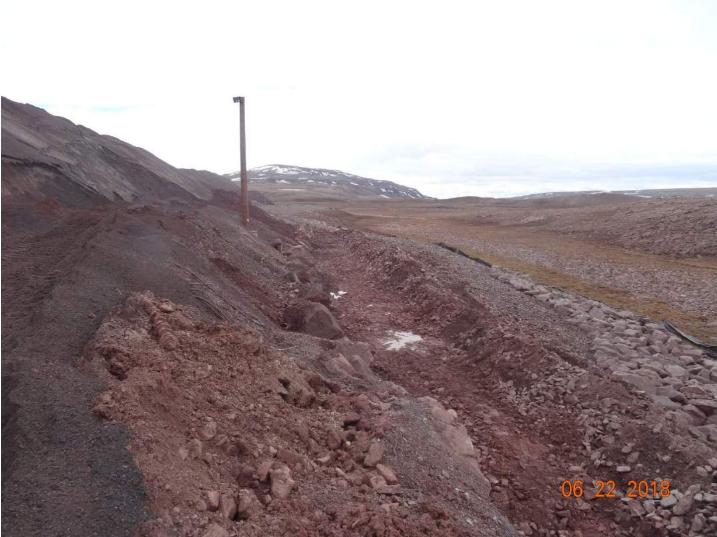
Figure 1: Inconsistent ditch height, land of 8m between ditch and stockpile, ditch inconsistent with approved drawings.
