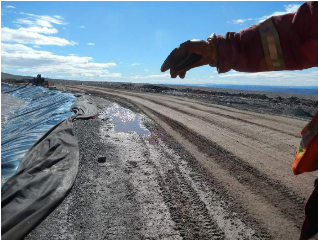
Photo 3: WRF Pond - Berm settlement, geotextile exposed & water ponding btw. 0+040 & 0+060
