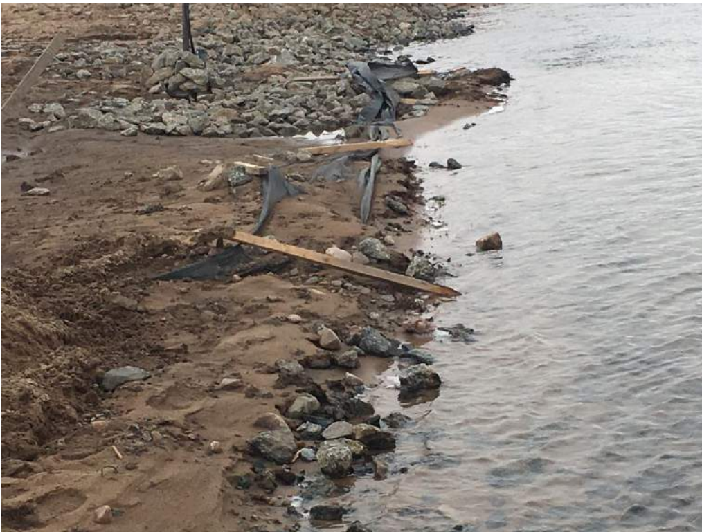
Phot0 10: Southside Downstream of km 80 Bridge – Broken silt fence, sediments went over
