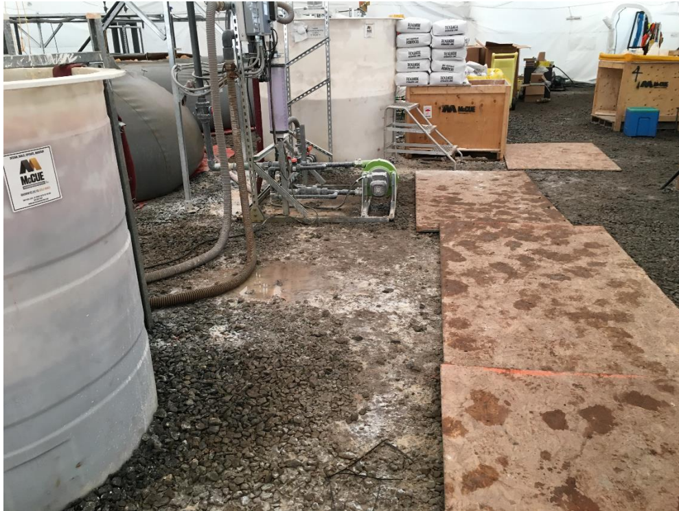
Photo 1: Water treatment plant pad floor – white substance is hydrated lime
