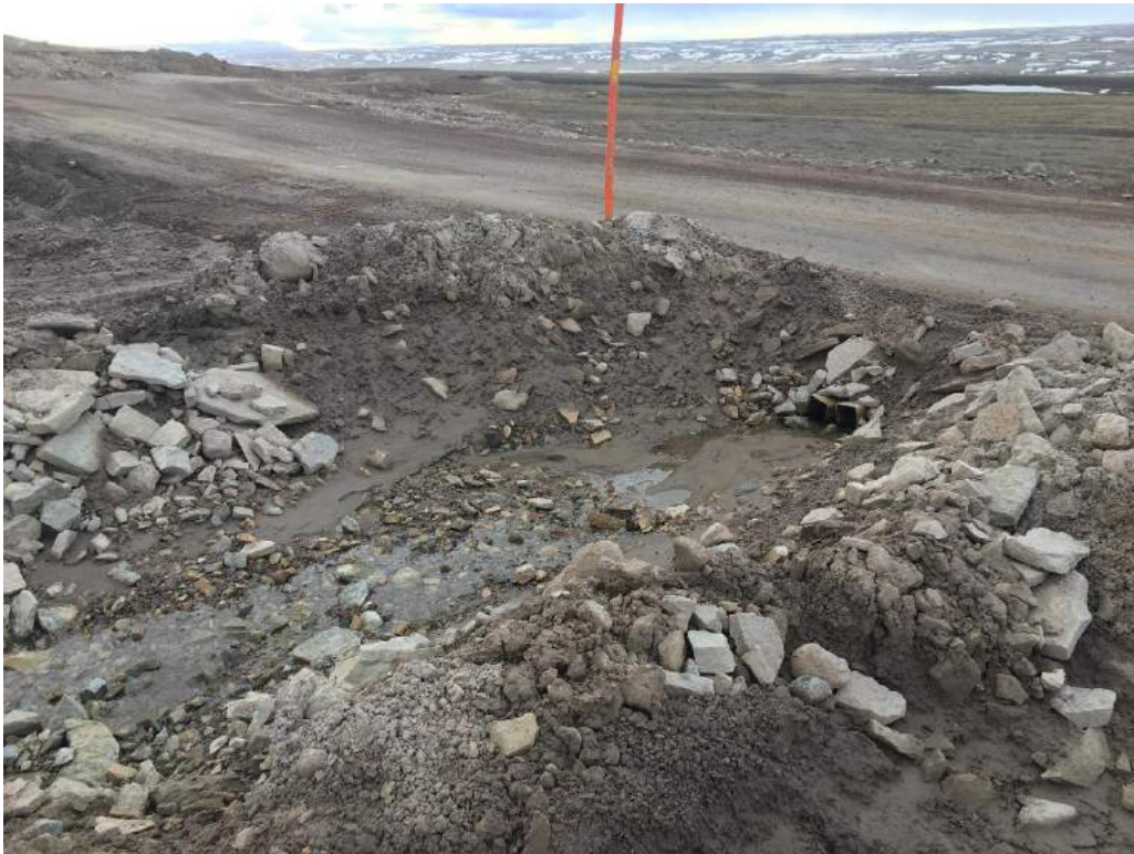
Photo 11: Tote Road Km 74 – Pipes installed in place of damaged culvert
