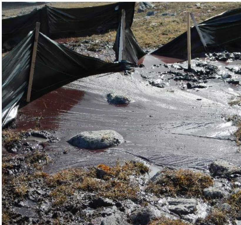
Photo 2: Exploration Drill Location MR3-18-240 – Overloaded and broken silt fence
