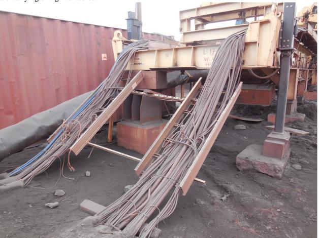
CEC Subrule 12-2200 (5) states, "Cable trays shall be adequately supported by non-combustible supports". CEC Subrule 12-2208 (1) states, "Except as provided for in Subrules (2) and (3), metal cable tray shall be bonded at intervals not exceeding 15 m and the size of bonding conductors shall be based on the ampacity of the largest ungrounded conductor as specified in Rule 10-814 in the circuits carried by the cable tray. Provide support for and bond the cable tray.
