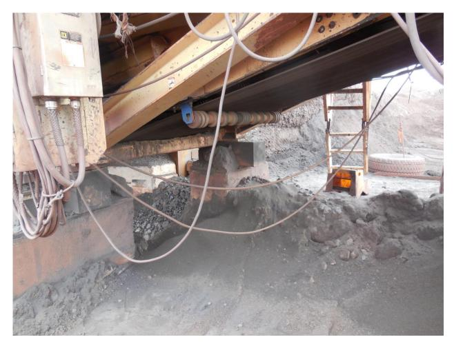
The CEC Rule 2-112 requires the mechanical arrangement and execution of the work in connection with any electrical installation to be acceptable. Properly support the cables such that they are protected from physical damage during clean up operations.
