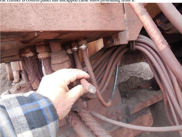
7. The crusher B control panel has uncapped cable stubs protruding from it.
