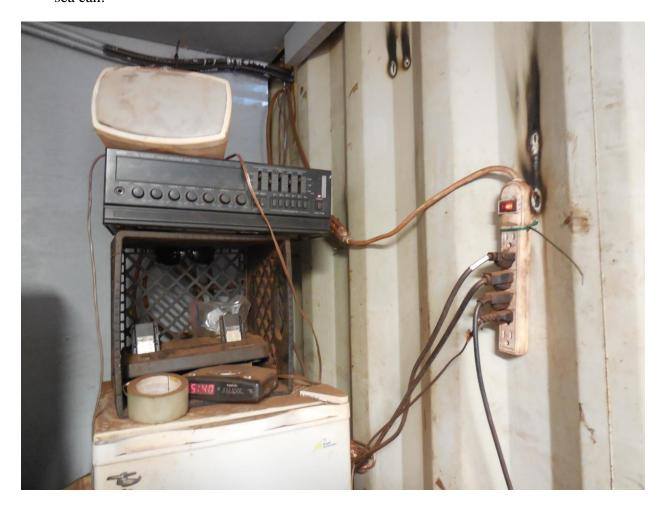
The Canadian Electrical Code Item 4-012 (3) (a) states that, "Flexible cord and cord sets shall not be used as a substitute for the fixed wiring of structures and shall not be (i) permanently secured to any structural member; (ii) run through holes in walls, ceilings, or floors: or (iii) run through doorways, windows, or similar openings." The CEC Subrule 2-300 (4) requires defective equipment to be put in good order or permanently disconnected.
