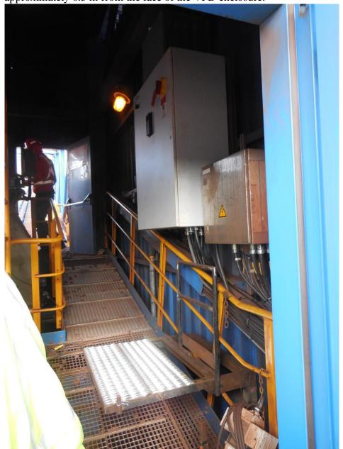
CEC Subrule 2-308 (1) requires a minimum working space of 1 m with secure footing about this type of electrical equipment. Modify the design of the platform to provide 1 m working space. A suggestion was made to add a removable railing on the downhill side as the platform doesn't extend much past the edge of the enclosure and an electrician attempting to use the left hand rule for switching would be well over to that side.
