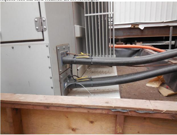
4. Ensure that the pad mount transformer and containment is installed in accordance with a certified design and that clearances are in accordance with the CEC Sub-Rule 26-242 (2) which states, Dielectric liquid filled pad-mounted distribution transformers shall be installed at least 3m from any combustible surface or material on a building and at least 6m from any window, door, or ventilation inlet or outlet on a building,
