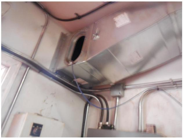
The CEC Rule 2-112 requires the mechanical arrangement and execution of the work in connection with any electrical installation to be acceptable. Also, CEC 60-314 states that communication conductors shall not be placed in ducts or plenum chambers except as permitted by Rules 2-130 and 12-010.
